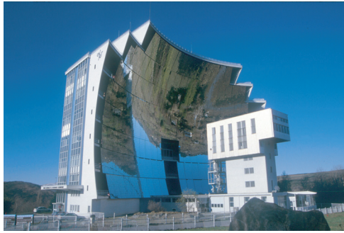
FIGURE 95 The last mirror of the solar furnace at Odeillo, in the French Pyrenees (© Gerhard Weinrebe).
