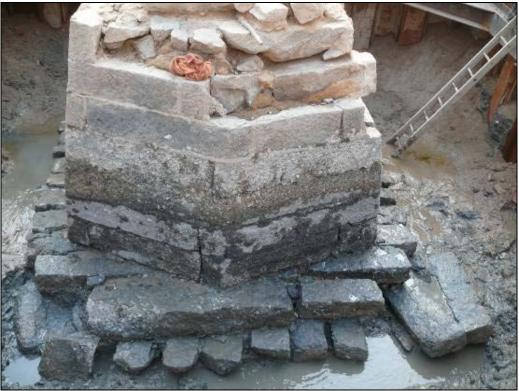
Figure 8 Supporting pillar SP6 and its footings
