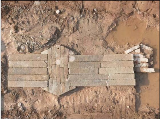
Figure 6 Supporting pillar and granite decking (From right to left: SP1, GD1, SP2, GD2)
