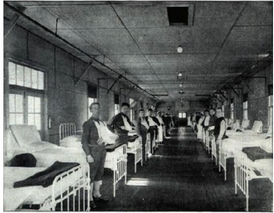
FIG. 26.—Interior of typical one-story ward of temporary construction.
