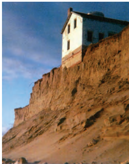
The Smith Island Lighthouse as appeared in 1970 after its lantern room was removed. The structure is now standing precariously close to the edge of the 60-foot high cliff. ( Lighthouse Digest archives.)
