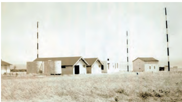
Various support buildings at Smith Island Lighthouse in 1940. At the far left and barely in the photograph is the paint house, then two water tanks, the garage, a shop, radio building, and engine room. (Photo courtesy Judy Bearman.)
