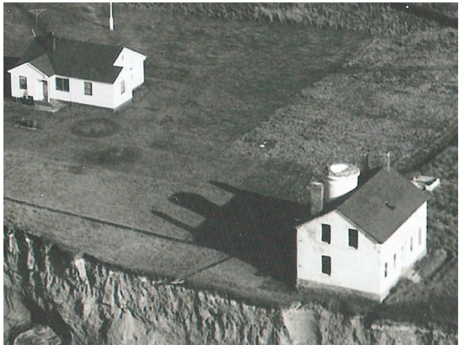
The Smith Island Lighthouse as appeared in 1970 after its lantern room was removed. The structure is now standing precariously close to the edge of the 60-foot high cliff. ( Lighthouse Digest archives.)
