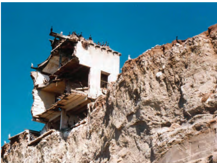
This series of three photographs, taken in 1989, show what remains of Smith Island Lighthouse, ready to collapse over the edge of the cliff marking the end of a once important lighthouse station on the Pacific Coast of the United States of America. Shortly after these photos were taken the last remnants of Smith Island Lighthouse went went down over the side. (Courtesy of David and Georgene Finch.)
