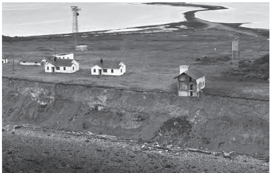
As can be seen in this 1983 photo, a section of the Smith Island Lighthouse has broken away and debris can be seen on the beach below. Also, the bluff has moved dramatically closer to the keepers' homes and other structures. ( Lighthouse Digest archives.)
