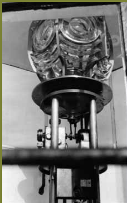
The Fresnel lens was still in the tower at Smith Island Lighthouse when this photo was taken in 1948. Photograph by Don Skiff.
