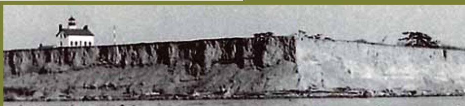
Smith Island Lighthouse in 1949 as it appeared from the water. It was less than 50 feet from the edge of the bluff by this time.
