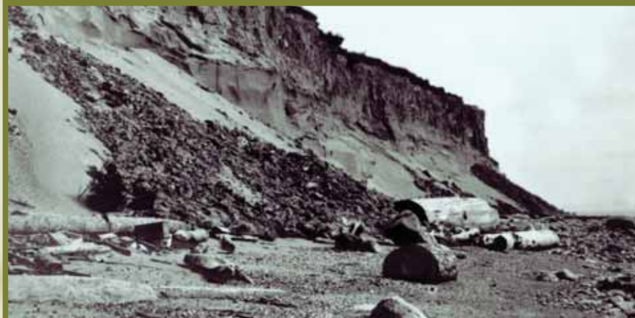
This image shows how serious the erosion problem was at Smith Island with pieces of the lighthouse structure seen scattered about.
