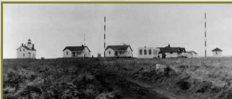
Smith Island Lighthouse Station as it appeared in 1949. The block building in the center was the watch shack, containing radio gear, generators and batteries. The tall poles were the radio beacon antennas used for navigation. All electric on the island at that time was D.C. from a bank of 18 large lead-acid truck batteries connected in series and recharged by gasoline powered generators. It was still a family station in those days. At that time there were three families, plus one single keeper who boarded with one of the families. Only one child was living on the island at that time. Don's wife, Pat, was pregnant at that time. The 83-foot cutter stationed at Port Townsend had to make an emergency run to take Pat to the hospital and the boats crew said they made the trip to Port Townsend in record time. By the 1950's families were no longer permitted to live on the island. Don said this was a good idea since the station was too isolated for most women and he recalled that he saw a lot of tears out there. Photograph by Don Skiff.
