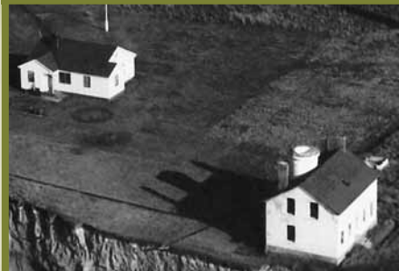
In 1964, lighthouse historian, Jim Gibbs wanted to save the lighthouse. However, by that time it was too close to the edge of the cliff to move in the necessary heavy equipment to safely move the structure. So, with the government's permission, he was at least able to save the lantern room by removing it. This aerial view shows the lighthouse without its lantern room only a few feet from the edge.
