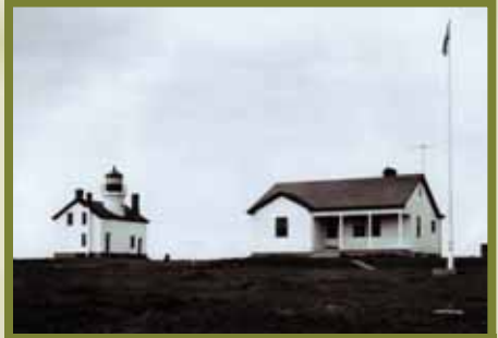
As erosion crept closer to the lighthouse, the structure was deemed unsafe and the keepers moved into more modern housing as shown at the right.
