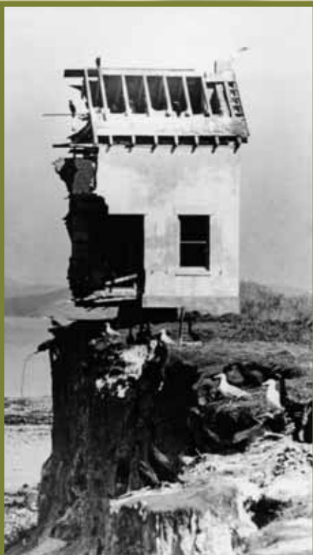
What is left of the Smith Island Lighthouse teeters on the brick of the bluff in the 1980's. Shortly after this photo was taken, the last remaining section of the structure finally toppled over the edge. Photograph courtesy Coast Guard Museum Northwest.
