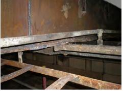
Frame 77, web and lower flange buckled (buckled longitudinal deep frame already removed)
