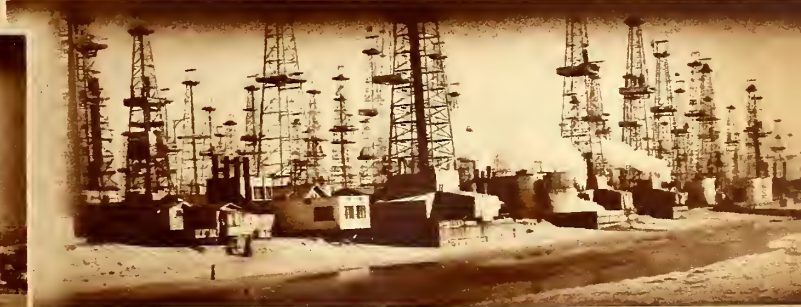
OIL PRODUCTION forms one of the basic industries of Southern California, Los Angeles County having several thousand wells in production. Here is a scene at the seashore in the Venice oil field.
