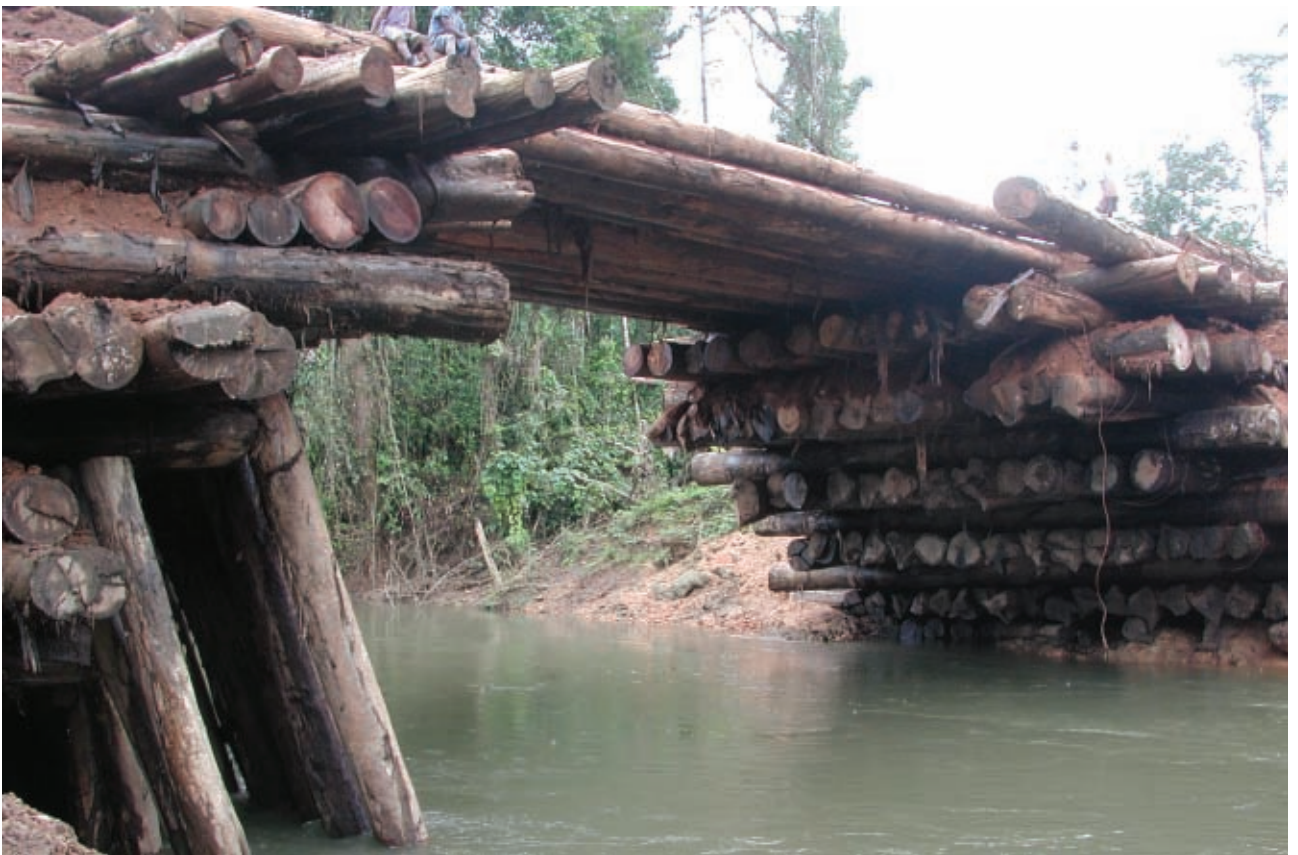
Plate 7: Large numbers of trees are used in the building of temporary bridges. Here approximately 250 trees are in the construction of this bridge in central Wawoi Guavi, Western Province. In this concession, several bridges of this size are constructed within each kilometre of roading.
