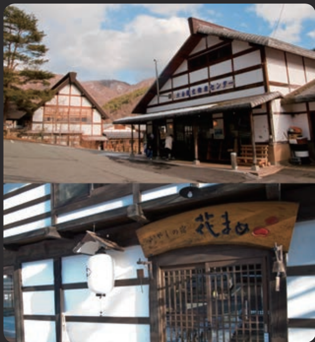
Road Side Station KUNI
