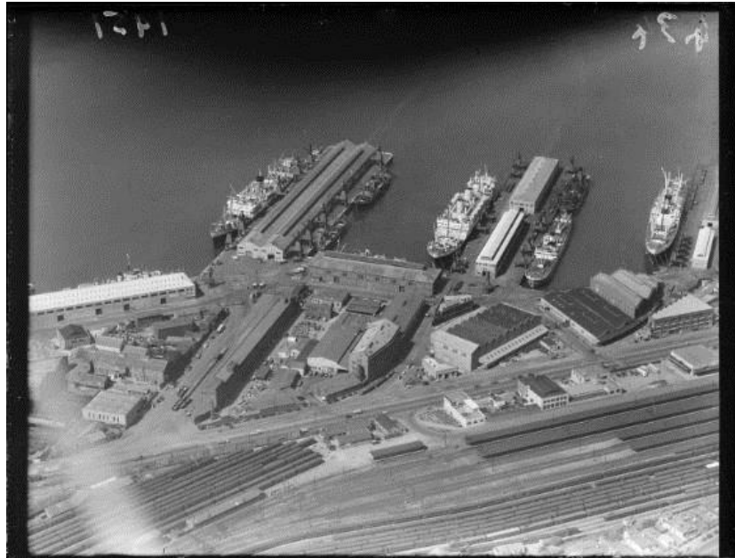
Figure 4: Aerial view of Wellington Harbour and the wharves, ca 6 April 1951. ATL, ID: 114/277/07-G. Shed 35 is between Pipitea Wharf (left) and Kings Wharf (right). The wedge shaped building at the end of Kings Wharf is Kings Wharf Office (Former). Permission of the Alexander Turnbull Library, Wellington, New Zealand, must be obtained before any re-use of this image.
