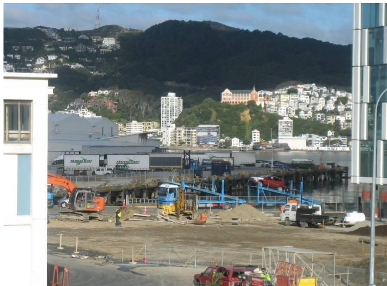
Figure 8: King's Wharf from Waterloo Quay overbridge
