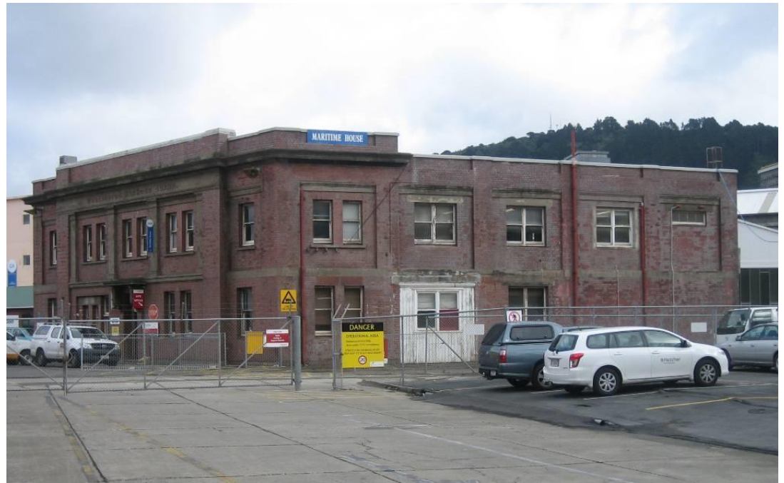
Figure 6: Kings Wharf Office (Former)
