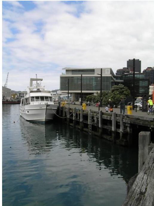
Figure 24: Ferry Wharf No.2 (Former), December 2011. (K. Astwood, NZHPT)
