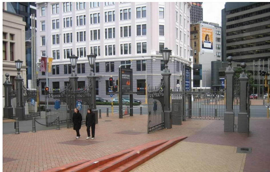
Figure 17: Queens Wharf entrance gates
