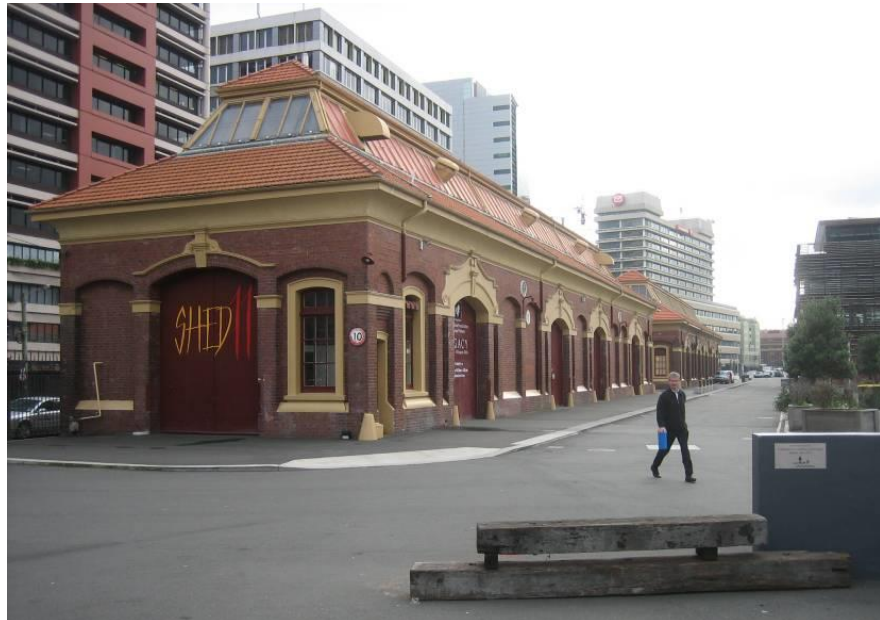
Figure 26: Shed 11 in foreground with Shed 13 behind
