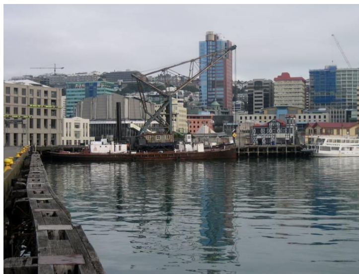
Figure 46: Looking west towards Taranaki Street Wharf with fendering system on the left and Hikitia at the berth
