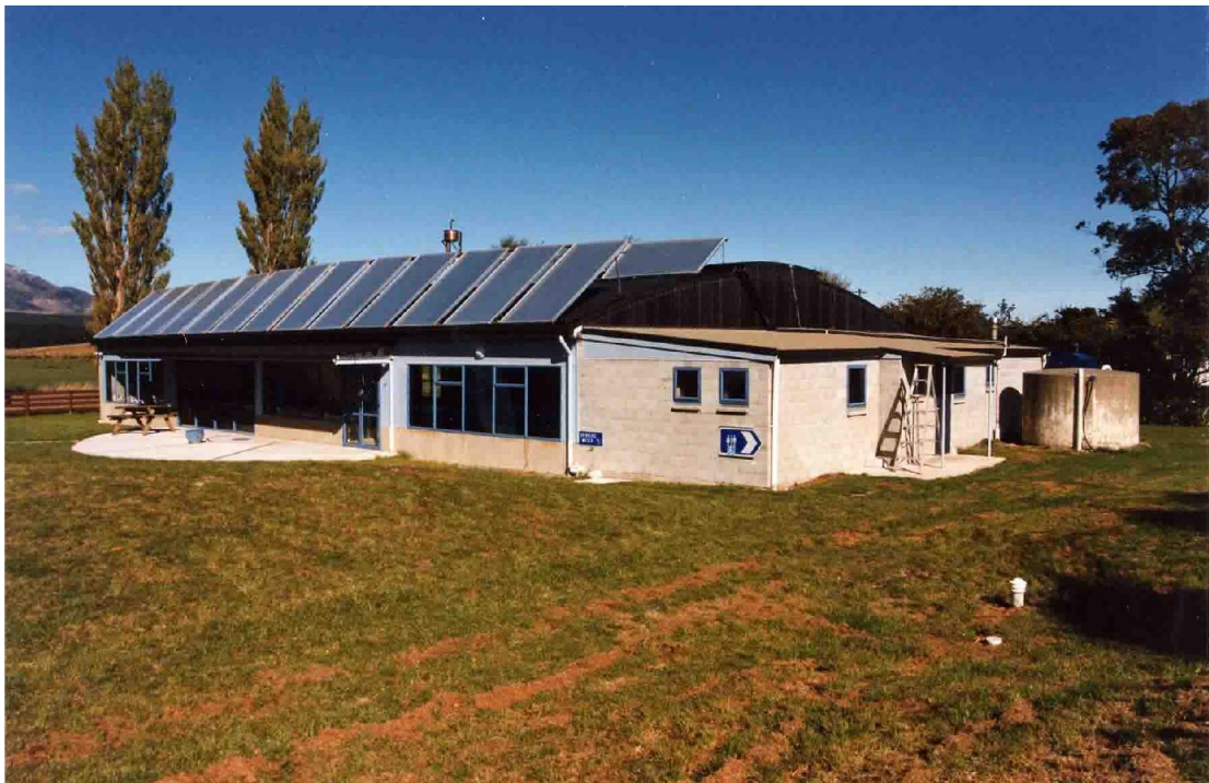
Figure 2, Swimming pool with solar panels installed.
