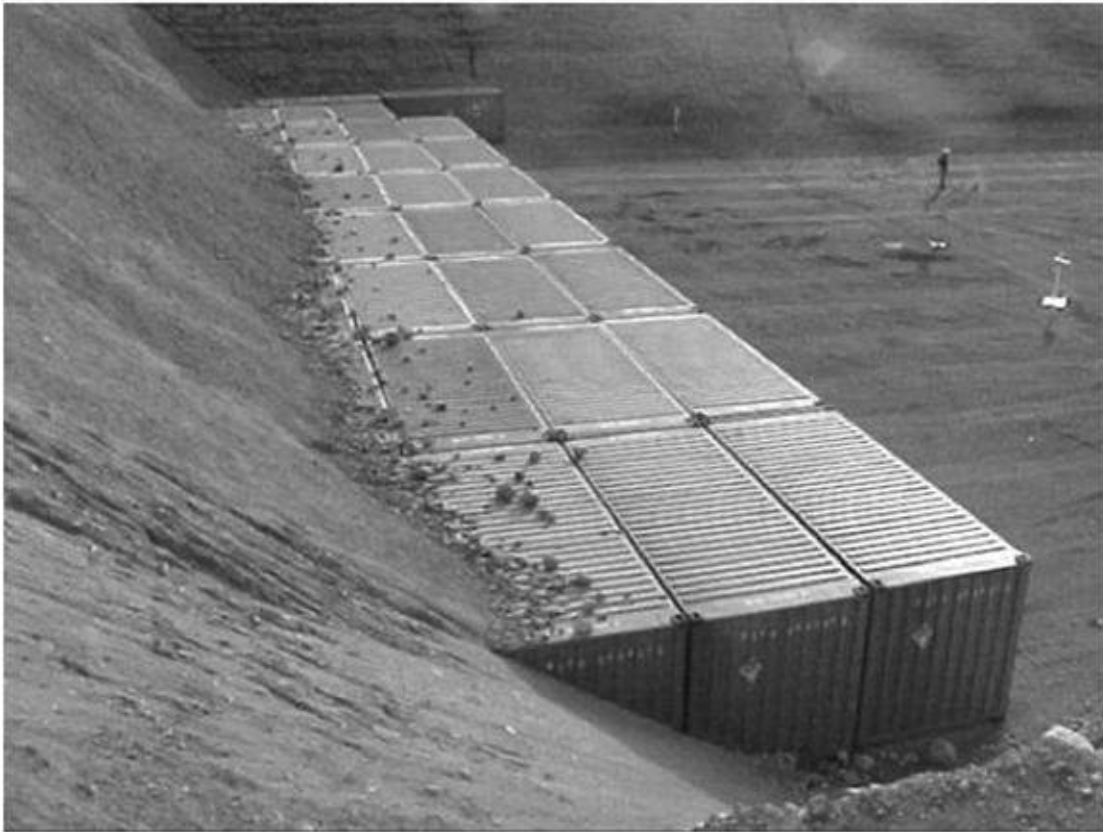
Figure 9b. Due to lack of current demand, the U.S. government has returned about 3,200 metric tons of refined thorium nitrate to the crust, burying it in the Nevada desert. Image courtesy of the National Nuclear Security Administration Nevada Site Office.
