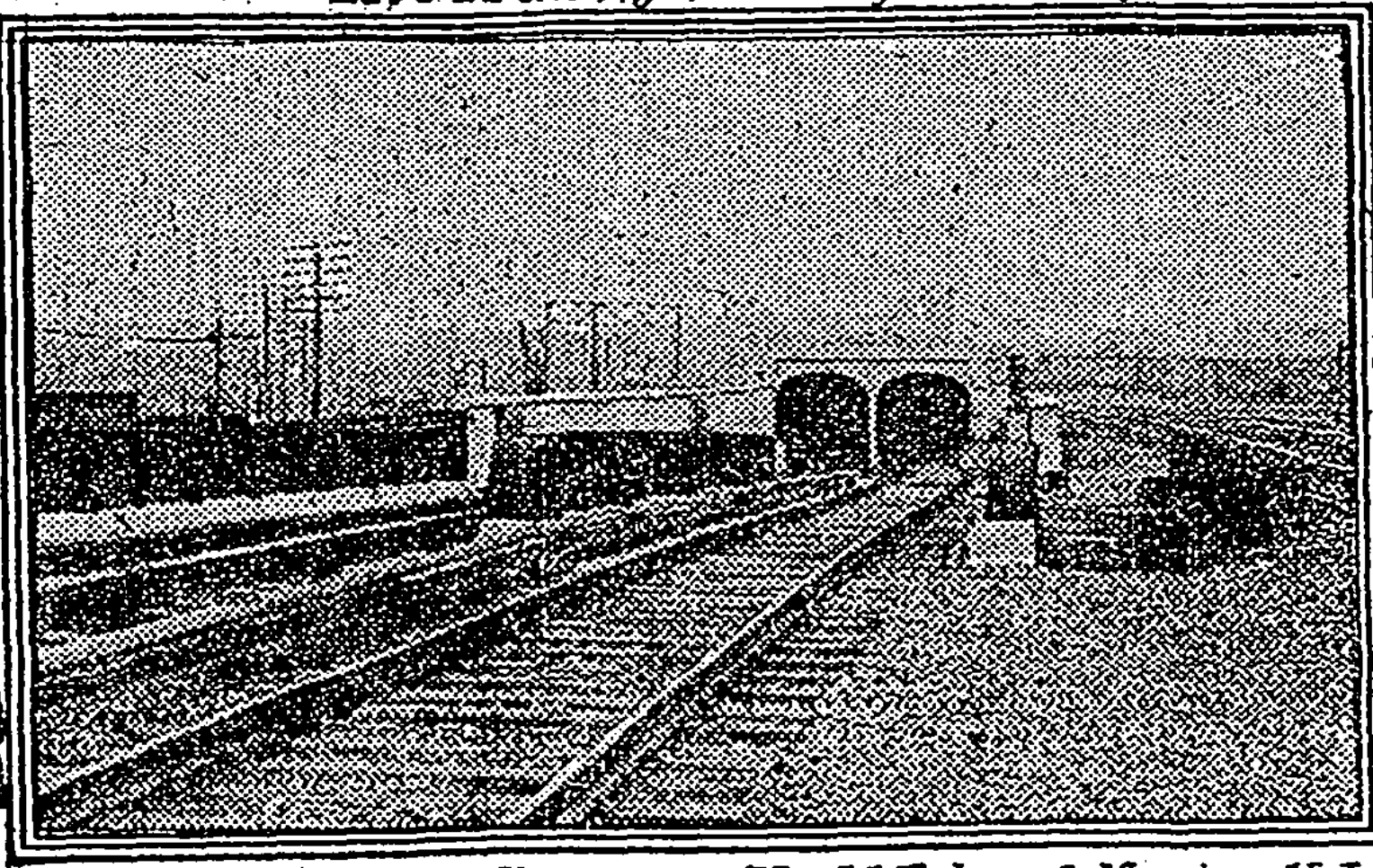
Portals of the Extended H&M Tubes at Marion N.J.
