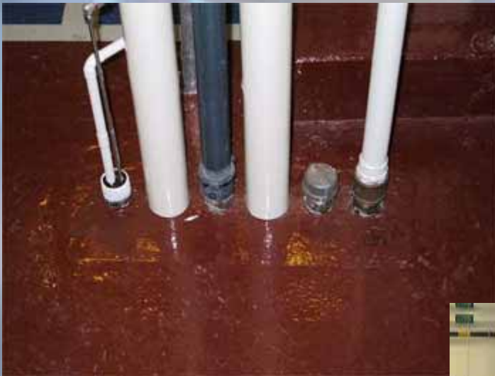
Sealed pipe penetrations
