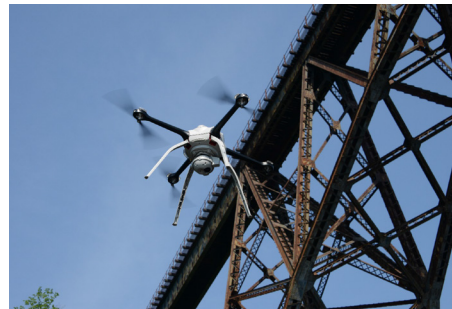
Drone Bridge Inspection
