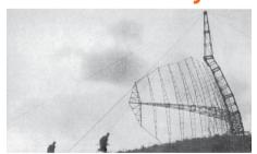
The 5N84A Oborona-14 is a very high frequency band (30–300 MHz) early-warning radar meant for installation in a transportable, trailer-mounted configuration. The NATO reporting name 'Tall King'.
