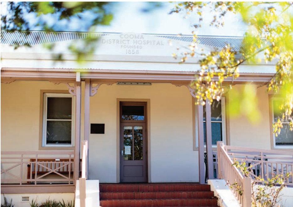
← Part of the original 1867 Cooma Hospital building
