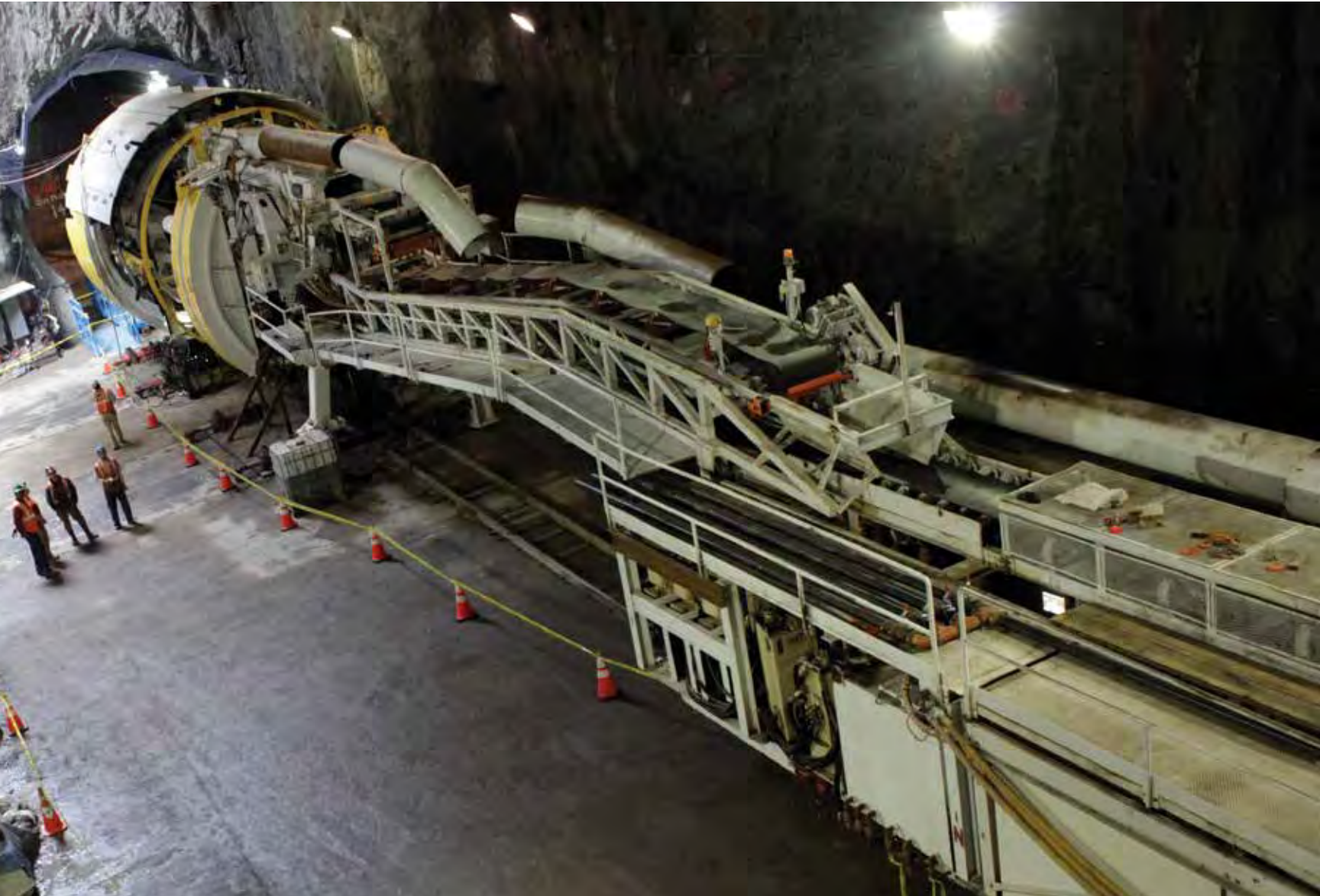
Digging into Manhattan's bedrock for the new Second Avenue Subway, on which Peter Chamley served as chief engineer.
