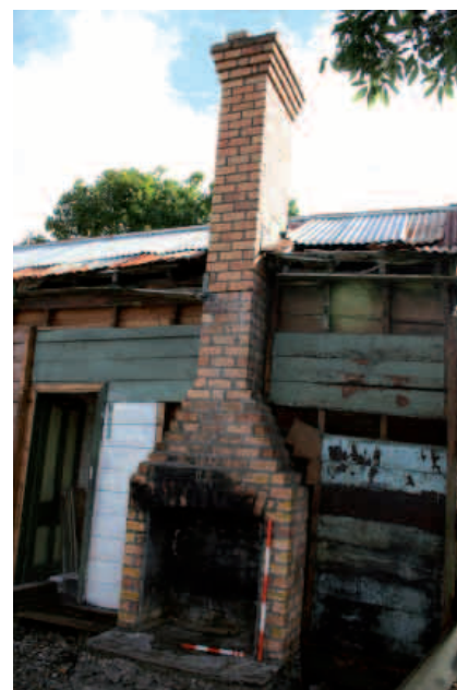
29 (above). The chimney and fireplace within room G4, following deconstruction of the lean-to.
