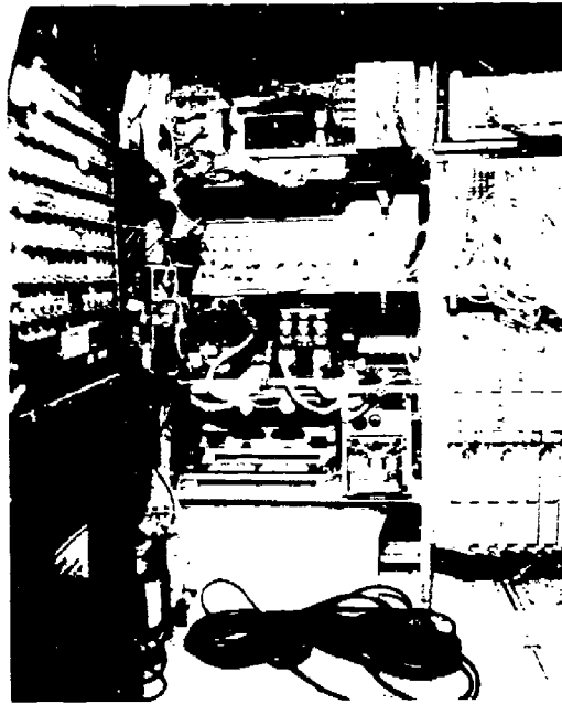
Figure 42. Cabin Instrumentation Rack - Forward Section.
