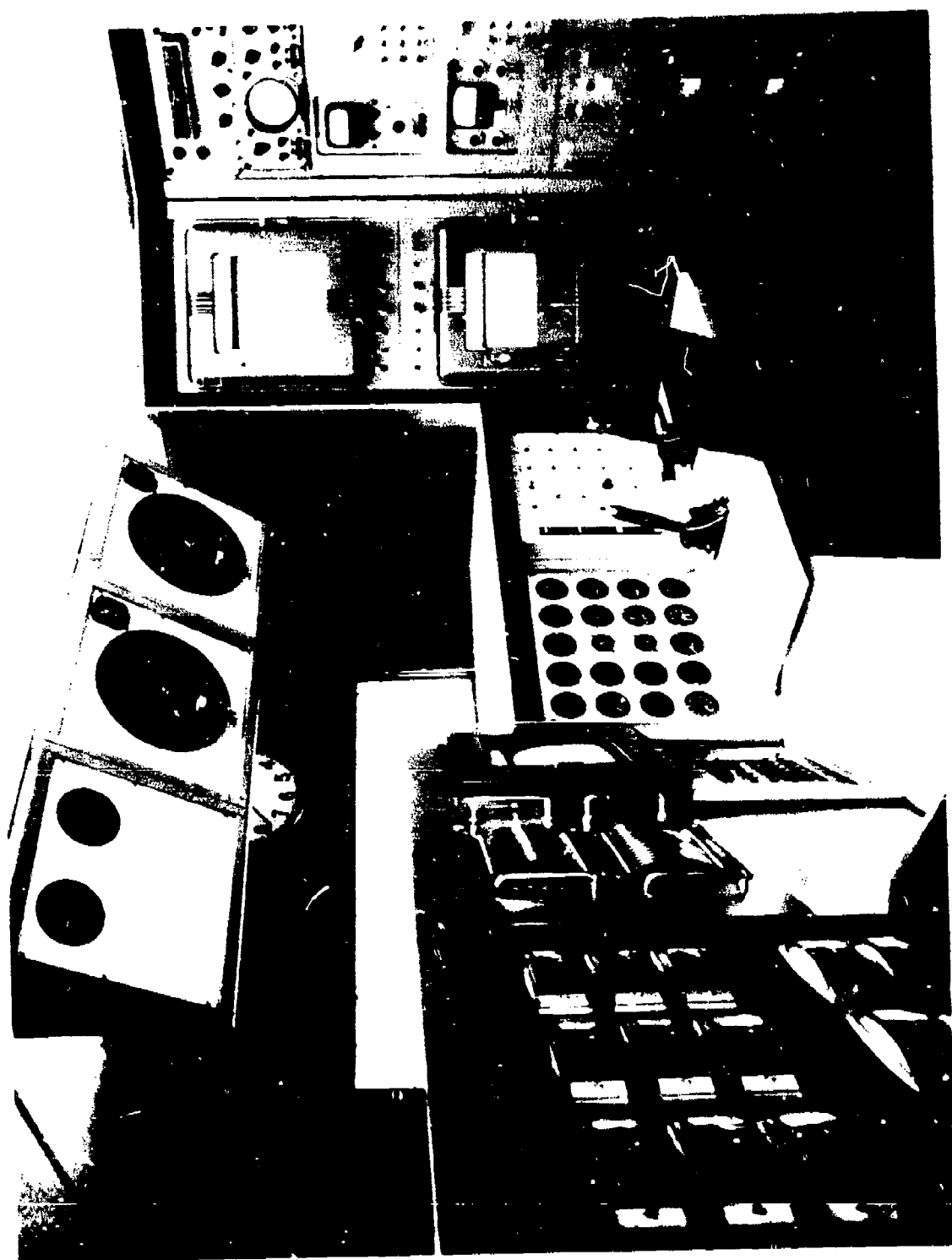
Figure 40. Propulsion System Test Bed Control Room.
