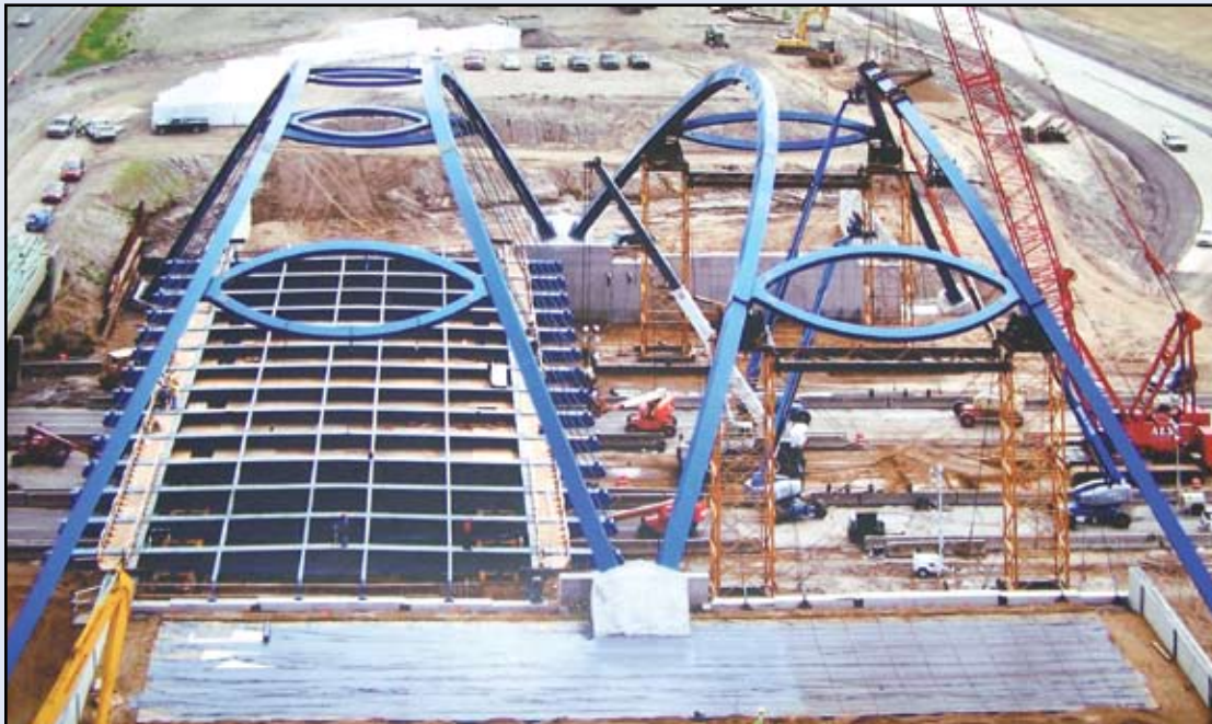
Figure 8: Arch mid-section being lifted into place
