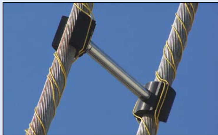
Figure 6: Spacer to minimize hanger vibrations
