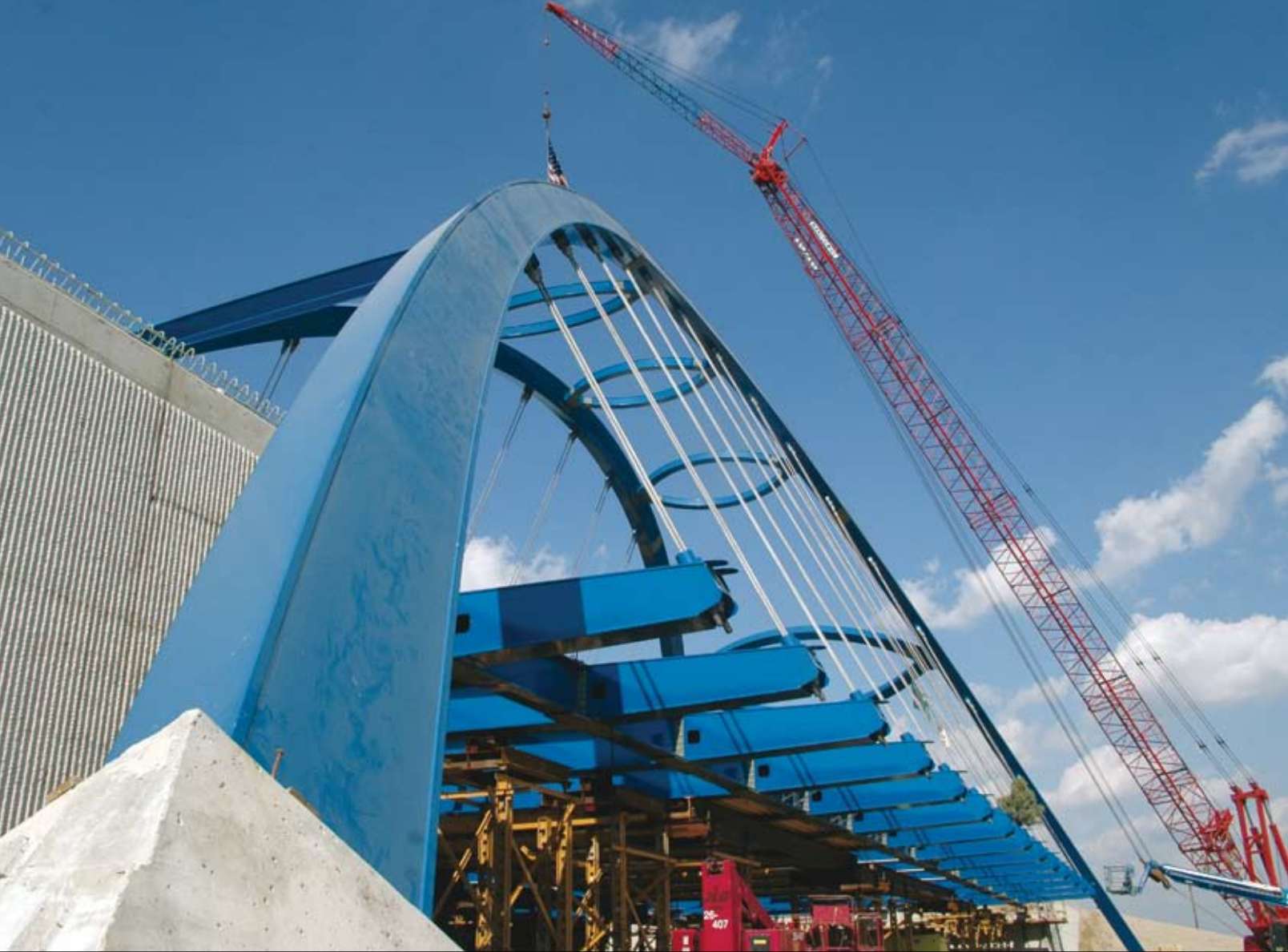
Figure 5: Transverse I-beams with box shaped end
