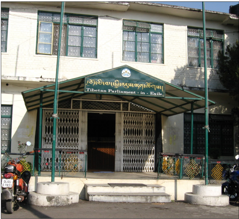
Image 2.1 Below, the Tibetan Parliament-in-Exile building, in Dharamsala, India houses the semiannual parliamentary gatherings. (Photo by author)
