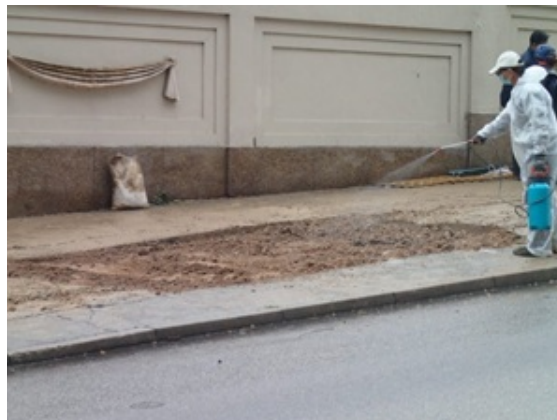
Photo 15 The planter was backfilled with new soil
