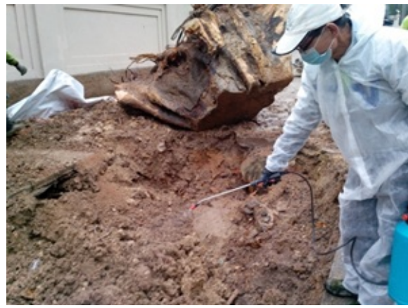
Photo 14 Application of disinfectant on the soil inside tree pit
