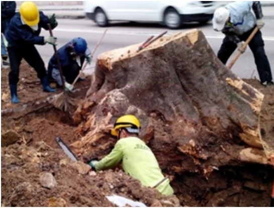
Photo 11 Stump removal in progress
