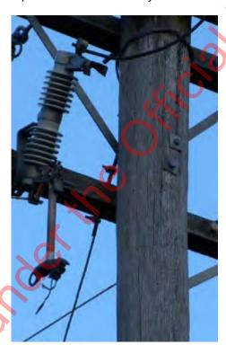
Fuse tube (orange) lodged in fuse carrier and Earth Clamp
