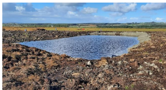
Figure 42. EIP-funded pond intended for aerial fire-fighting near Athea, Co. Limerick. (Image: DAFM)
