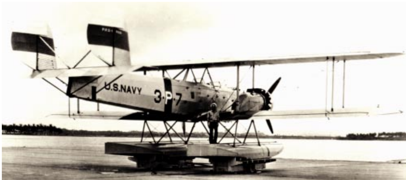
A squadron P2D-1 on the launching ramp.
