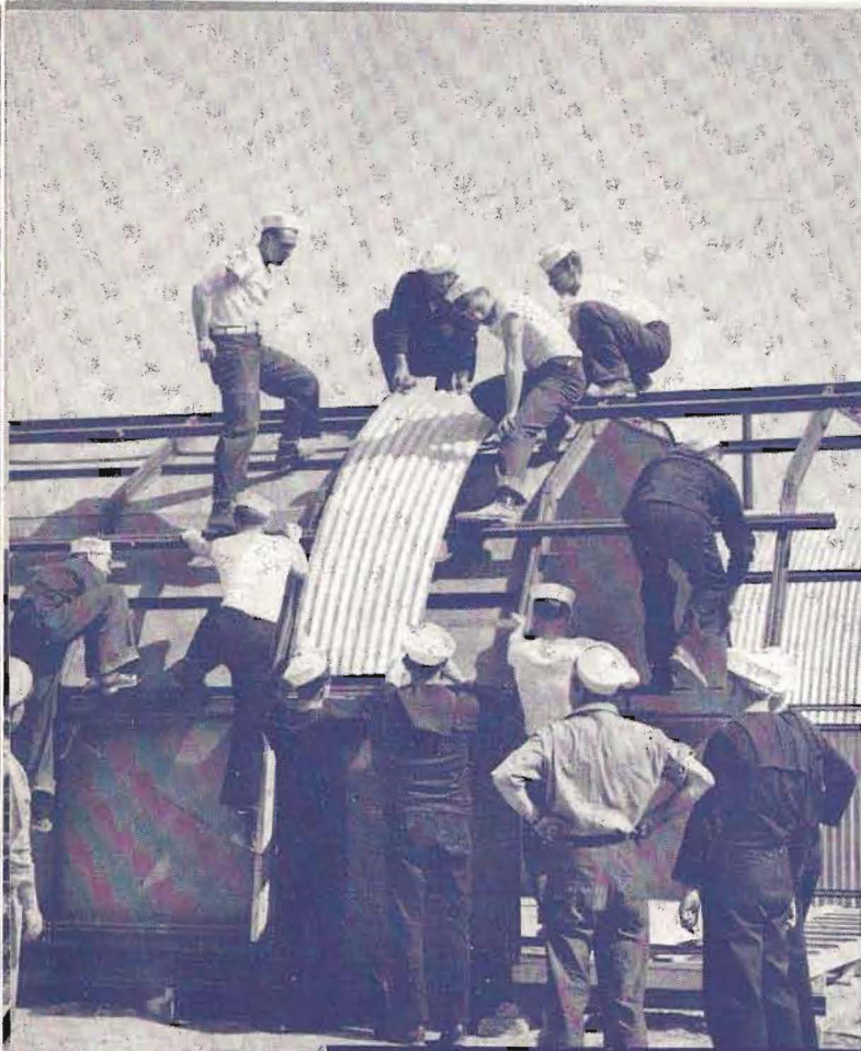
At a Virginia training center, Seabees learn how to build the famous Quonset huts in which they will live overseas.
