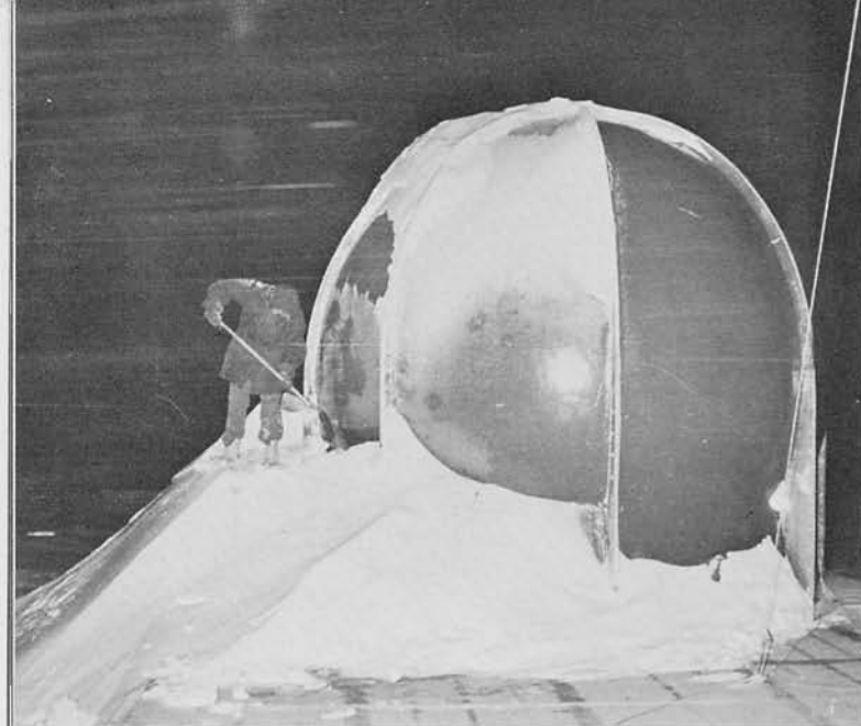
WEATHER data radioed back from "bugged" balloons high in sky are picked up by parabolic antenna inside rawin dome. Plastic dome is kept free of snow to allow reception of radio signals. Below, John and Noble work on meteorological data before releasing it to IGY Weather Central.
