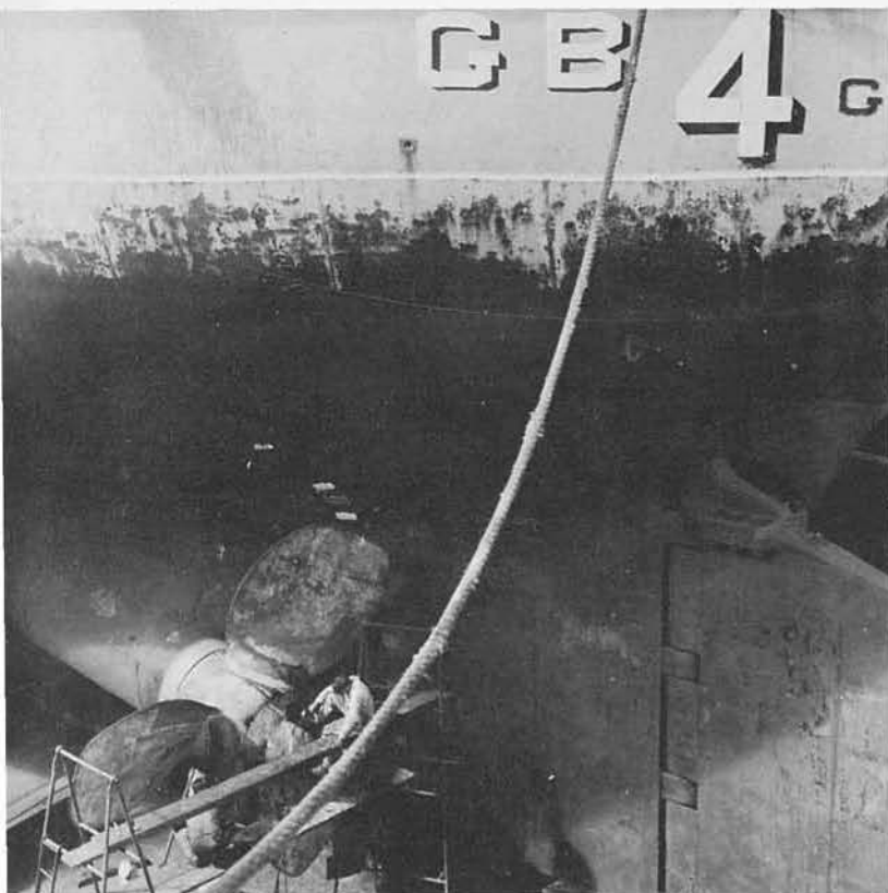
◀ PUTTING FINISHING TOUCH ON NEW BLADES.
