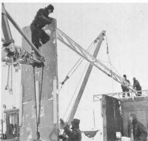
and P.W. Officer LTJG Robert K. White work on tractor boom (center) used to raise roof trusses of new garage (right), a valuable facility built of scrap material.
