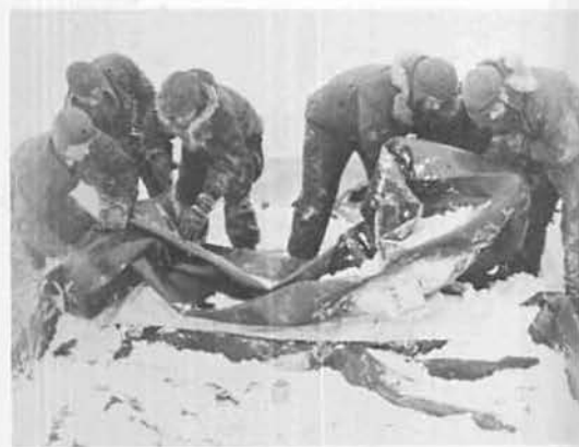
Byrd Land. Fuel caches consisted of 3,000-gallon rubber tanks (right, being serviced) buried in the snow and marked by trail flags for easy spotting in featureless icecap.
