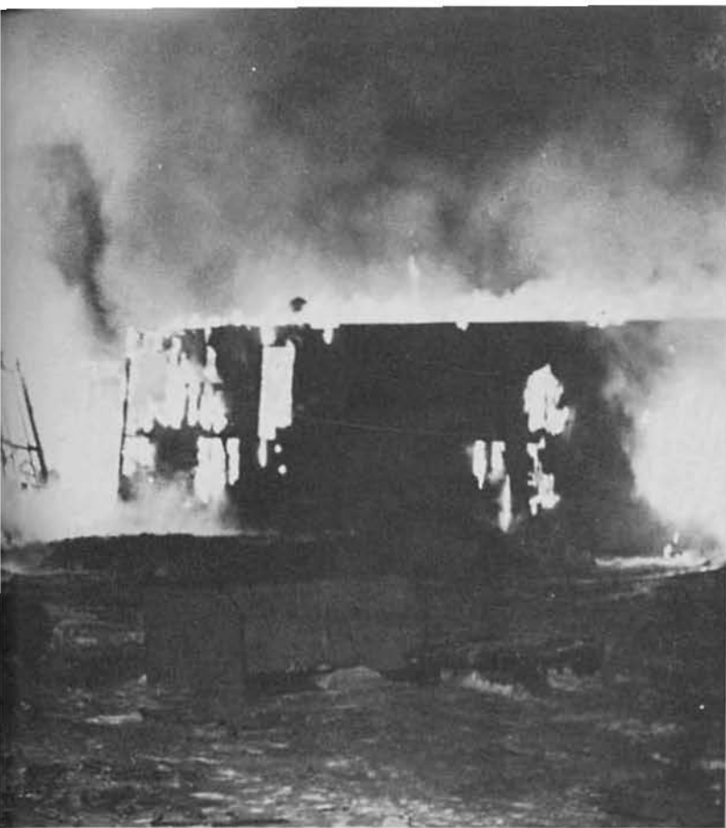
NAF GARAGE, REPAIR SHOPS A COMPLETE LOSS.
