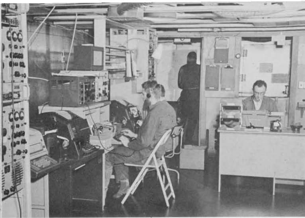
CORNER OF BUSY COMMUNICATIONS BUILDING AT LAS.
