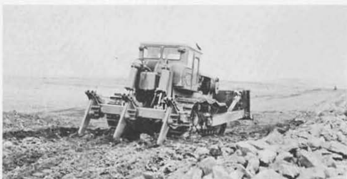
AFTER permafrost dam was breached by dynamite to form channel (opposite page) temporary runway for supply purposes was completed. The D-9 Caterpillar tractor (left) heaviest made in the U.S., ripped and graded the rocky
