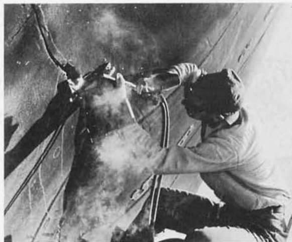
BURNING OUT CRACK FOR REPAIR PATCH.
