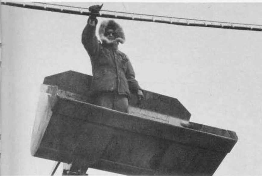
SECURING POWERLINES TO WITHSTAND HIGH WINDS.
