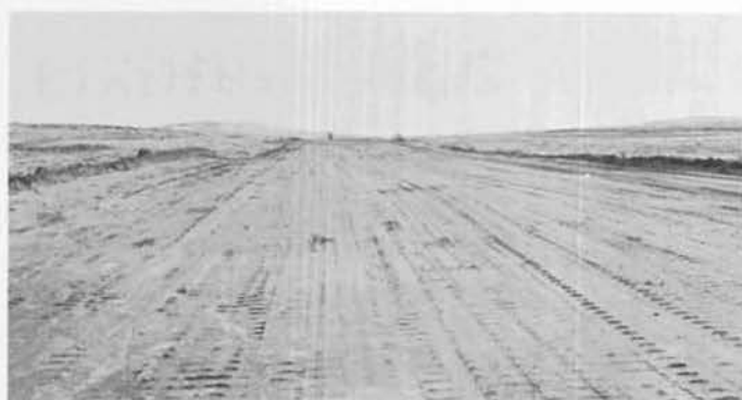
terrain to smooth strip. Runway appears in upper left photo on opposite page, running diagonally from bottom of picture toward meltwater creek. (Mountains in that photo are foothills of Royal Society Range in Victoria Land.)
