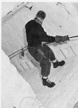
DEEP PIT at Byrd reached 60 feet (left, center). Glaciologists descended by rope, came out by ladder. Ellsworth pit (right), dial thermometers in wall.
