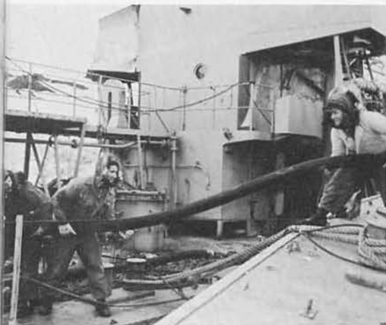
NESPELEN offloads avgas. Oiler is moored to ice by deadmen (far top). Fuel line is passed from ship to shore where it is hitched to 250,000-gallon storage tanks (at LAS and
