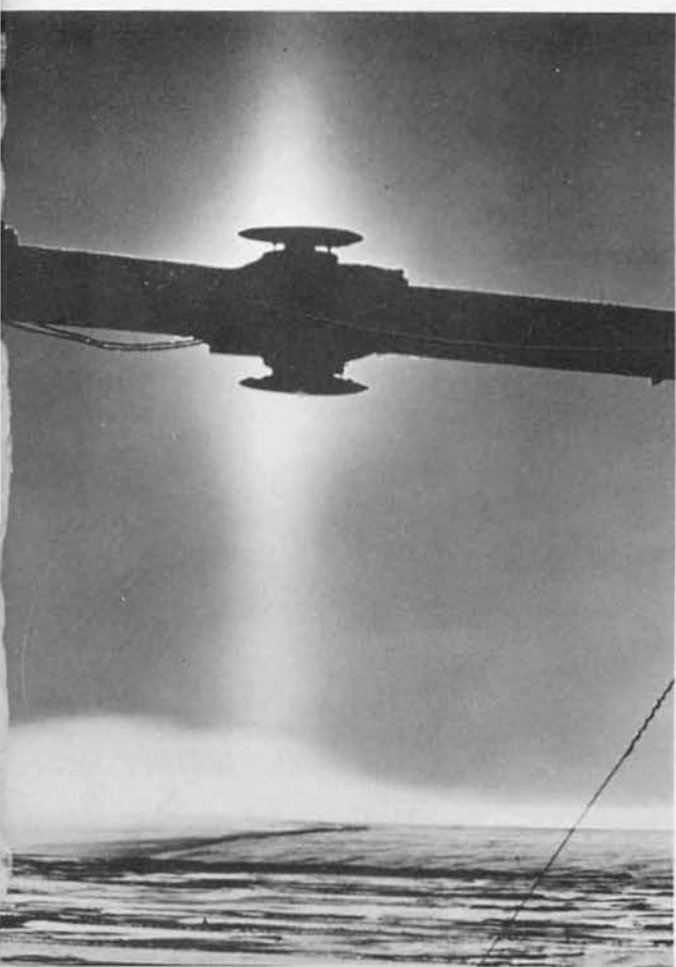
USNC-IGY SUNSET and Taps and the lowering of the flag. With the sun goes light and warmth. Pyrheliometer at LAS (above), measuring incoming and reflected thermal radiation, is silhouetted against the darkening sky and "sun pillar."
