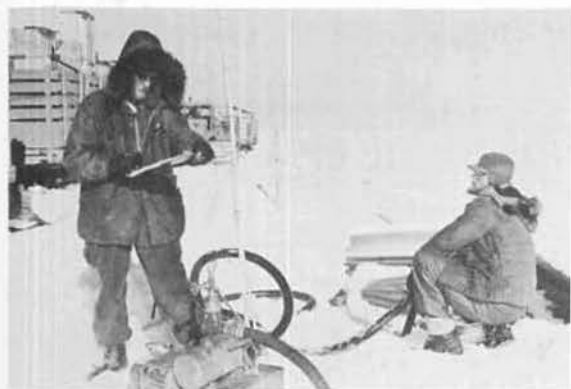
tank. Automatic portable pump (right) is used at Mile 120 to fuel tractors. Liv Base was similarly equipped with buried tanks for emergency Pole-bound plane landings.
