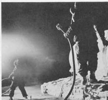
TRANSFER of diesel fuel for station use was a tedious job. Left, fuel is pumped from 55-gallon drums into sled tanks on barrier for transfer to station storage tanks.
