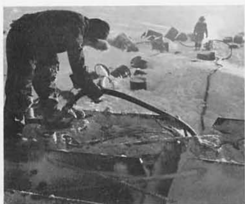
TRANSFER of diesel fuel for station use was a tedious job. Left, fuel is pumped from 55-gallon drums into sled tanks on barrier for transfer to station storage tanks.
