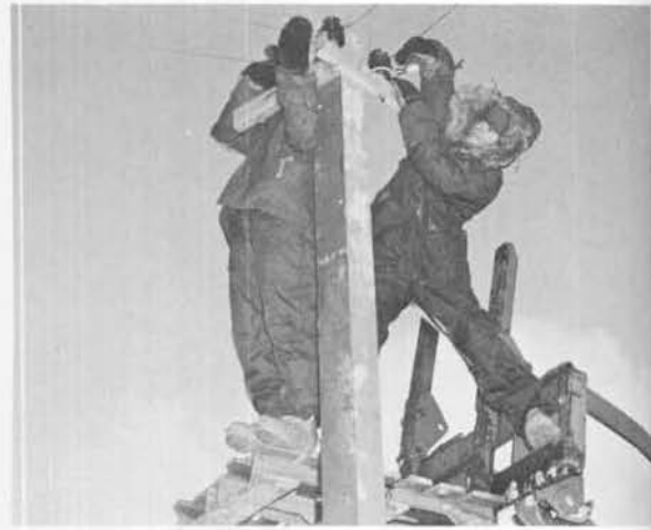
STRINGING ANTENNA WIRE IN ICY AIR.
