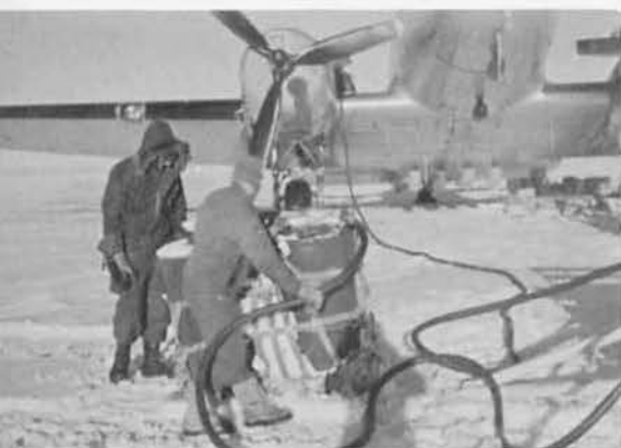
BYRD TRAIL posed major logistics problem. Navy R4Ds with huge interior tanks (center, being filled) were flown from LAS or Byrd Station to caches along tractor trail in
