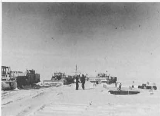
TRACTOR train halts at Mile 380 where VX-6 laid fuel cache; train took on 5,400 gallons at this call. Note trail flags marking tanks, valved standpipe emerging from
