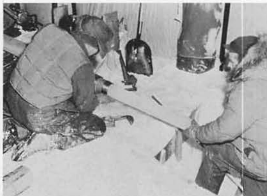
ICE CORE DRAWN FROM CORE BARREL.
