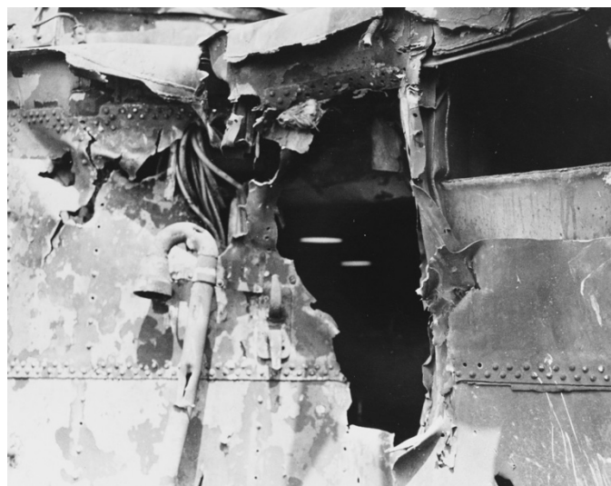
This view of Laffey shows severe exterior damage to the wardroom bulkhead on her starboard side (NH 75423).
