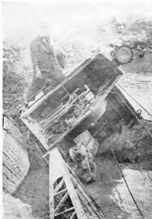
Crane overturned in Bay
