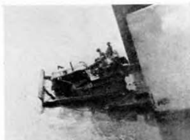
As a bulldozer rolls down the ramp
