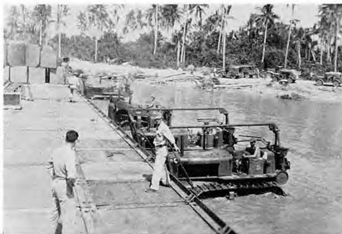
Seabee-devised pontoon docks and causeways have played major parts in most invasions. Here the 105th shows how
