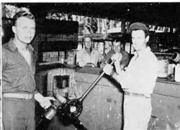
The pipe shop
