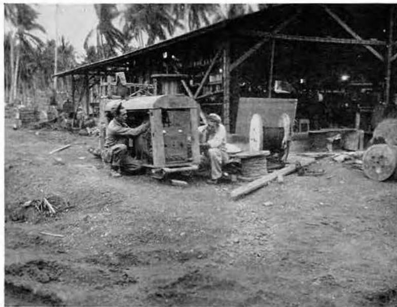
Generator repair in the yard
