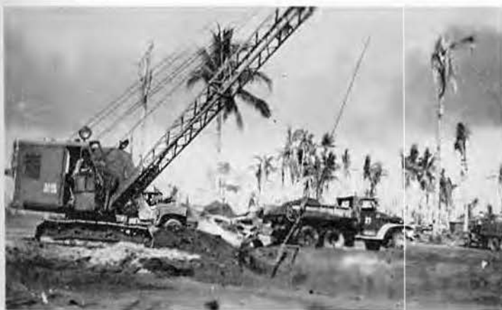
Draglines, too, scoop fill out of the sea
