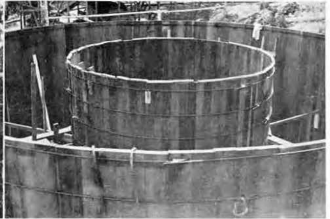
Three stages in the construction of a filtration plant designed to serve all Navy shore activities in the area. Also a closeup showing concentric construction of the wooden tanks, and covering the top
