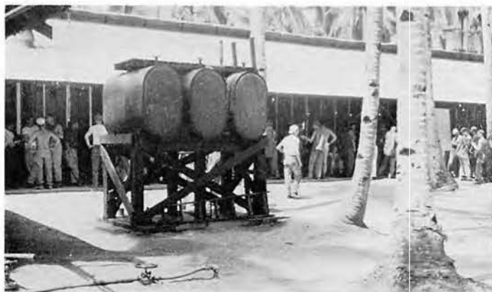
Fuel tanks serving the galley ranges
