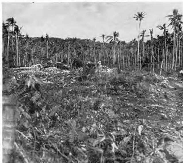
Areas like this are cleared for air strips
