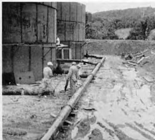
Welding pipe connecting the tanks
