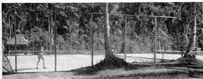
Concrete tennis courts built for the fleet
