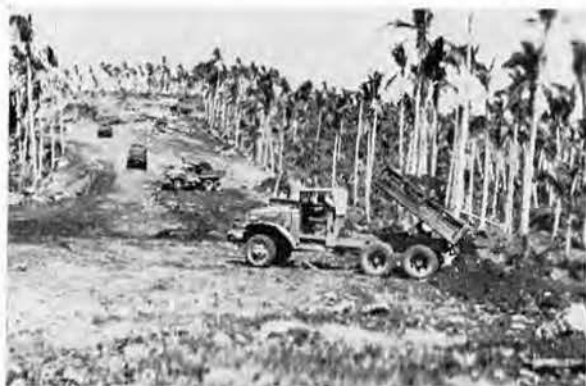
Trucks supplying fill on road project
