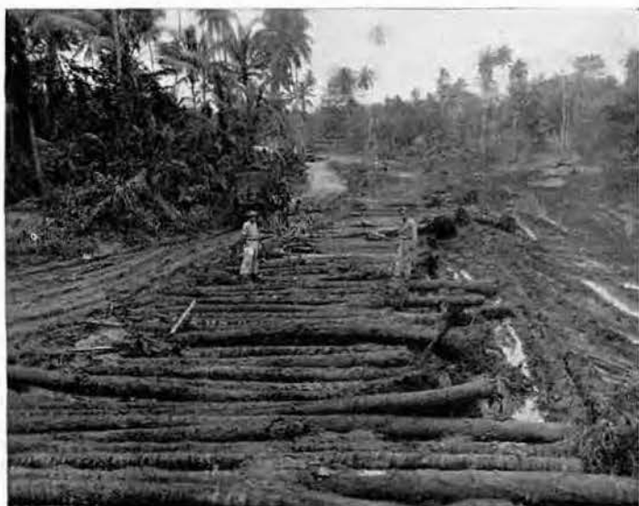
But sometimes the going is too boggy, and a log bed is used as a base for fill
