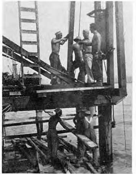
Pile driving, as speed and more speed is called for
