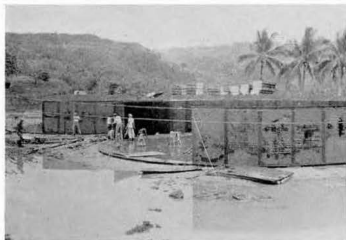
Wednesday . . . the tanks begin to take shape
