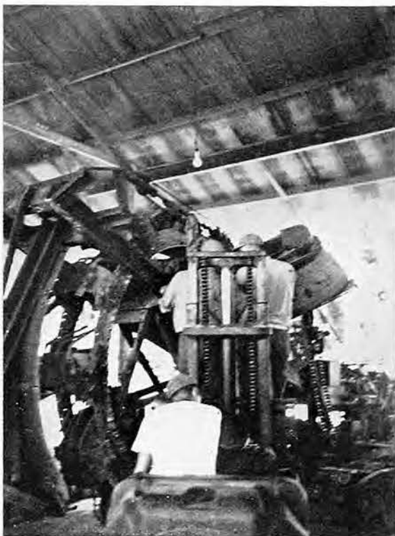
Ditcher undergoing repairs
