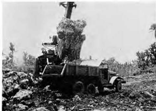
A dump truck is loaded with fill under a hot sun
