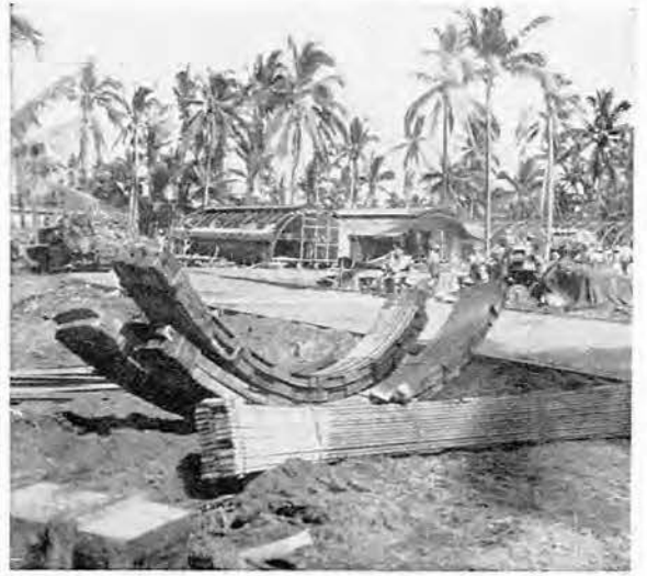
Quonset ribs in packages, just as they are shipped
