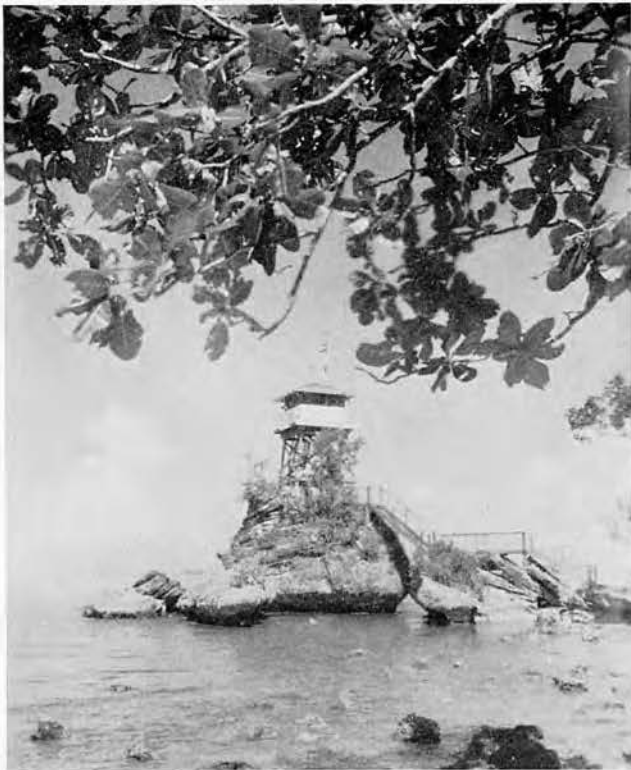
Signal tower built for ship-shore communications
