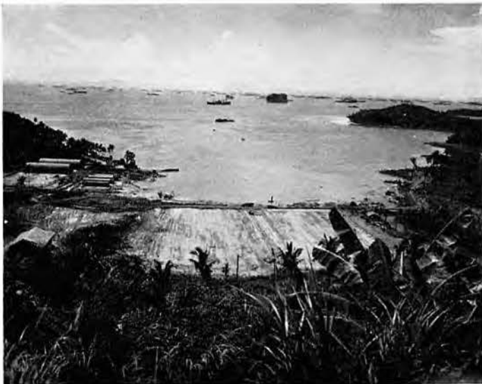
NSD, project of Heavy Equipment and Construction under the direction of Engineering
