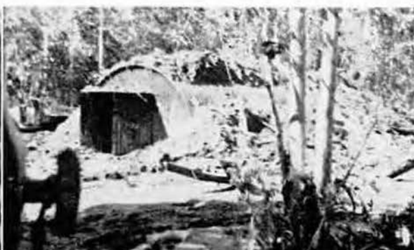
Ammunition storage hut, Nissen type
