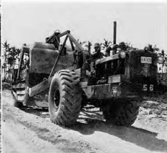
A turnapull working on a taxi way for an air strip in New Guinea
