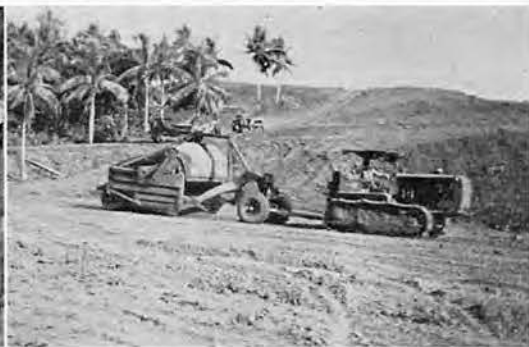
A pan grading fill as a road nears completion
