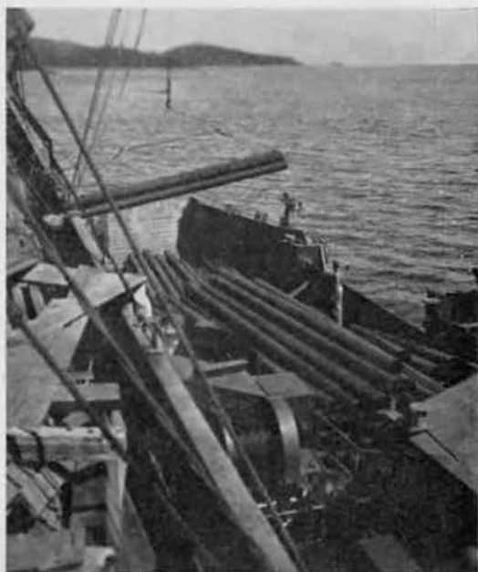
Loading barge with pipe for tank farm
