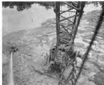
A high pressure hose washes the mud and silt from the coral
