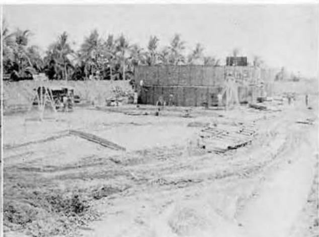
Friday . . . crews worked round the clock to get the tanks up
