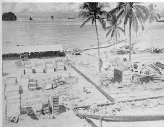
Completed fuel lines and pumping station
