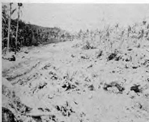
Before and after scenes of another road job in the Philippines
