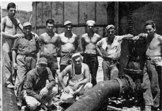
Oleszkiewicz' pipefitting crew
