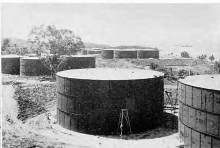
View of a portion of the completed tank farm
