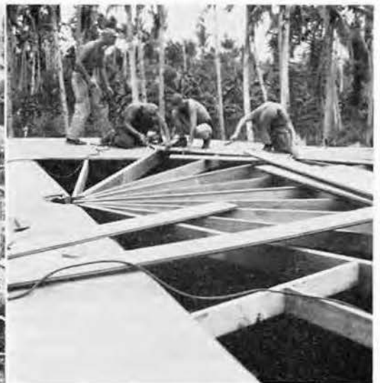
Three stages in the construction of a filtration plant designed to serve all Navy shore activities in the area. Also a closeup showing concentric construction of the wooden tanks, and covering the top
