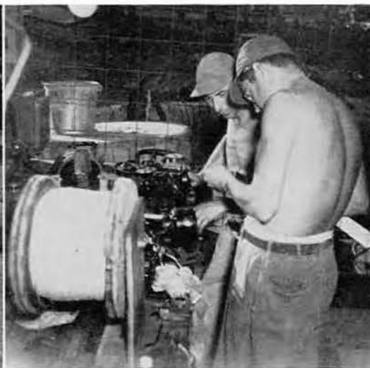
Rewinding motor in shop
