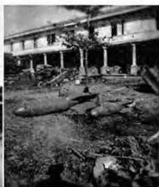
The warehouse near the dock area
