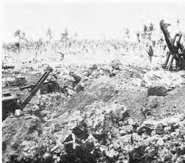
Shovels scoop out fill for the roads from coral pits, such as this one
