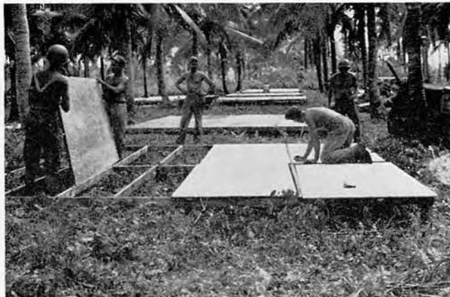
Laying floor for tents to house personnel
