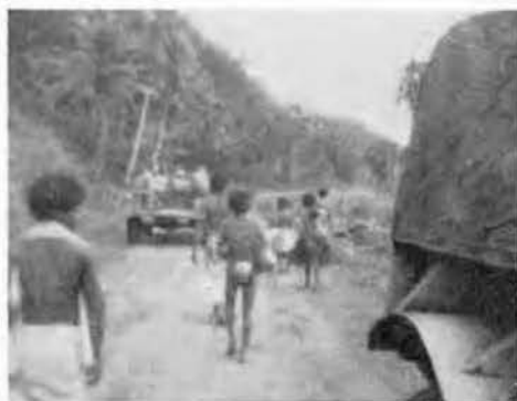
Natives on a road at Hilimoi
