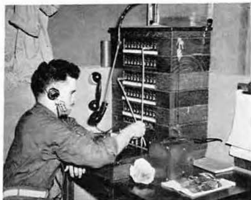
The switchboard for intercamp communication
