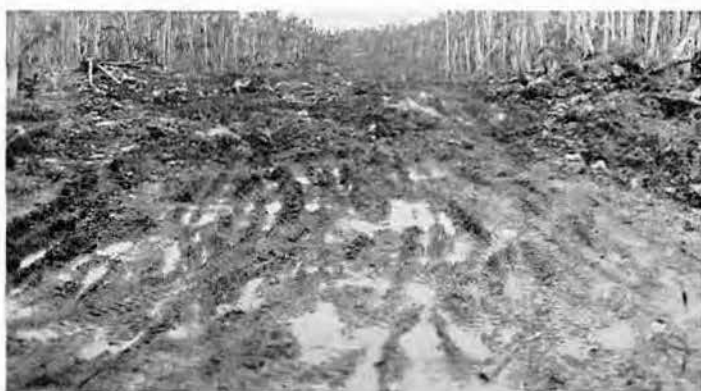
But sometimes the going is too boggy, and a log bed is used as a base for fill
