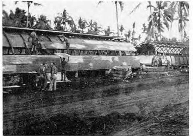
Applying roof to insulated hut in B.O.Q.
