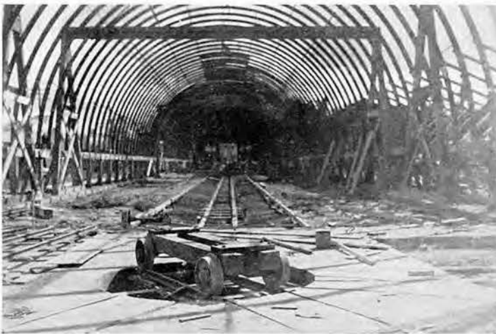
Uncompleted quonset viewed from the end
