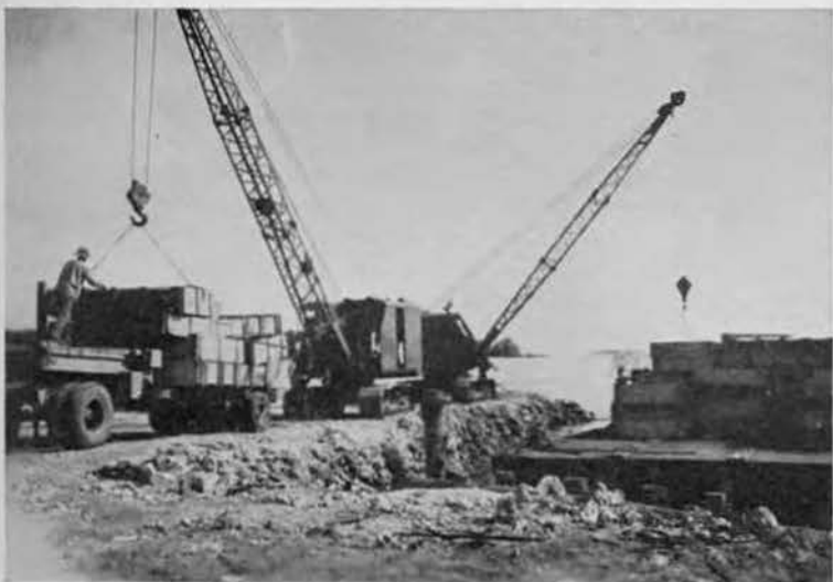
Quonset pieces being unloaded by cranes
