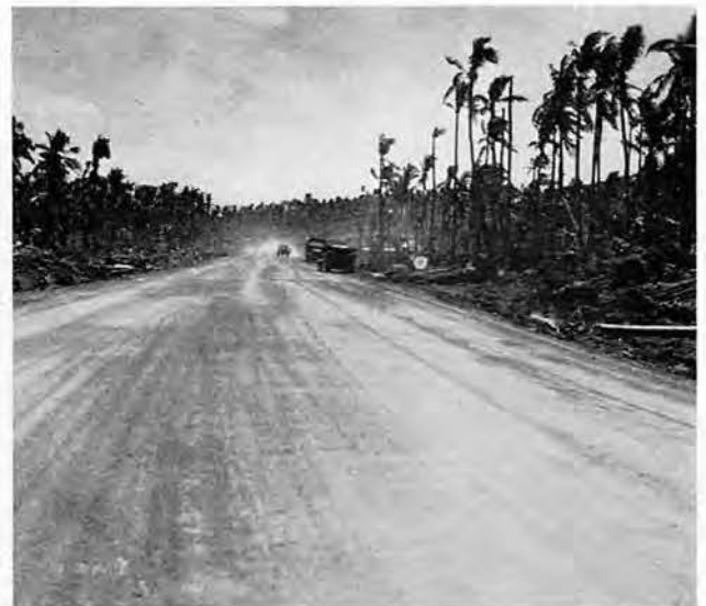
From the jungle emerges the completed road
