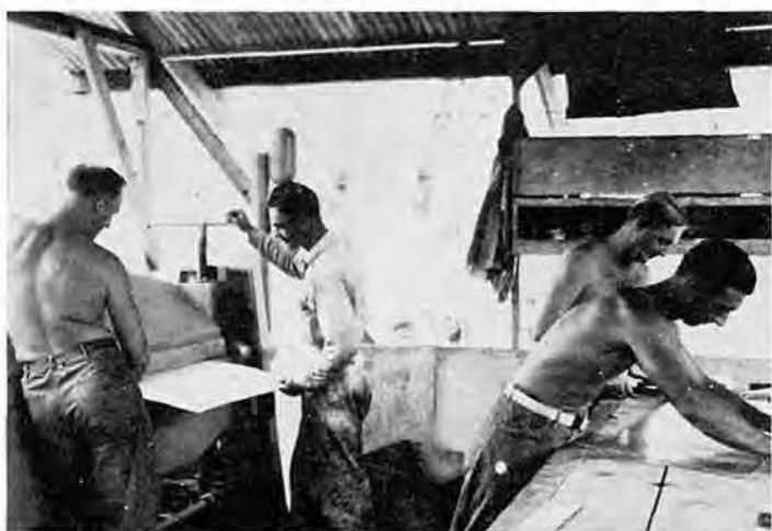
Sheet metal crew working with a captured Jap sheet metal brake
