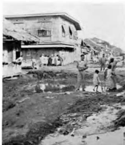
Pedestrian traffic detours around rain-filled bomb craters
