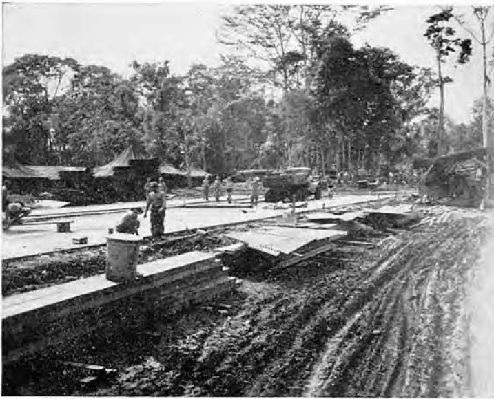
Cement pad on which quonset is to be erected
