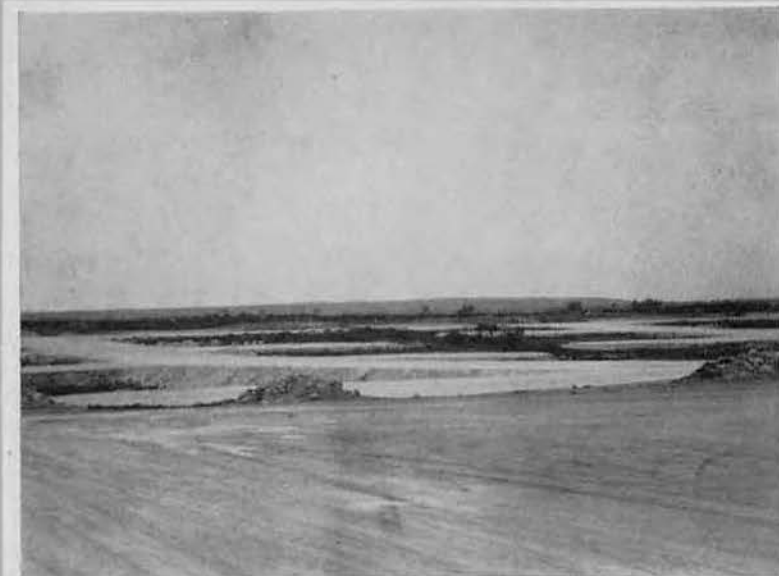
. . . with smooth, level hardstands.
