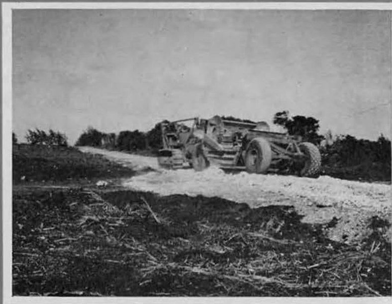
Right: A Carry-all, one of the big earth movers.
