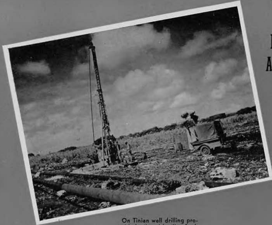
On Tinian well drilling provided the Island's fresh water supply.
