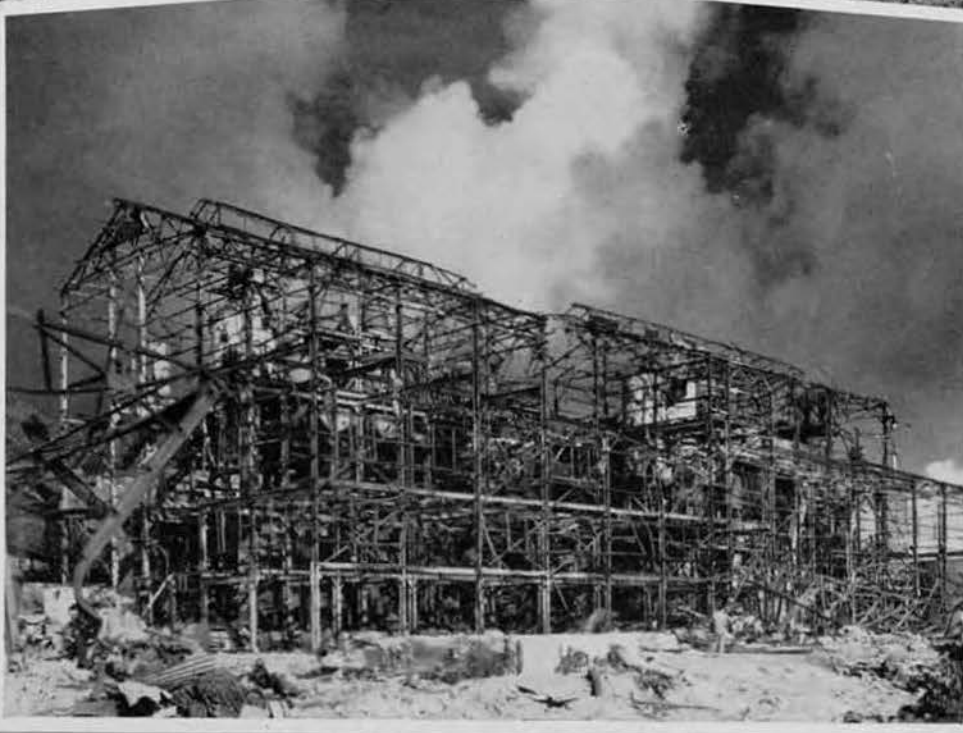
Twisted and tangled from fire and explosion, the Tinian Sugar Refinery was a tremendous salvage project for the iron workers.
