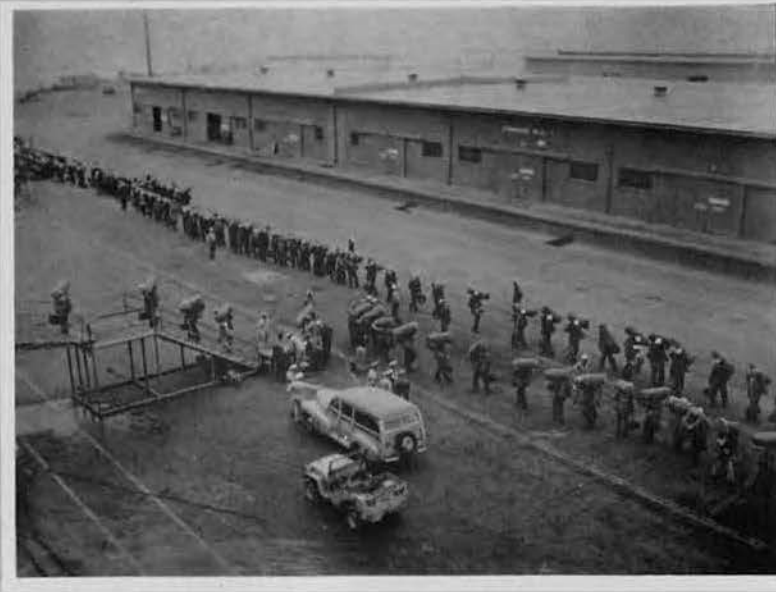
The gangplank was a difficult bridge to cross.
