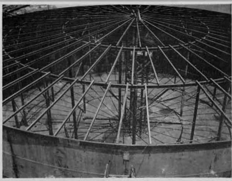
Interior of 50,000-bbl. storage tank.
