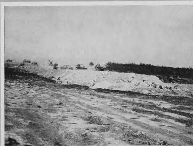
Every available piece of equipment was placed on airfield construction.
