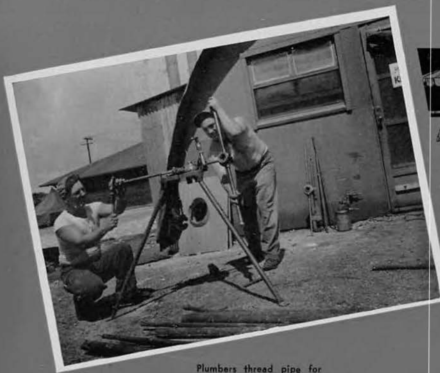
Plumbers thread pipe for interior steamfitting.
