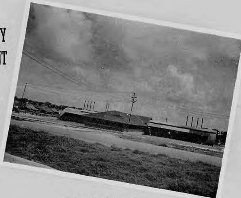
Exterior view of battalion galley and mess hall
