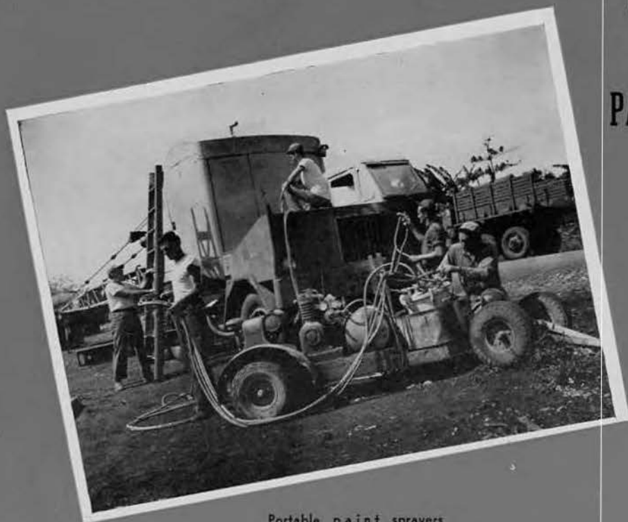
Portable paint sprayers "pretty up" heavy equip- ment in the field.
