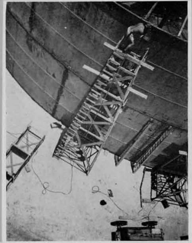
Right: Scaffold welding.
