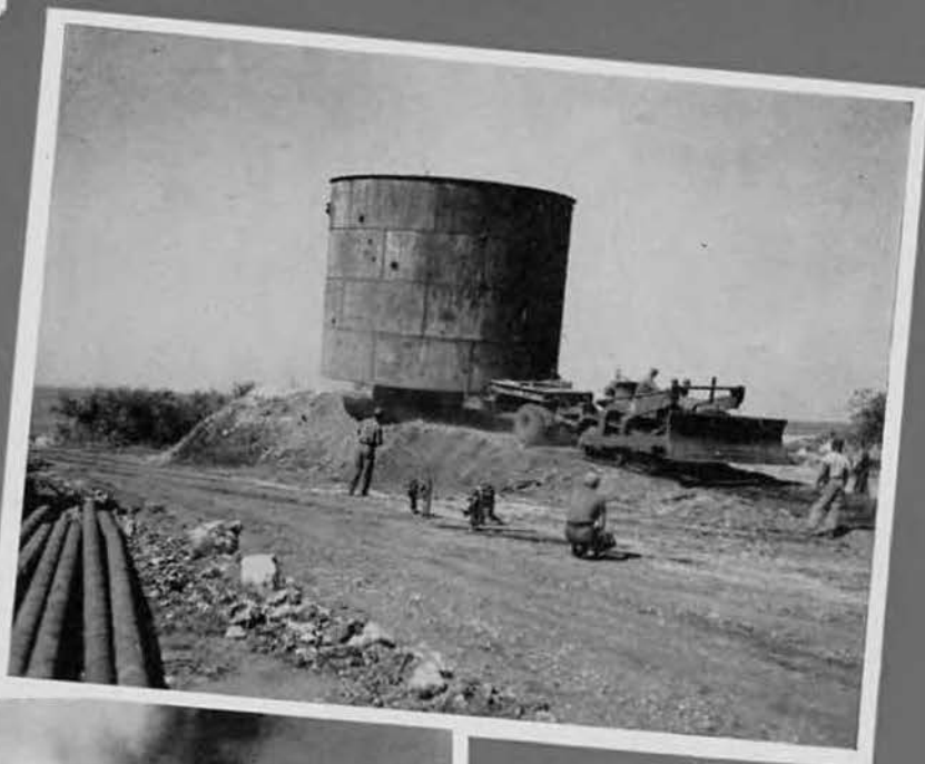
Enemy storage tank perforated from American shell burst was salvaged and repaired for salt water storage.
