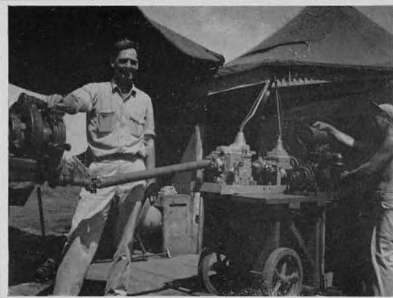
CWO Cross and his power pipe threader.
