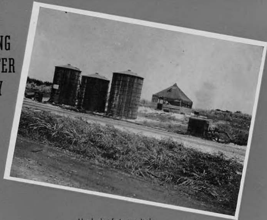
Hundreds of storage tanks and pipelines distributed water to all parts of Tinian.
