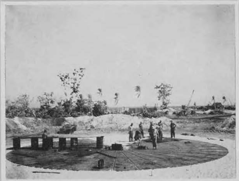
Right: for 10,000-bbl. steel tank decks.
