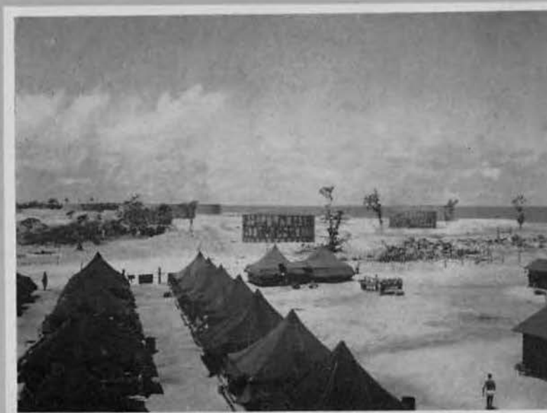
More sand and tanks.
