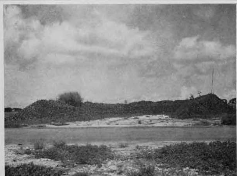
Old Jap revetments were replaced . . .
