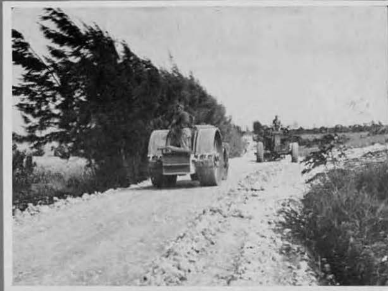
Finishing off and final shaping a coral road.
