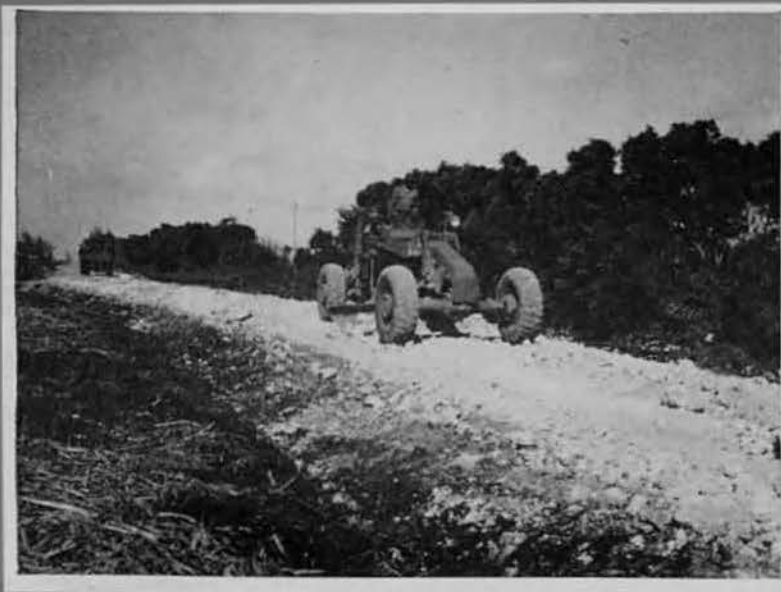
The Seabees' grader—No. 2 tool in road building.
