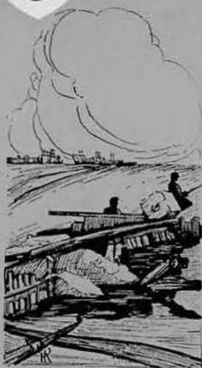
Right: Jap cement was used for the deck.
