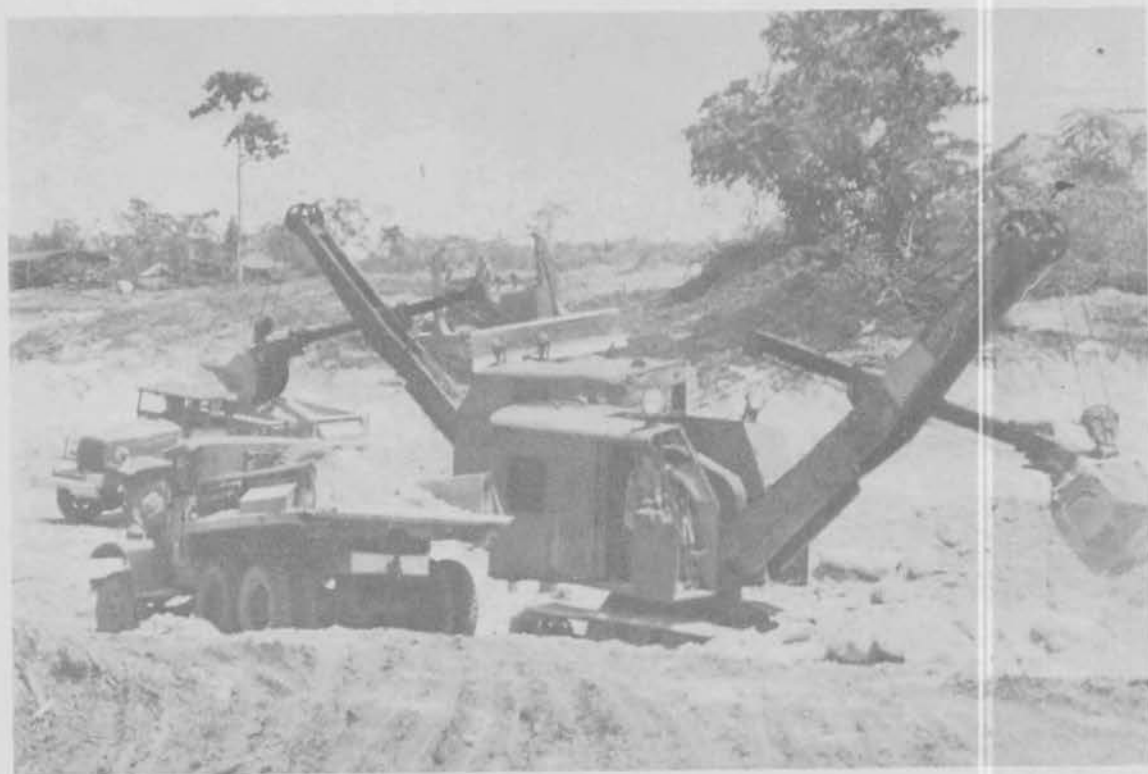
AIRSTRIP BORROW PIT
