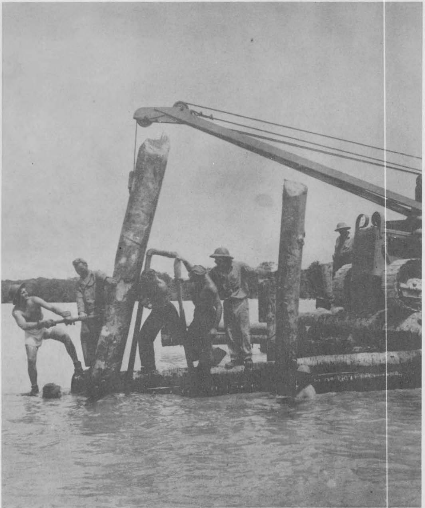
JETTING PILES FOR FINGER PIER
