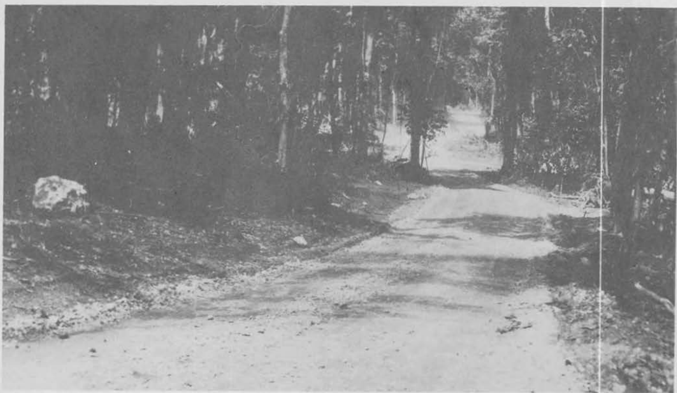
TYPICAL ROAD BUILT BY BATTALION
