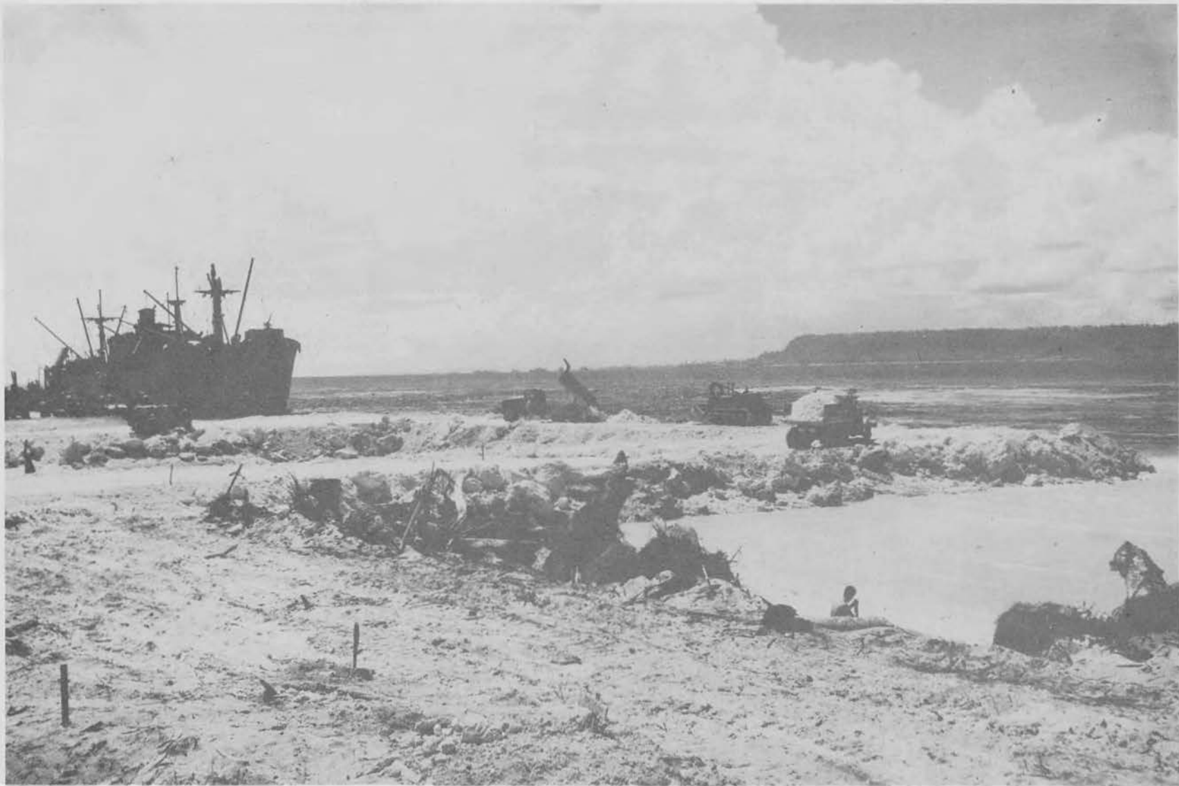
CONSTRUCTING L.S.T. JETTY
