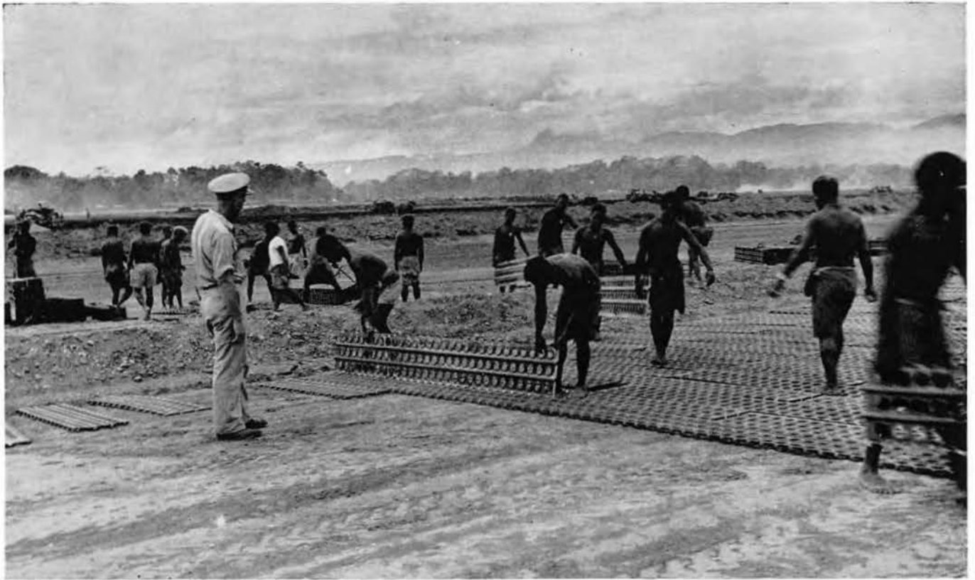
Solomon Islanders assist the 61st Seabees in laying mat on Koli Field, Guadalcanal.
