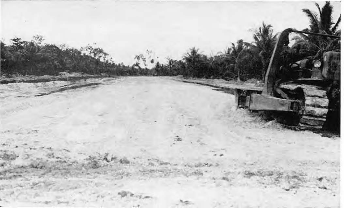
61st equipment smoothing coral for highway on Emirau Island
