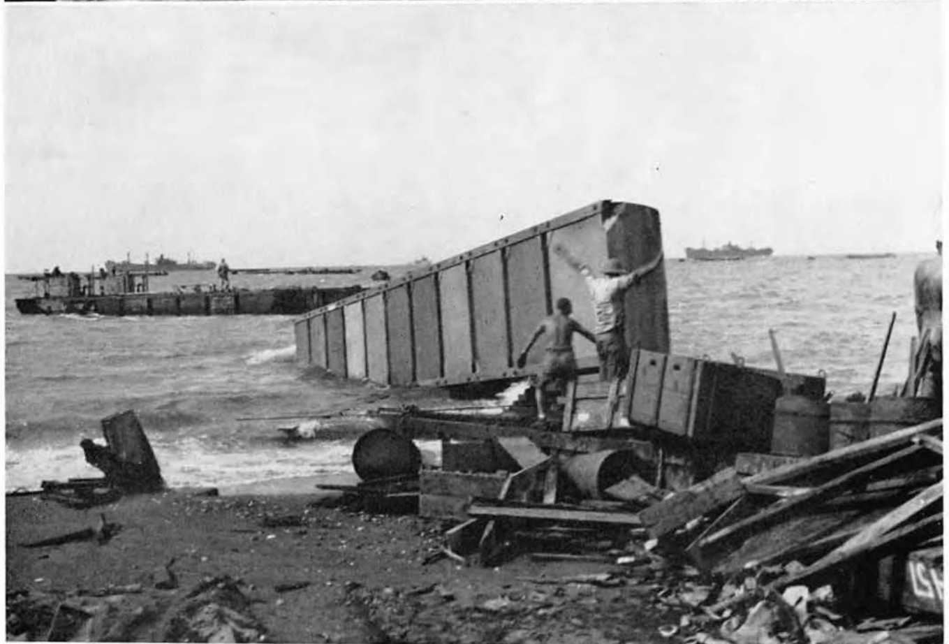
Top, Guadalcanal sawmill being operated by the 61st Seabees. Bottom, 61st pontoon crews at work on Guadalcanal.
