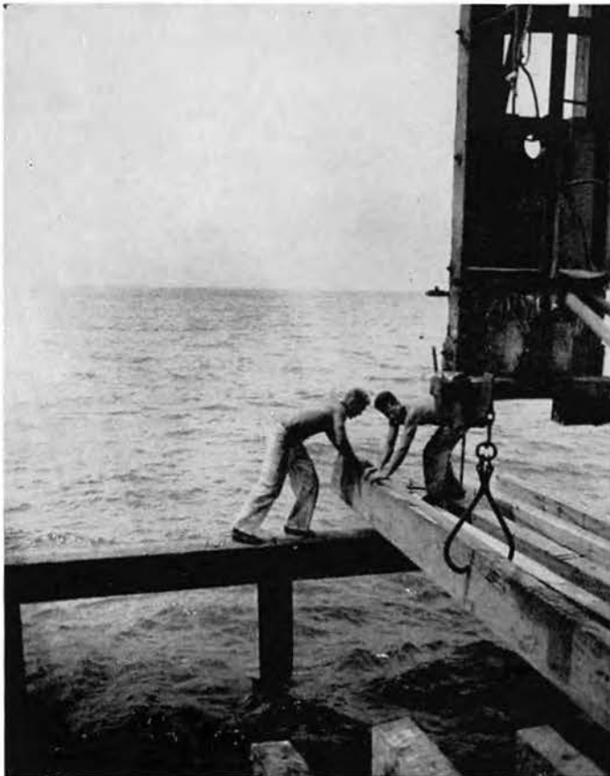
61st dock workers building a pier at Guadalcanal
