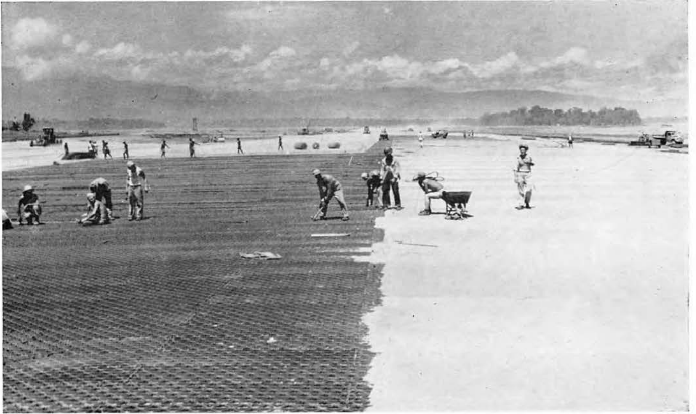
61st crews laying mat on Koli Field, Guadalcanal
