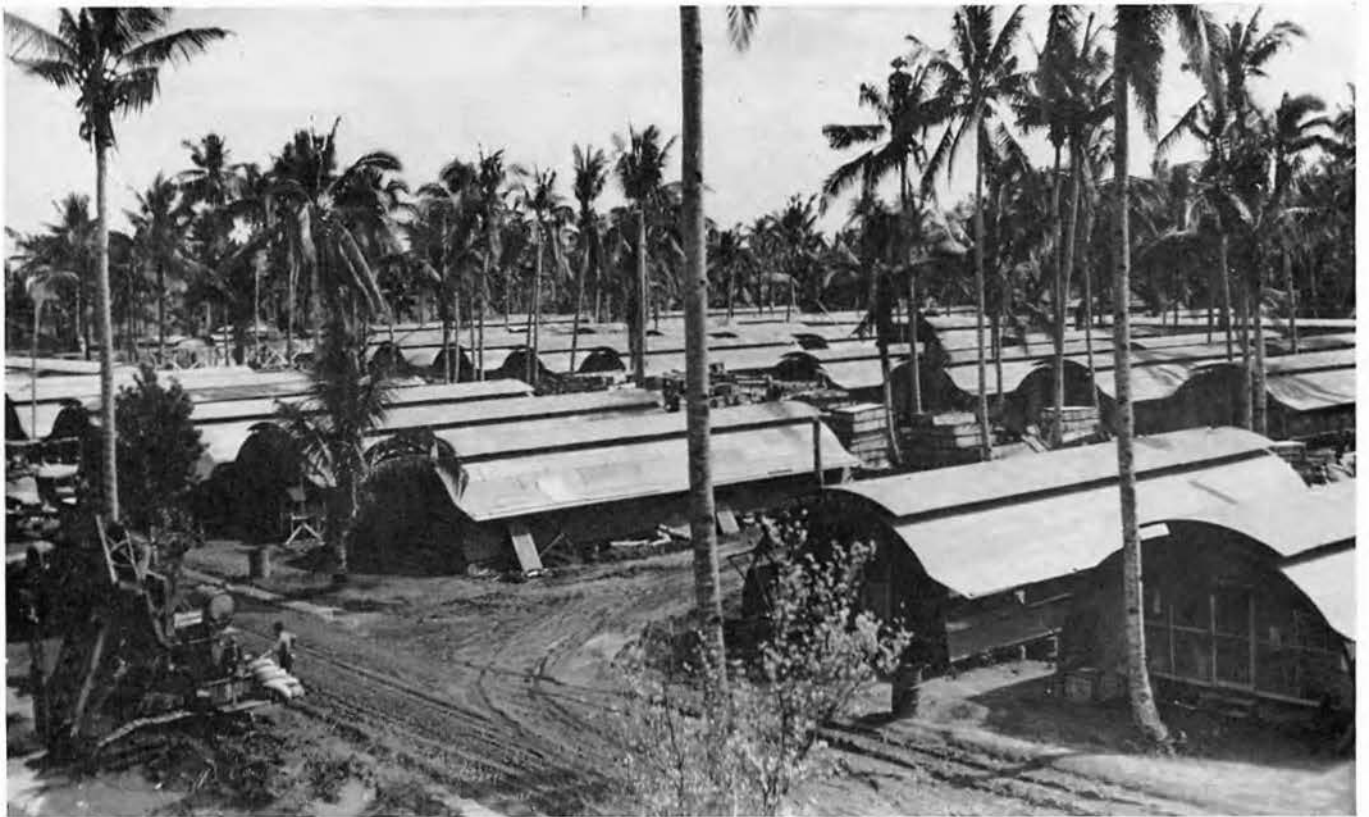
The Tolosa Quonset hut project after completion
