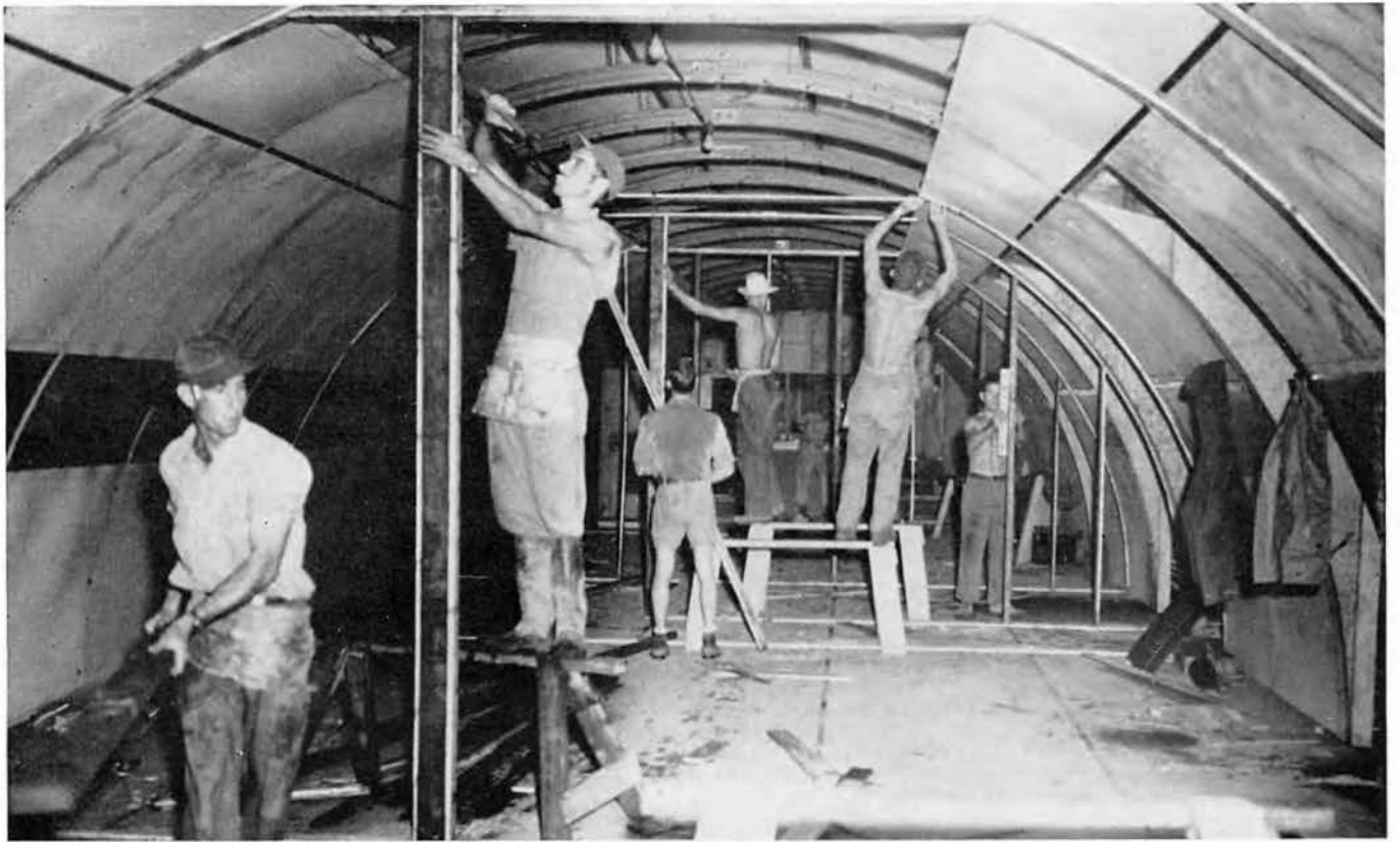
61st Seabees constructing Quonset huts at Tolosa, Leyte, P. I.
