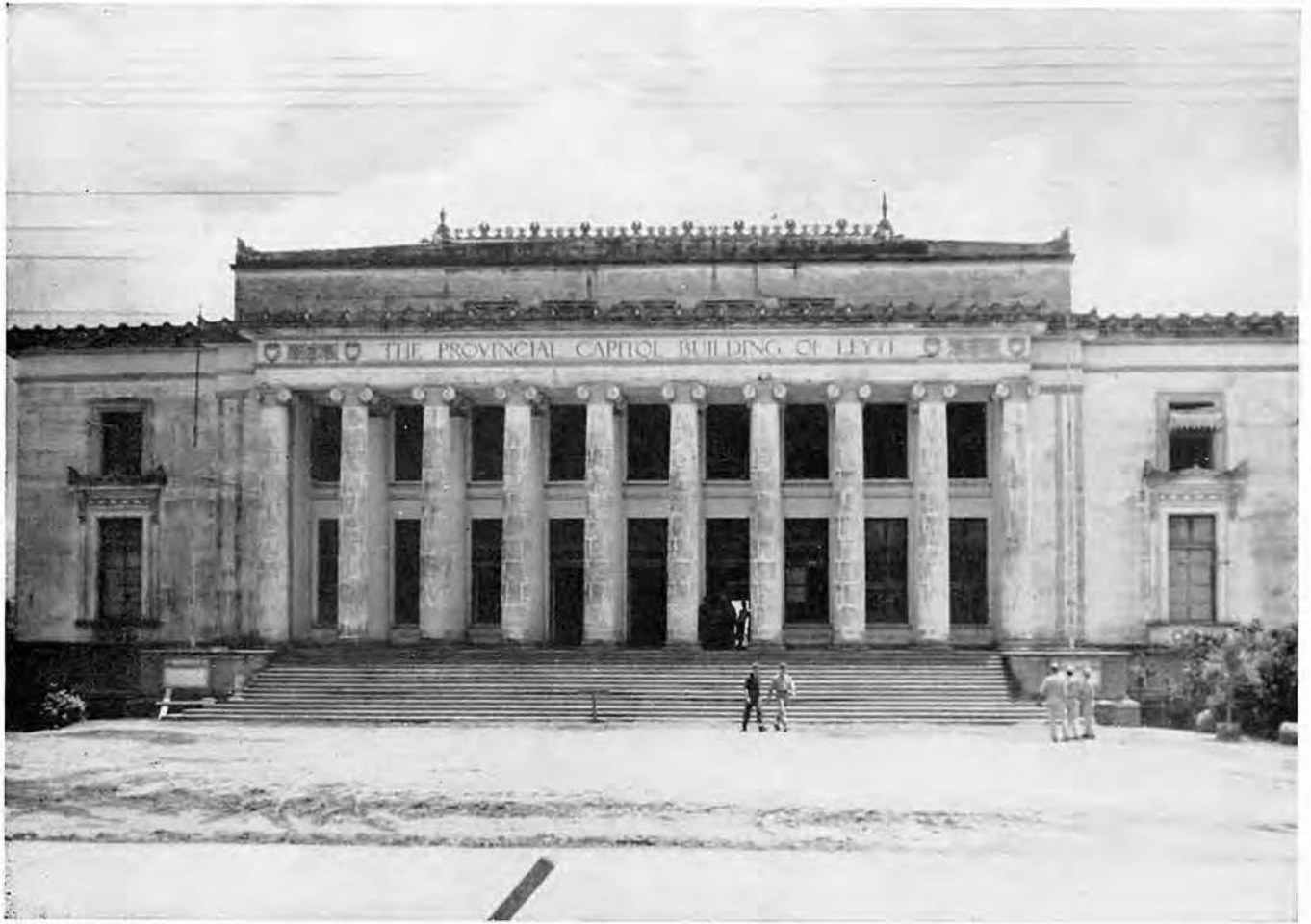
Provincial Capitol Building of Leyte Island, at Tacloban
