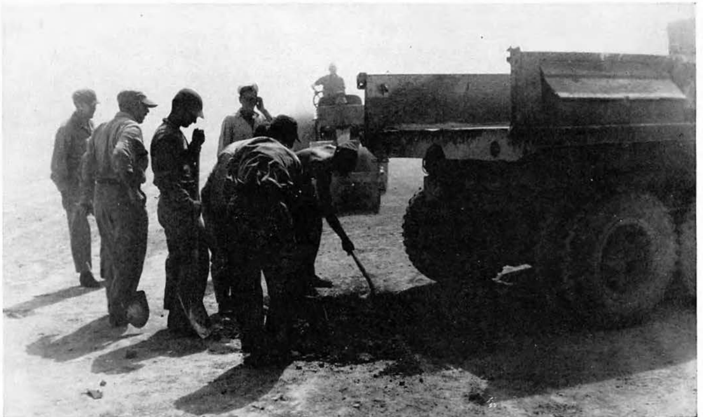
Airfield maintenance crew filling in a bomb crater on a Samar Island airstrip
