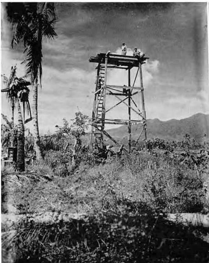
Construction of tower on San Pablo Strip, Leyte, P. I.
