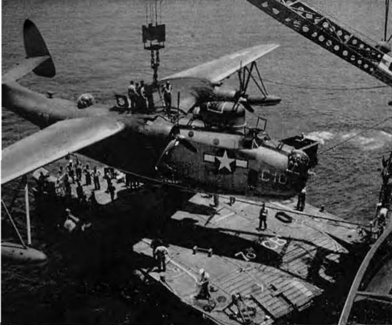
A P.B.M. is lowered into barge
