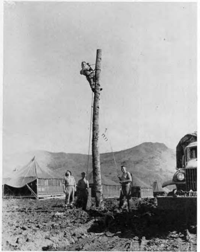
Erection of power lines
