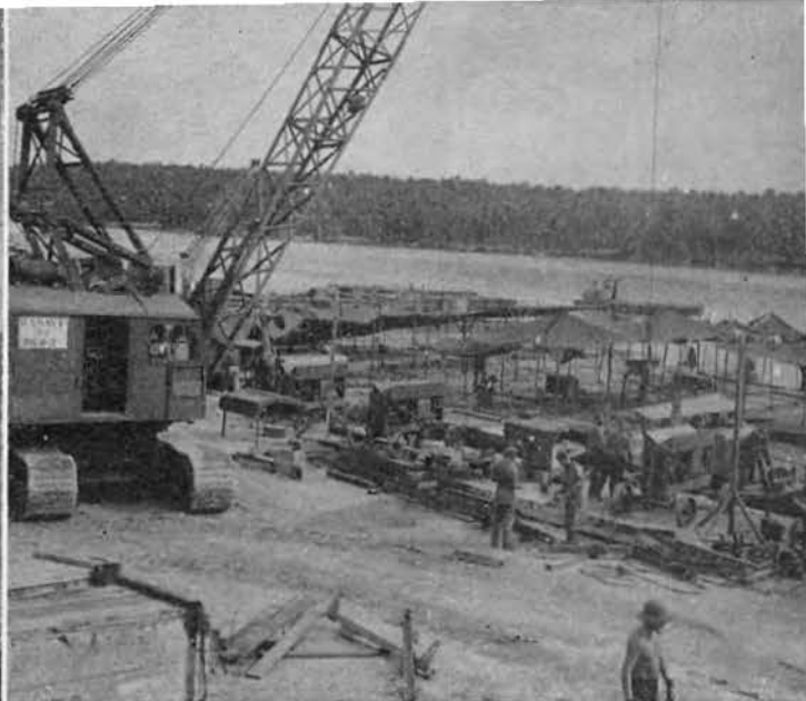
Barge outfitting yard
