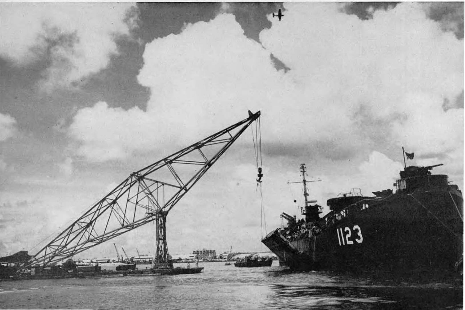
75 Ton crane raising barge on side of LST
