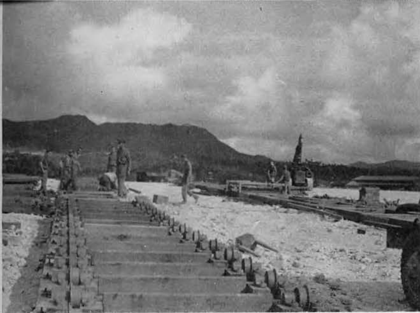
Pontoon yard, launching ways
