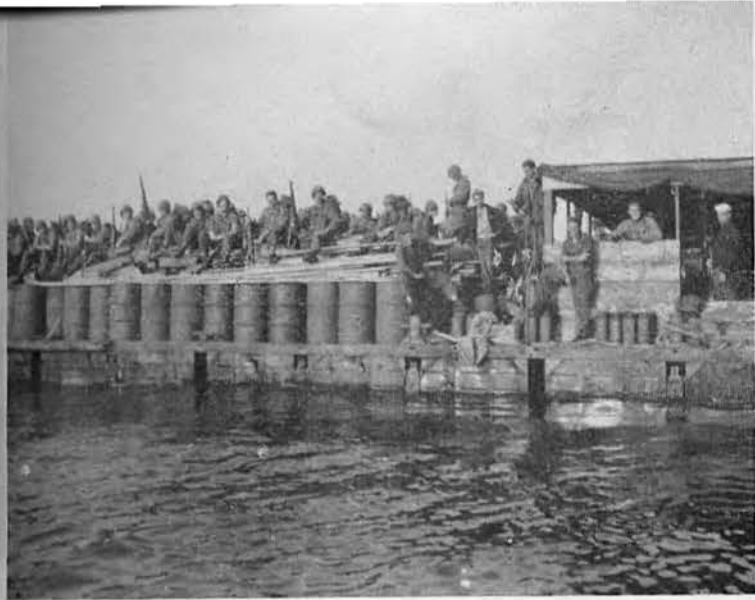
Barge loaded with engineers being taken ashore by CB's
