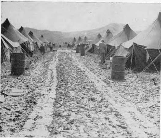
Typical camp street before surfacing
