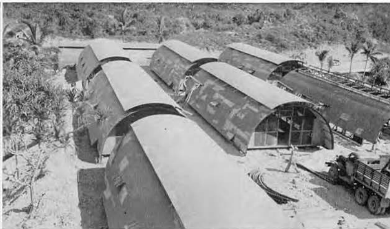
Below: Adcomphibspac quonset hut construction Bottom: Harman Field Administration Building
