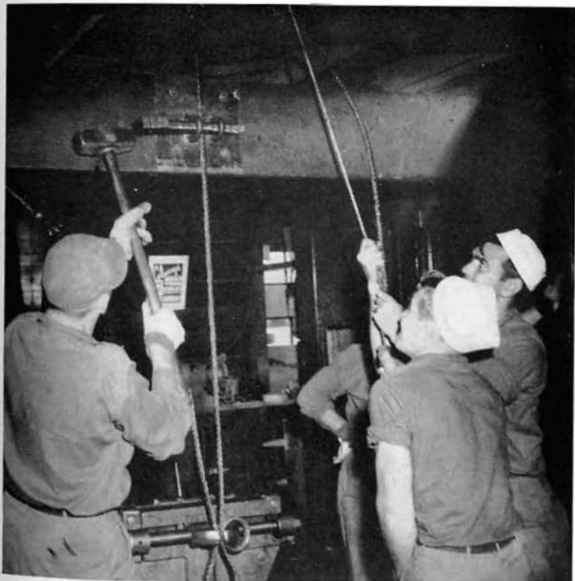
Right: Splicing wire in the rigging school. Above: Securing cable in preparation for a splice.
