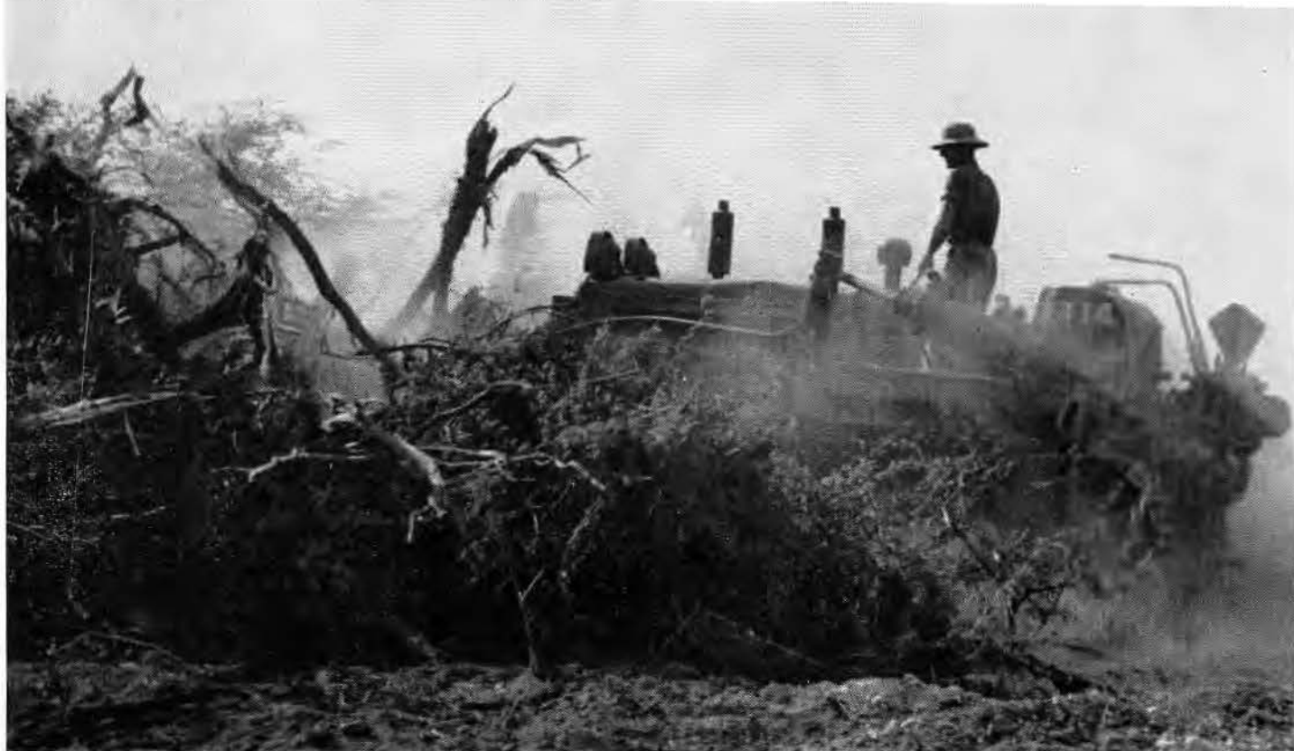
The jungle doesn't stand a chance against this Seabee equipment.
