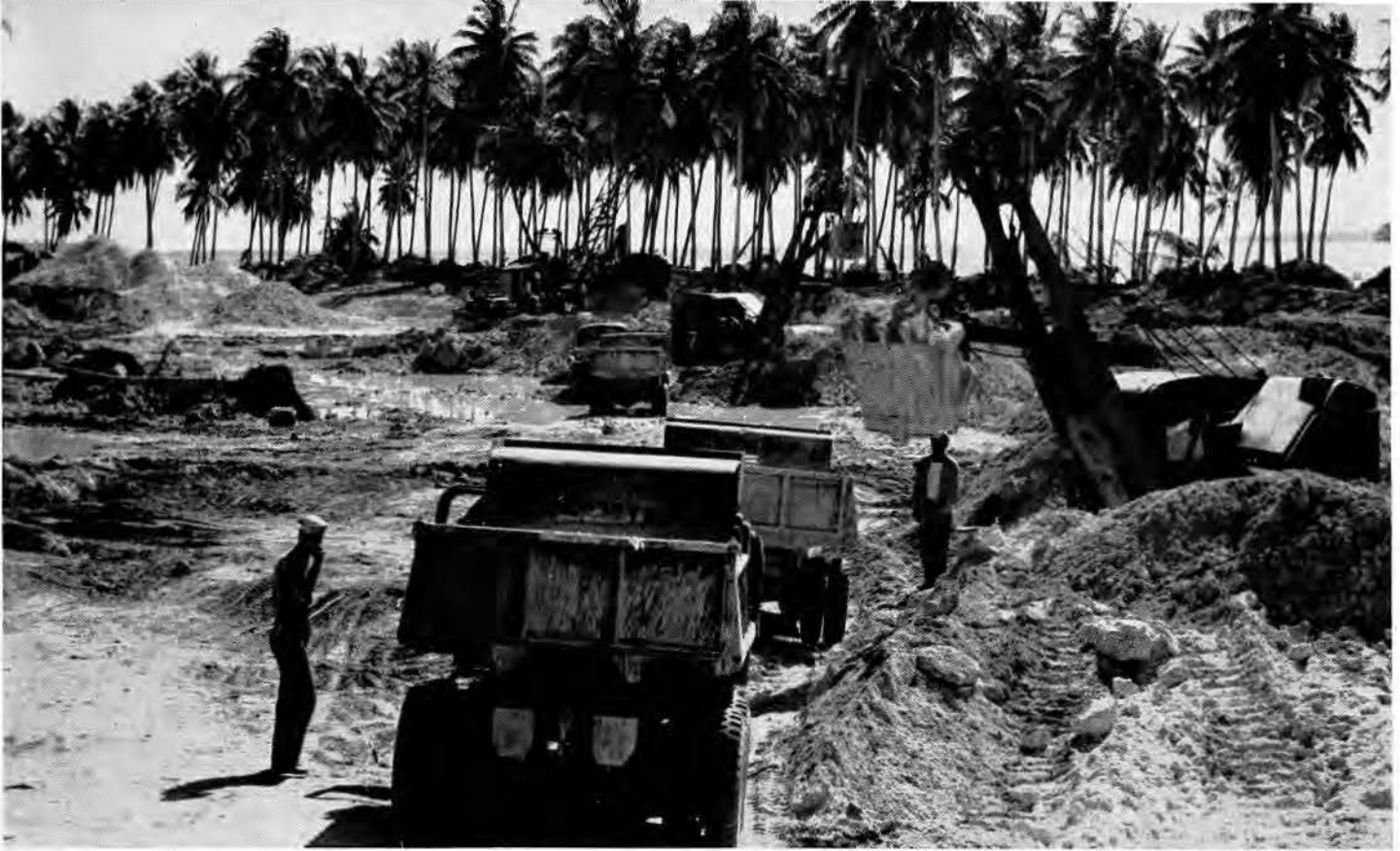
This is the Bougainville airstrip, in preparation.
