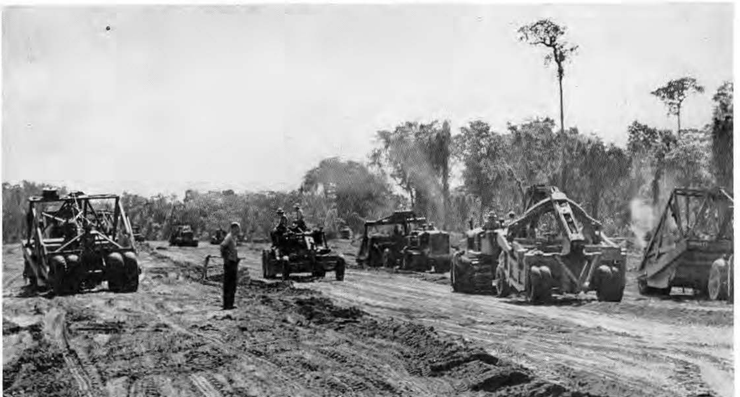
This is the Bougainville airstrip in preparation.
