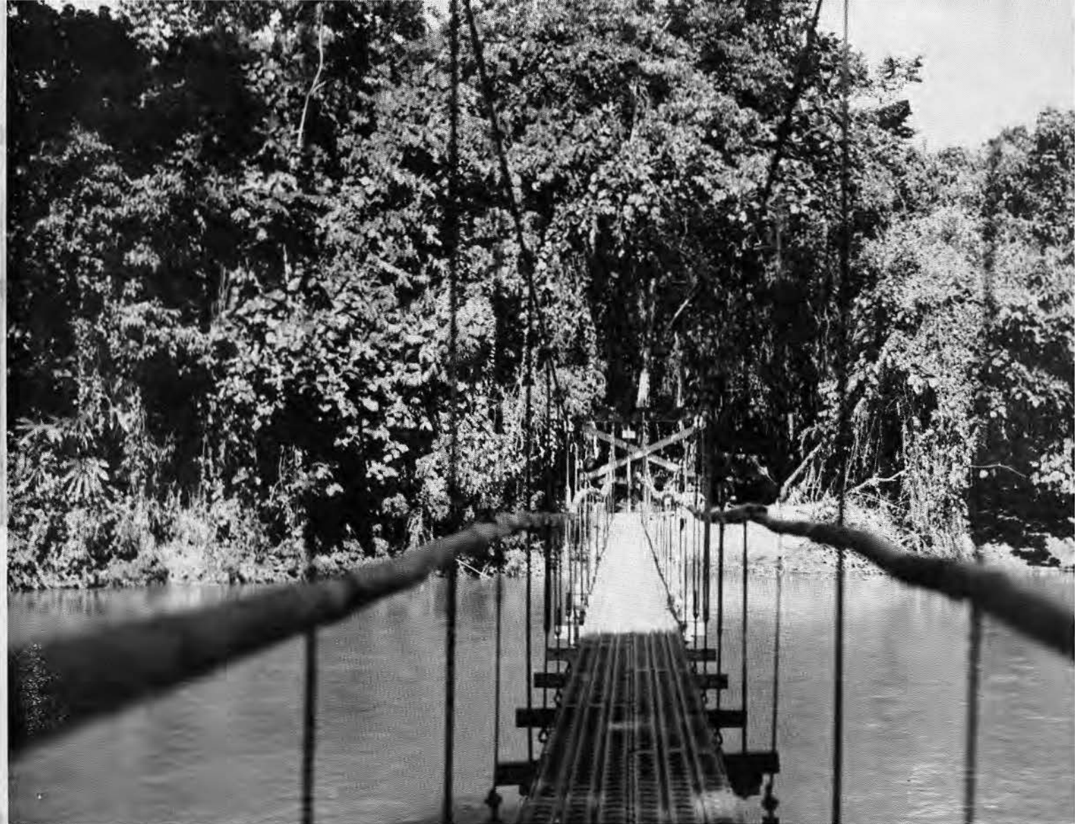
Above: That old motto, "Don't cross your bridges . . ." doesn't mean much to the Seabees—they're always coming to them, and in a hurry. This one, over a river on Guadalcanal, was erected in a day and a half. Flooring is pierced plank, handrails are of native bamboo, and the end towers were bents from a portable military engineer bridge.
