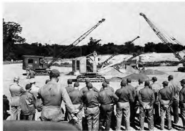
The Bulldozers and Draglines Levelled the Fields in Record Time.
