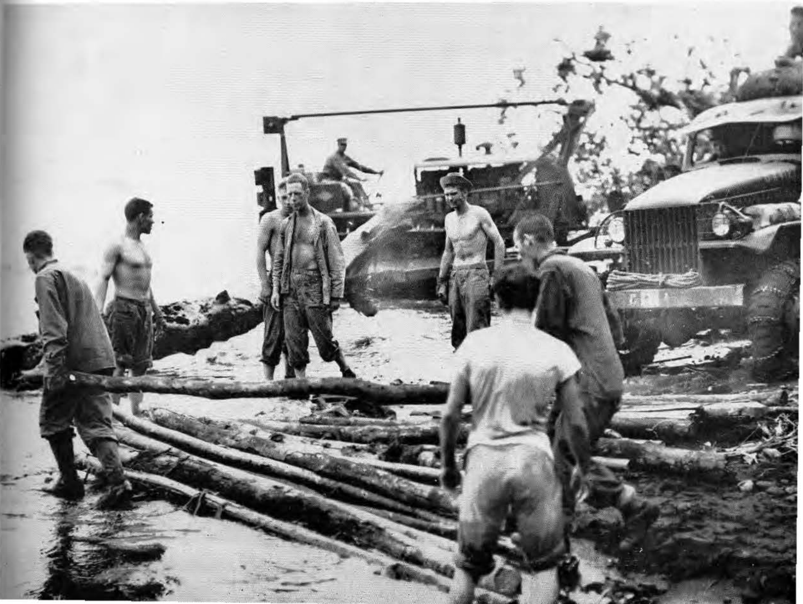
Trees and logs are put in place by Marines and Seabees for a bridge across a jungle stream on New Britain Island.
