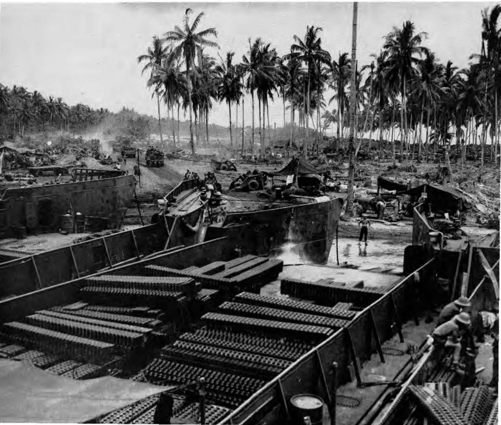
Seabees unload their supplies and equipment, to clear the jungles, roll the airport and put the metal strips together to form an airfield. The scene is in the Bougainville jungles.
