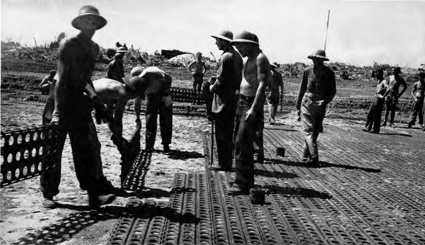
A close-up of Seabees laying Marston mat in Bougainville. Planes will shortly be landing on it and taking off from it.
