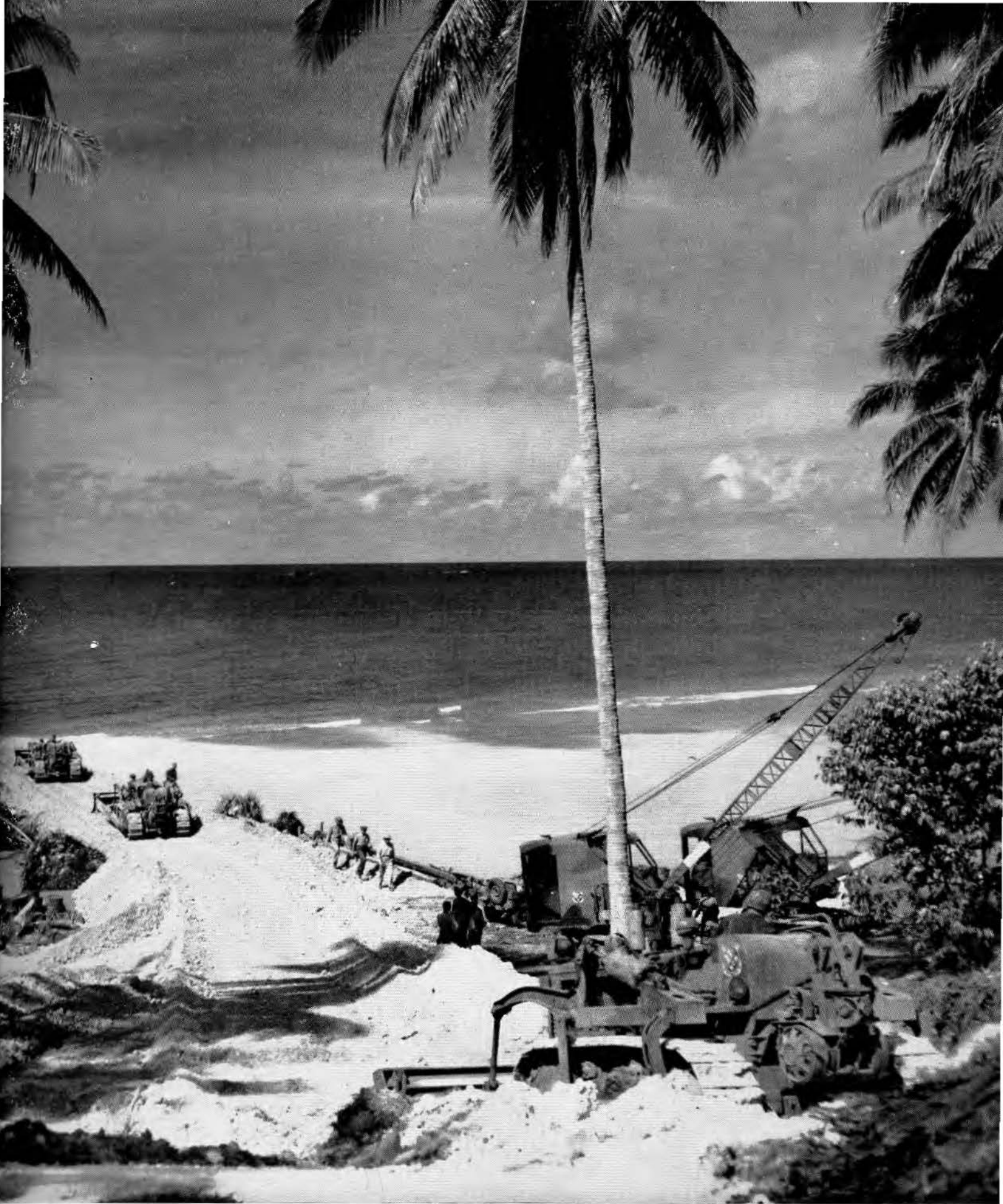
Bulldozers clear a road to the site where a dock will be built on Emirau Island, to facilitate unloading of LSTs (Landing Ship, Tank).
