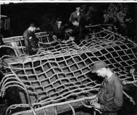
Cargo Net Repair.
