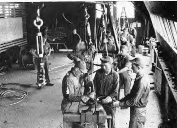
Splicing the heavy cables is a job that requires steady, skillful hands.
