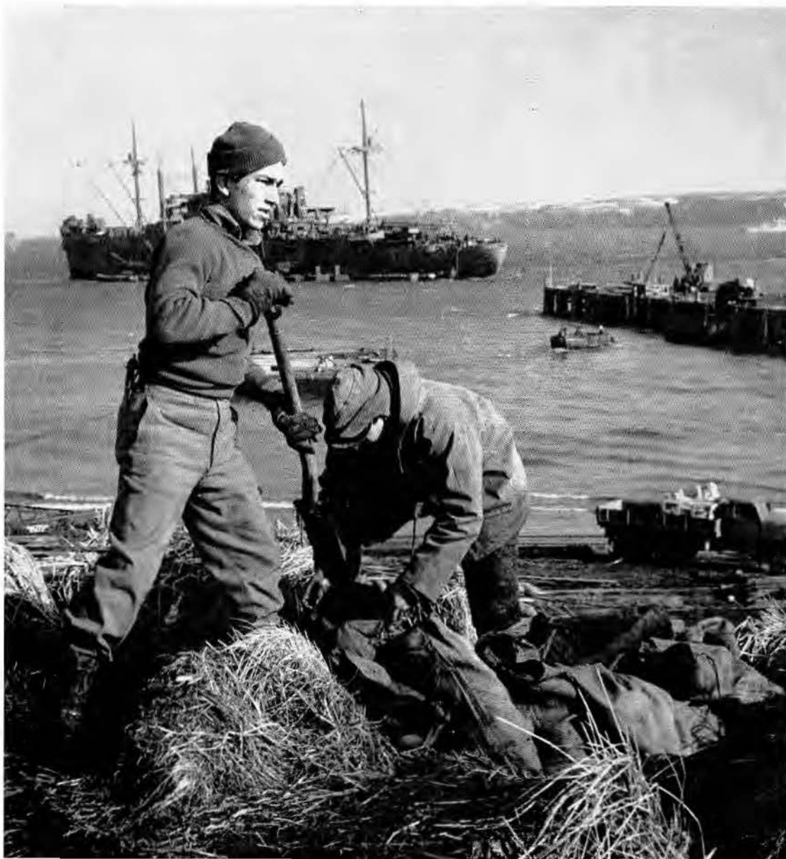
Warmly-clad Seabees fill sandbags for a machine gun emplacement on Amchitka in the Aleutians during the spring of 1943.
