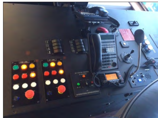
Figure 2D-4. Alarm Panel.
