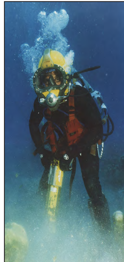
Figure 6-4. Underwater Construction Diving.
