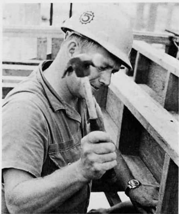
ABOVE LEFT: BU2 Carleton "Mac" McKenney adjusts tamper used to compact the ground before a concrete pour. LEFT: BU2 Don Underwood forms up the roof for an overhead pour. ABOVE: BU1 Ricardo Amposta and BU3 Dan Foster, Greeley, Colo., position and steady a concrete bucket on an overhead pour.
