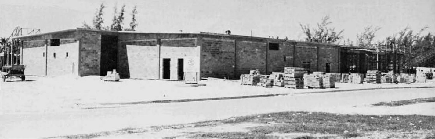
The subsistence building showing progress through late April. When FIVE arrived, only 15 of the 53 columns were in place, and some of the underground utilities were present. FIVE left with the overhead poured, most of the deck slabs in place, and a good start toward the completion of the exterior block walls.
