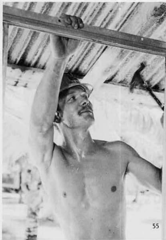
BU3 Rickey "Flu-Flung" Rapp rehabs office spaces in preparation for Naval Construction Forces due in.
