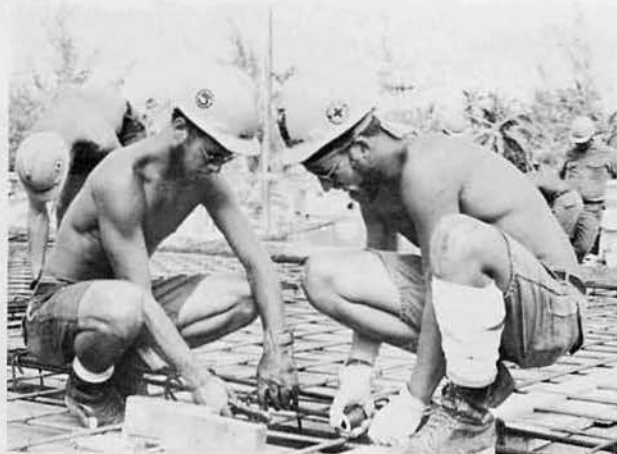
SW3 Lance Carver, Craig, Colo., sets high chairs on subsistence building roof beams.
