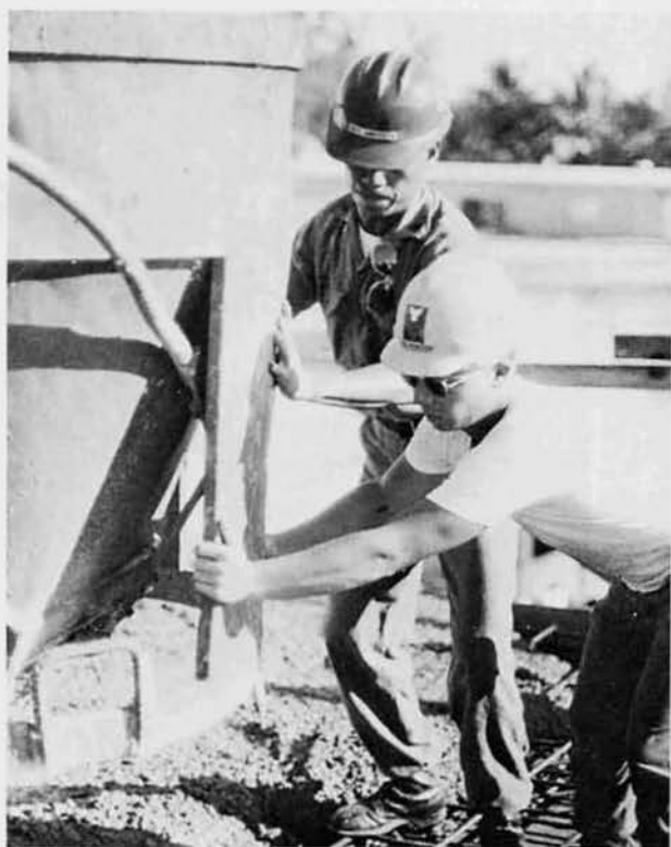
ABOVE LEFT: BU2 Carleton "Mac" McKenney adjusts tamper used to compact the ground before a concrete pour. LEFT: BU2 Don Underwood forms up the roof for an overhead pour. ABOVE: BU1 Ricardo Amposta and BU3 Dan Foster, Greeley, Colo., position and steady a concrete bucket on an overhead pour.
