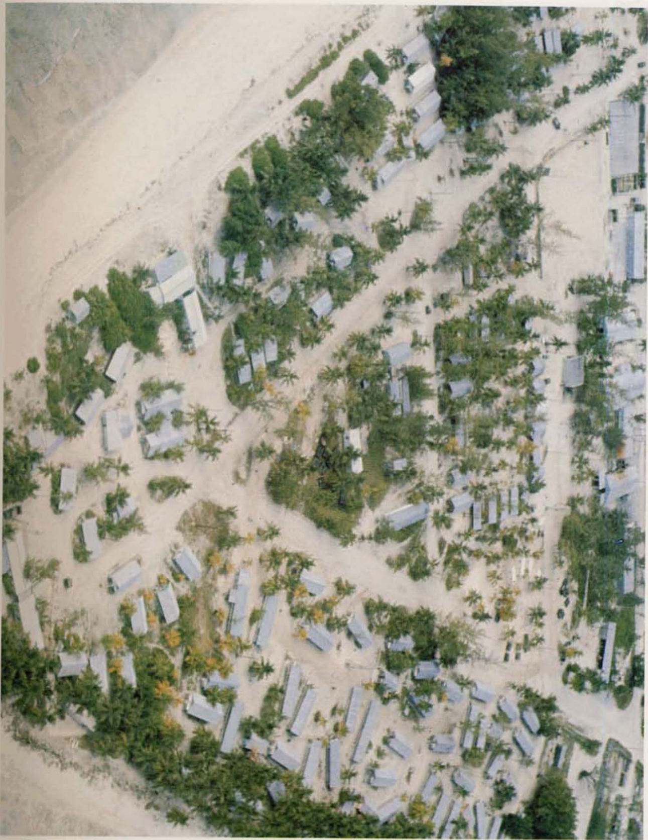
Camp C. S. Cummins, home for NMCB-FIVE and the Naval Construction Force on Diego Garcia. Aerial photos were taken January 17, 1976.
