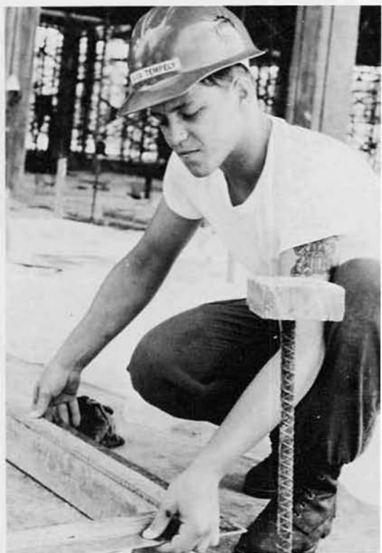
RIGHT: BUCA Mike Temperly, Galena, Ill., squares up form for a floating slab.
