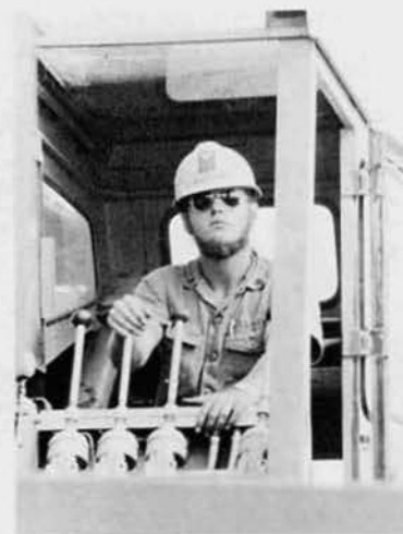
EO3 Bob Hanke, Jayton, Texas, on the 50-ton Lima, the biggest crane in the yard.
