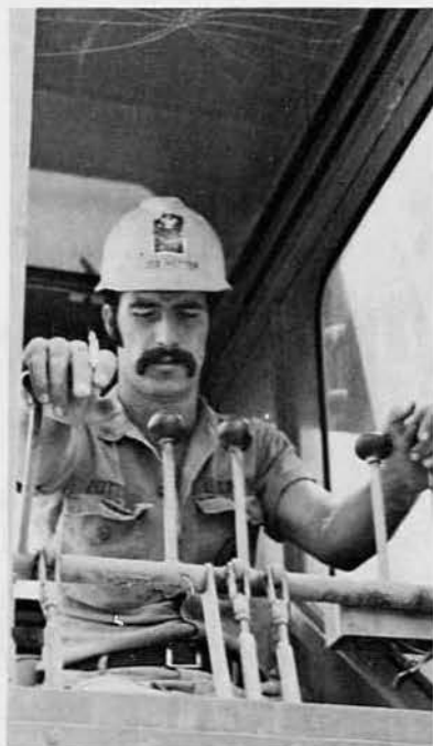
EO3 Chris Potter, Scotts Valley, Calif., at the controls of a Telescope cleaning up a cement spill at the silos.
