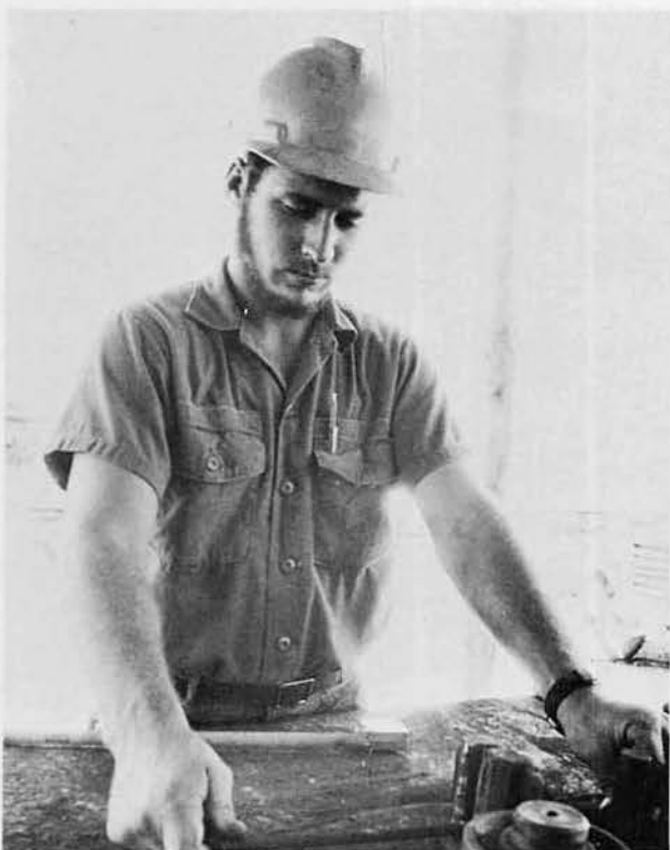
SW3 Jim Russell, Newman, Ca. , bends rebar at the pre-fab yard.
