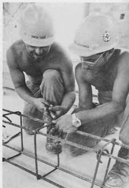
SWCA Billy Cook, Baytown, Texas, and SWCN Philip Latronica, Los Banos, Ca., make a rebar cage for a lintel at the chapel.
