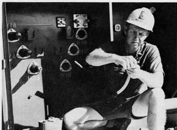
CE2 Joel Barber just cut his finger working on the I-level maintenance generator.
