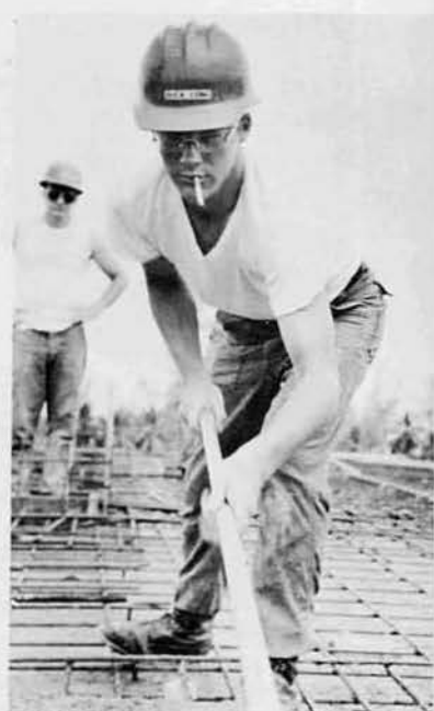
BUCA Scott Long, Bernville, Pa. , spreads concrete during an overhead pour.
