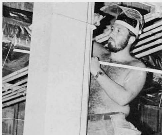
BUCN Gregg Zellers, Denver, Colo., aligns edge angle strips for the NEX suspended ceiling.
