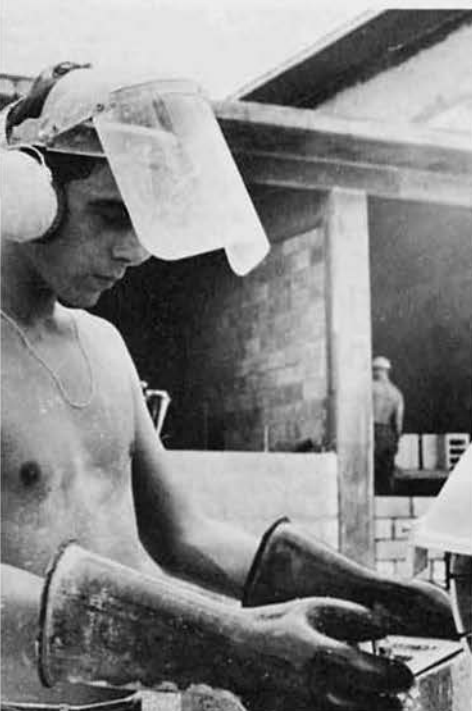
LEFT: BUCN Robert Thomas, Coshocton, Ohio, cuts 12" block for weight room and office space walls.
