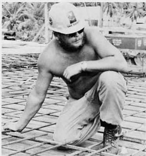
SW3 Bill Everett, Cabool, Mo., places the second rebar mat in place on the sub building roof. RIGHT: SW3 Don "Whitey" White, Oxnard, Ca., helps move the second mat into place.
