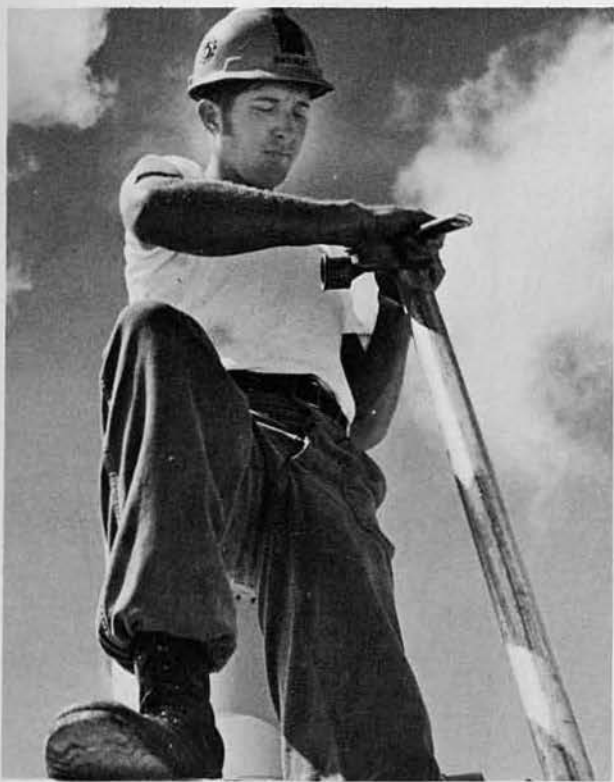
SW3 David Riley, Granger, Utah, installs fence post at the incinerator.
