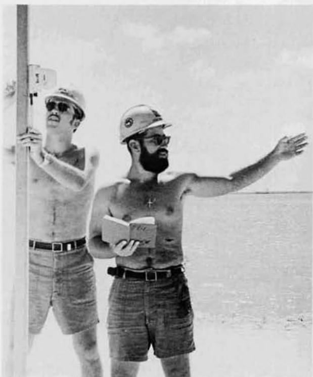
EA3 Kevin White, Raleigh, N. C., and EA2 Marty Miranda, Pinos Altos, N. M., with the laser plane Philadelphia rod, which senses the laser beam.
