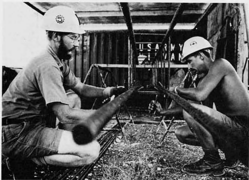
TOP LEFT: SWCN Dave Ahrens, Yuba City, Ca., and SW3 Bob "Pete" Peterson, Montgomery, Ala., tie the first rebar mat. TOP RIGHT: SWCN Dave Ahrens and SWCN Ray Herbine, West Lawn, Pa., also tie the first mat. RIGHT: SW3 Vic Joy, York, Neb., and SW2 Mike "Sandy" Sancrant, Anacortes, Wash., tie cages for roof beams.
