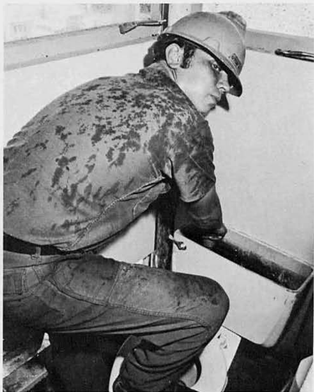
UTCN Tim "Buddy" Hopkins, Crystal, Minn. , fixes a toilet tank. The salt water flushing system caused many problems.
