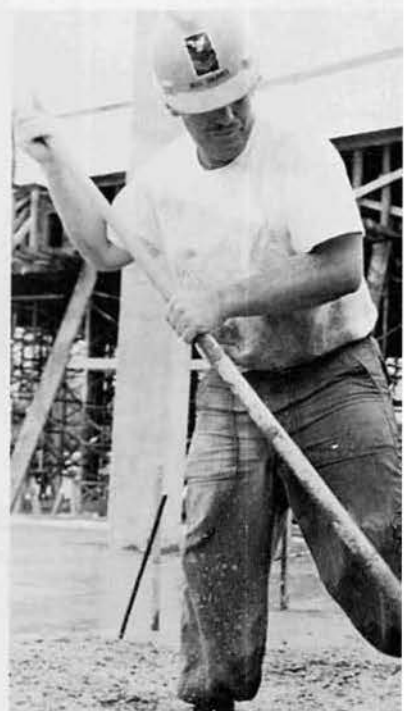
BU2 Joe Graves, Shelbyville, Mich., spreads concrete on a slab pour.
