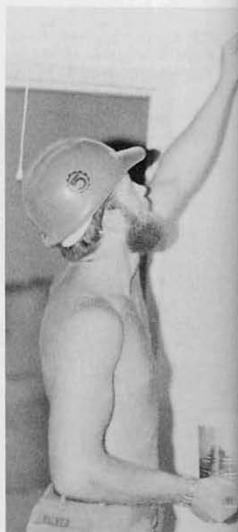
BUCA Freddie Walker, Doniphan, Mo., applies rubber-base paint to the walls.
