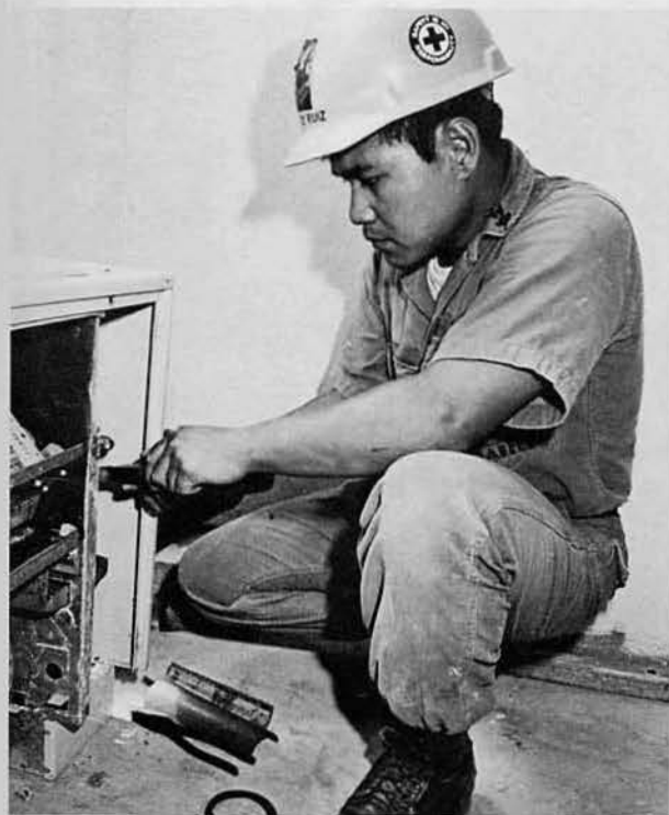
UT2 Constantine Ruiz insulates pipes on a chapel air conditioning unit.
