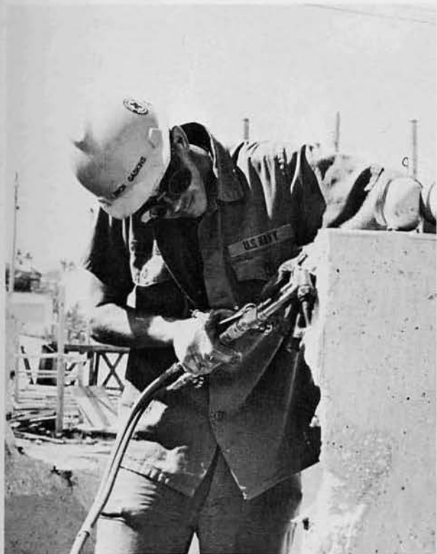
SW3 Len Gaskins, Lake City, S. C. , cuts rebar in converting a man-hole into a weir sump for the POL farm.
