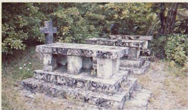
Some of the graves are above ground because of the high water table.
