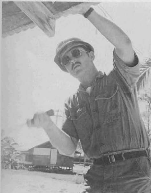
BU3 Billy Stanfill, Grants Pass, Ore., repairs a SEA hut roof.
