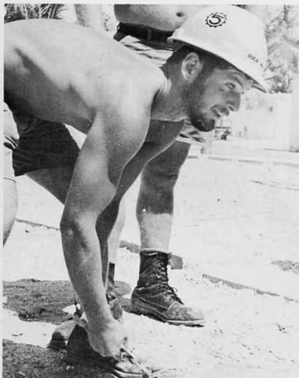
BUCA Perry Mace, New Castle, Dela. , pulls stakes holding sidewalk forms in place.
