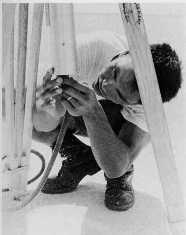
EA3 Gene Taday plugs the laser plane into the battery.
