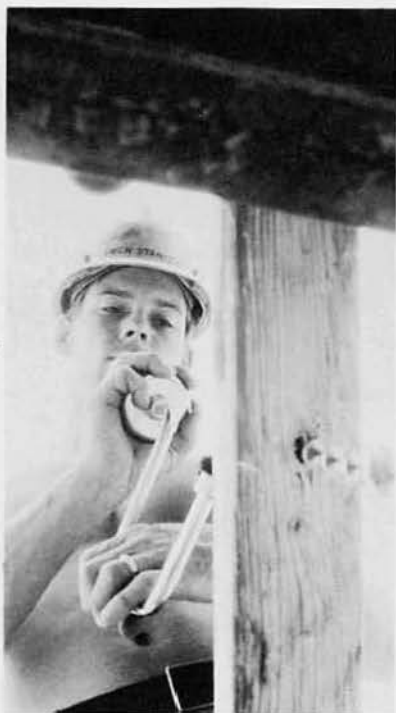
SWCN Steve Stancer, Rio, Wis., uses a brace and bit to form a dead man brace at the incinerator.
