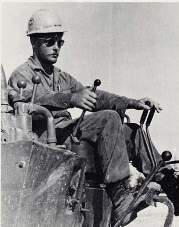
EOCA Loyd Hastings, Morristown, Ariz., atop a top a TD-20 dozer.
