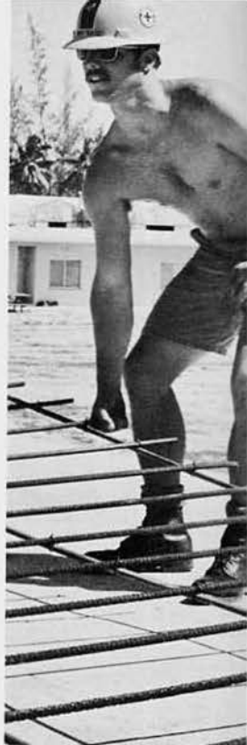
SW3 Bill Everett, Cabool, Mo., places the second rebar mat in place on the sub building roof. RIGHT: SW3 Don "Whitey" White, Oxnard, Ca., helps move the second mat into place.
