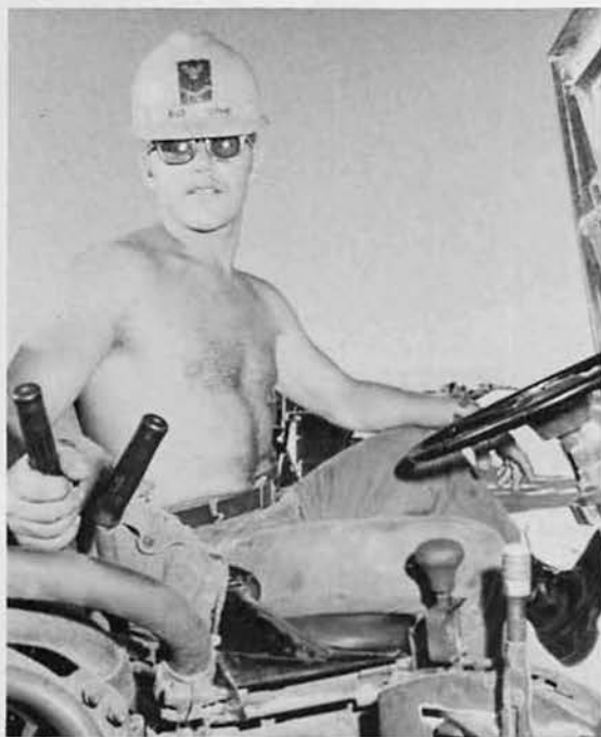
EO3 Steve "Wedge" Josephs on an MRS side dump. He was the asphalt finisher operator for the battalion.
