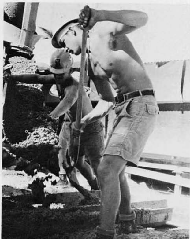
BU2 Glenn "Sonny" Dailey, Worcester, Vt. , and BUCN Dennis Robillard, Springfield, Ore. , pour porta-camp sidewalks.
