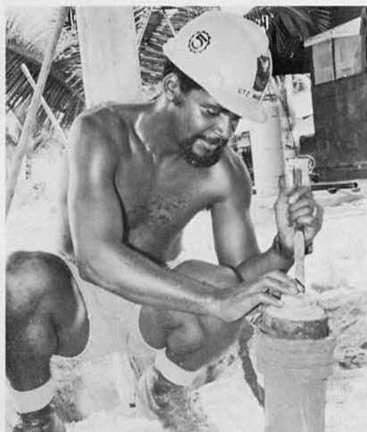
UT2 Clarence "C.W." Warden, New Castle, Pa., oakums a cast iron porta-head joint.
