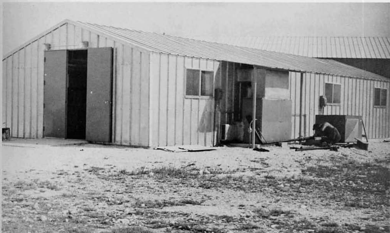
One of the smaller projects finished early in the deployment was the I-Level Maintenance facility at the airfield. FIVE arrived to find the footings in place, and Echo Co. had it completed by year's end. The project supervisor was SW1 Bobby Hamlett, Clovis, N.M.
