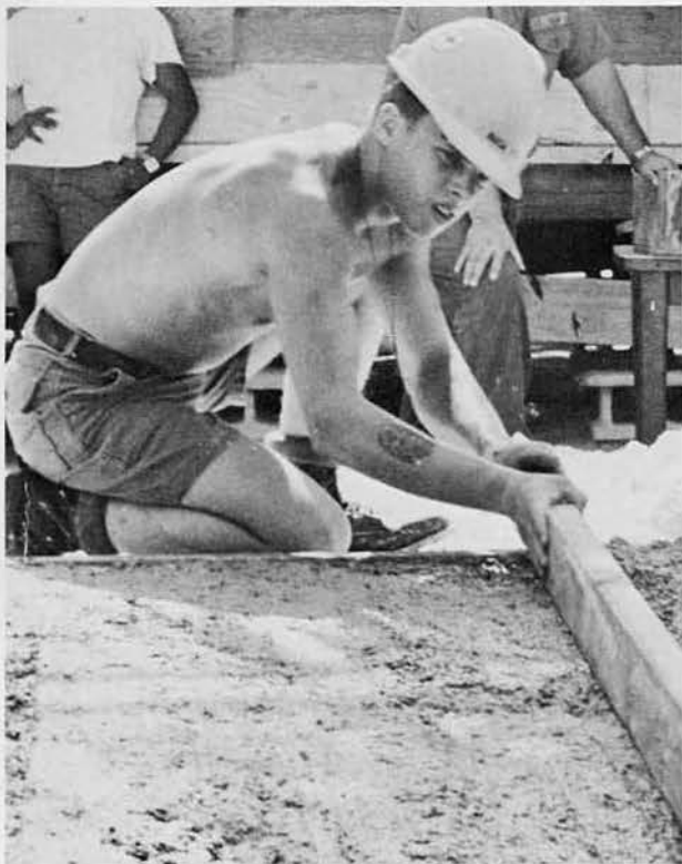
BUCA Perry Fish, Corry, Pa., screeds a porta-head pad.
