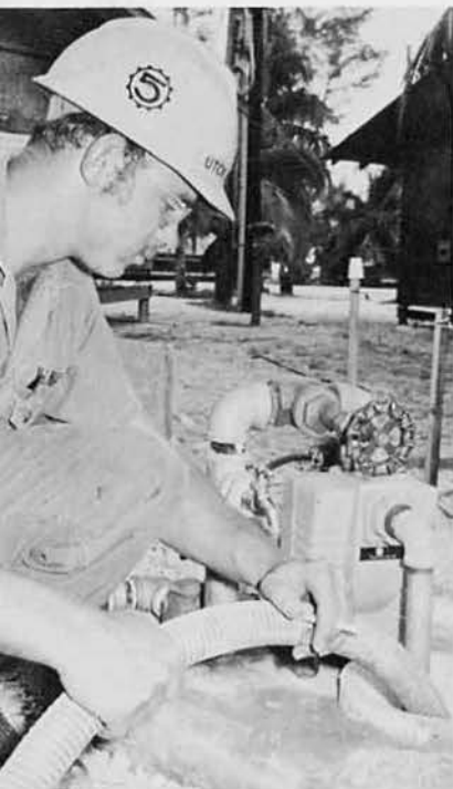
UTCN Gerry "Willie Wonka" Williams, Lawton, Okla., super-chlorinates the water in a new quadrangle well to purify it.
