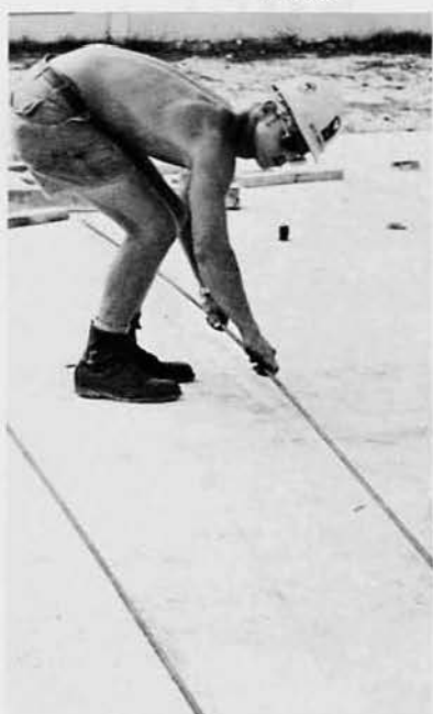
BU3 Bob Haverkost lays out rebar for the roof slab.
