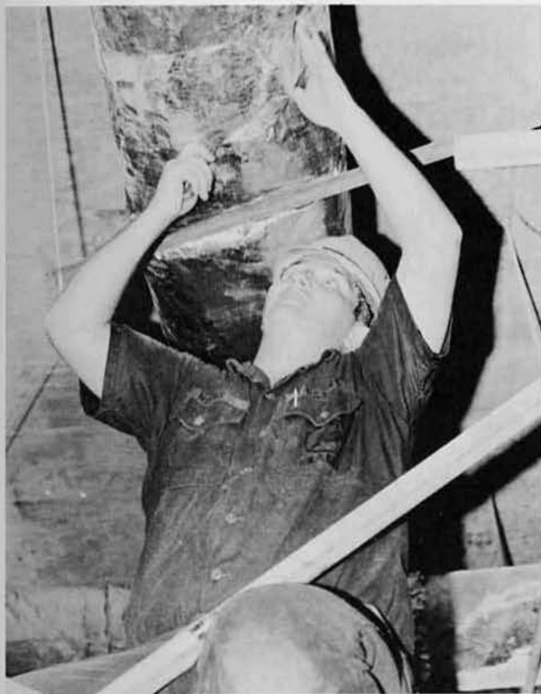
SWCA Jerry Woods, Red Hook, N.Y., adjusts insulation on ductwork at the NEX.
