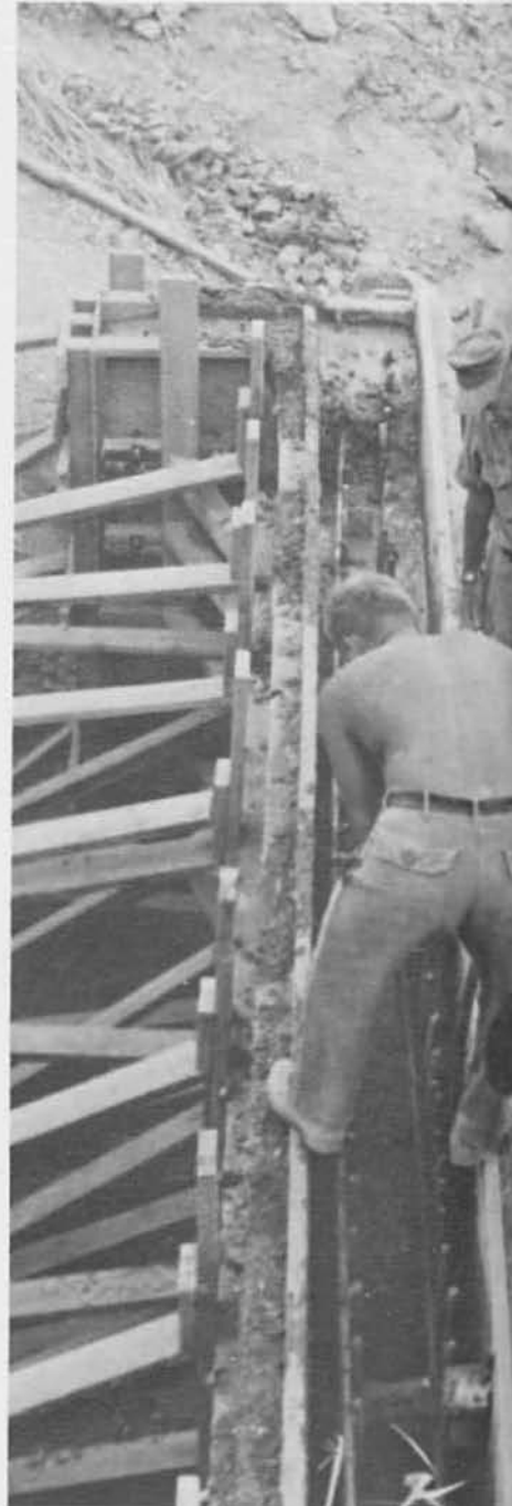
Far right: BU2 Duane Vance, BUCN Joseph Mazza and BU3 John Lang prepare a form for a concrete spillway at a culvert on Route #9. Center top: SN Tom Fritsch and BU3 James Cusato help swing a concrete culvert top into place on Route #9. Above: BUCN Weldon Scott, BU3 James Cusato and BU2 Joseph Lisuzzo build forms for concrete culverts at Elliott Combat Base. Right: A Charlie Company crew headed by BUC Frank Vollono prepares forms for the next pour.
