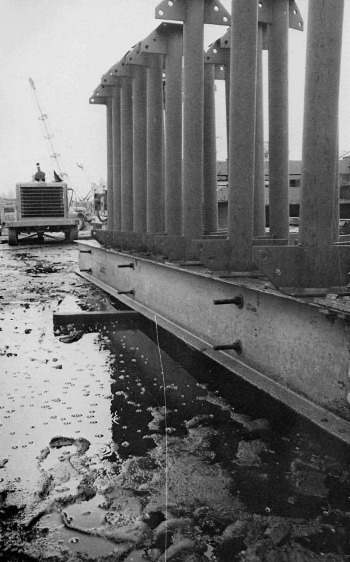
Above: Bridge components were prefabricated on the muddy bank of the Bo Dieu River. Right: Then they were bolted in place to form the trestles to support the mammoth structure. Far right: a traditional topping out ceremony marked the placing of the last girder. Top: Needing only the timber decking to be complete, the Dong Ha Bridge dwarfs the rickety, one-lane French structure it will replace.
