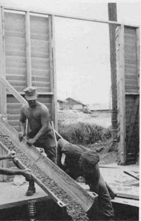
Top: A Detail Barracuda crew places concrete for a culvert endwall on Rt. #9. Middle left: A concrete grease rack is poured for Force Logistics Support Group Bravo at Dong Ha. Middle right: Delta men precast endwalls in Camp Barnes' precast yard. Left: A crew pours a concrete slab for a generator shed in Camp Barnes.
