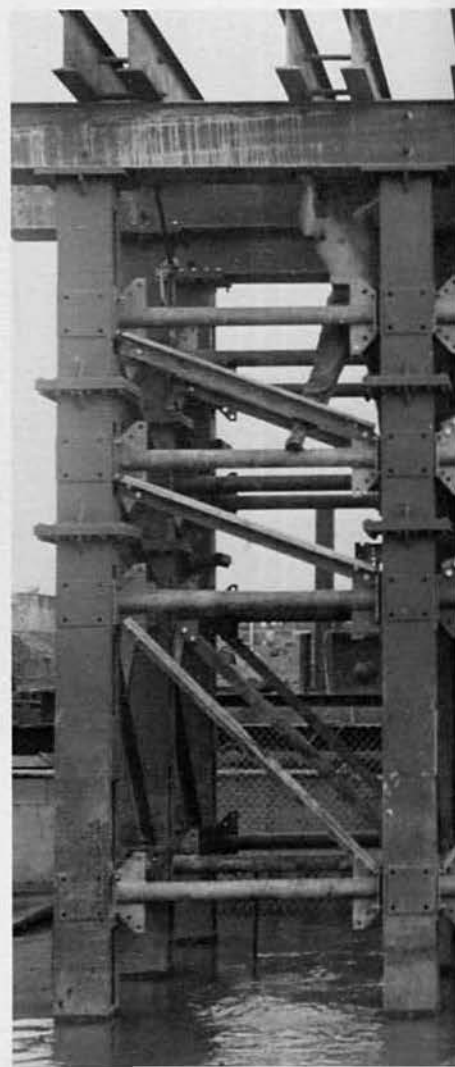
Above: Bridge components were prefabricated on the muddy bank of the Bo Dieu River. Right: Then they were bolted in place to form the trestles to support the mammoth structure. Far right: a traditional topping out ceremony marked the placing of the last girder. Top: Needing only the timber decking to be complete, the Dong Ha Bridge dwarfs the rickety, one-lane French structure it will replace.
