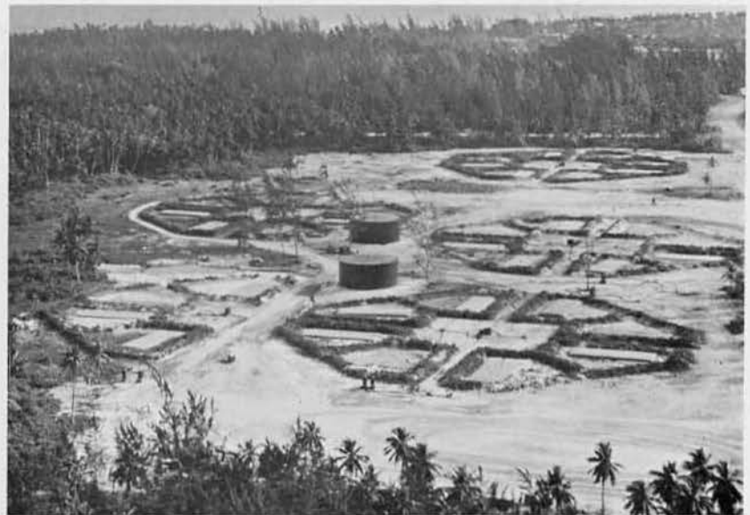
The partially completed temporary POL Facility
