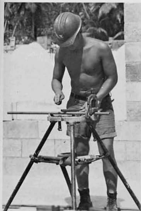
Plumbing work at BEQ 2.
