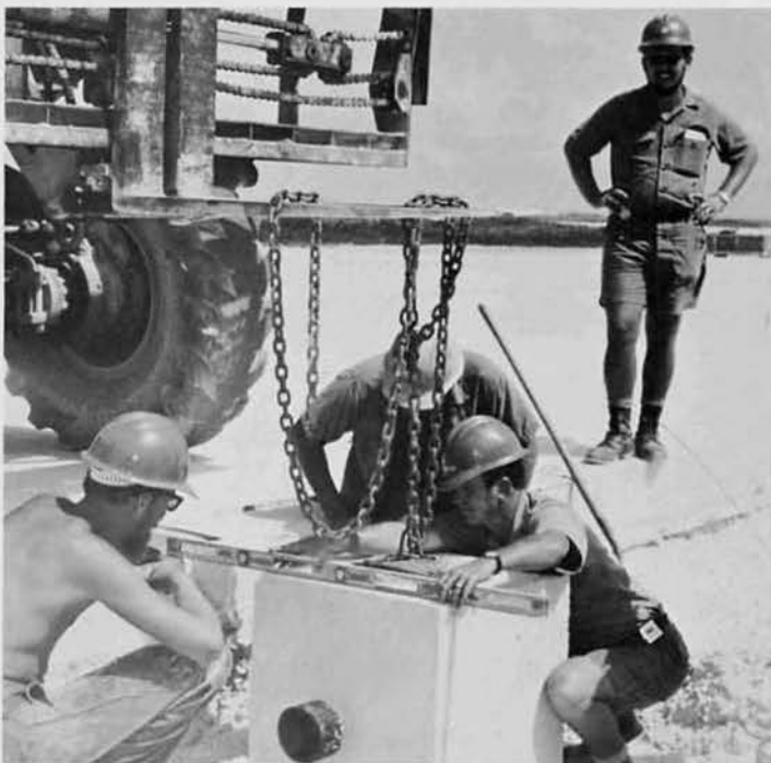
Setting light bases at the taxiway
