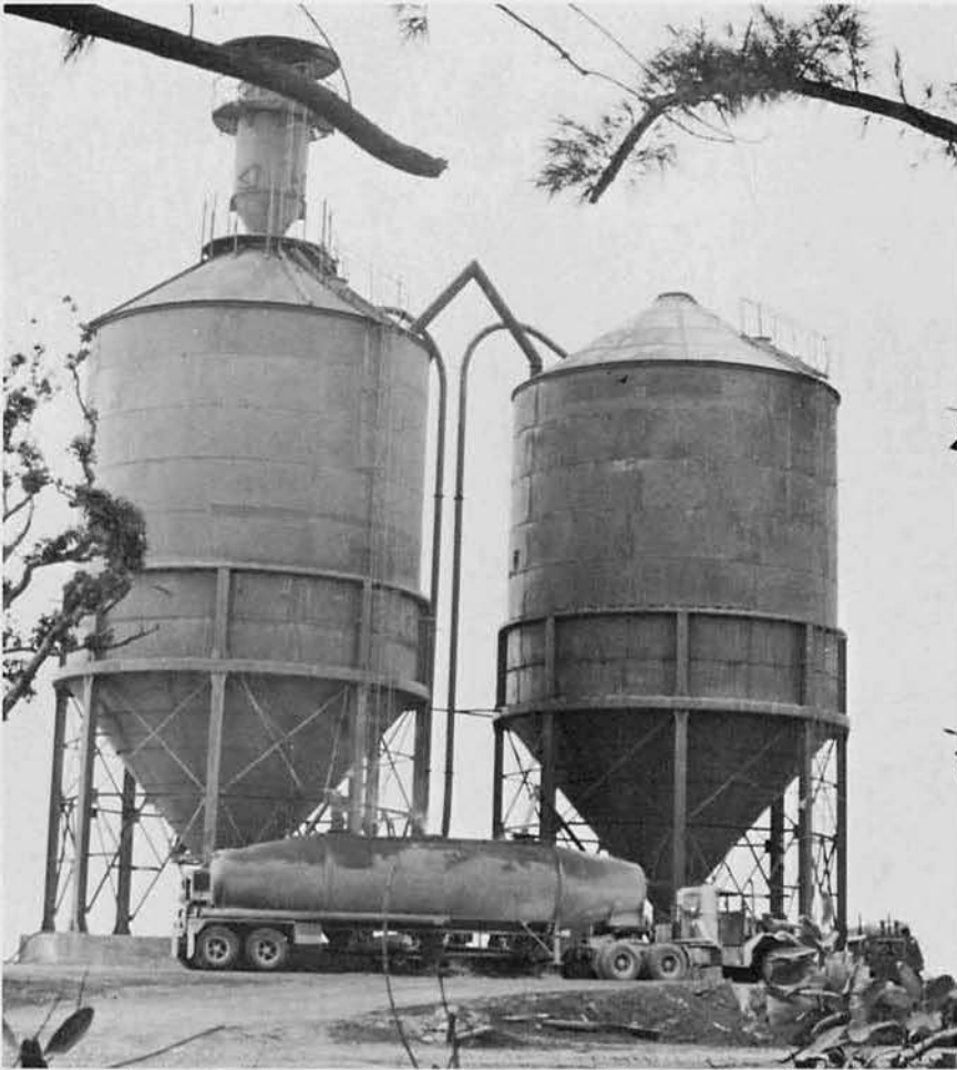
Cement silos — 58,000 cubic feet of storage space
