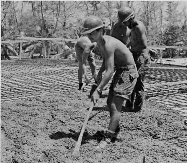
Placing concrete at BEQ #1
