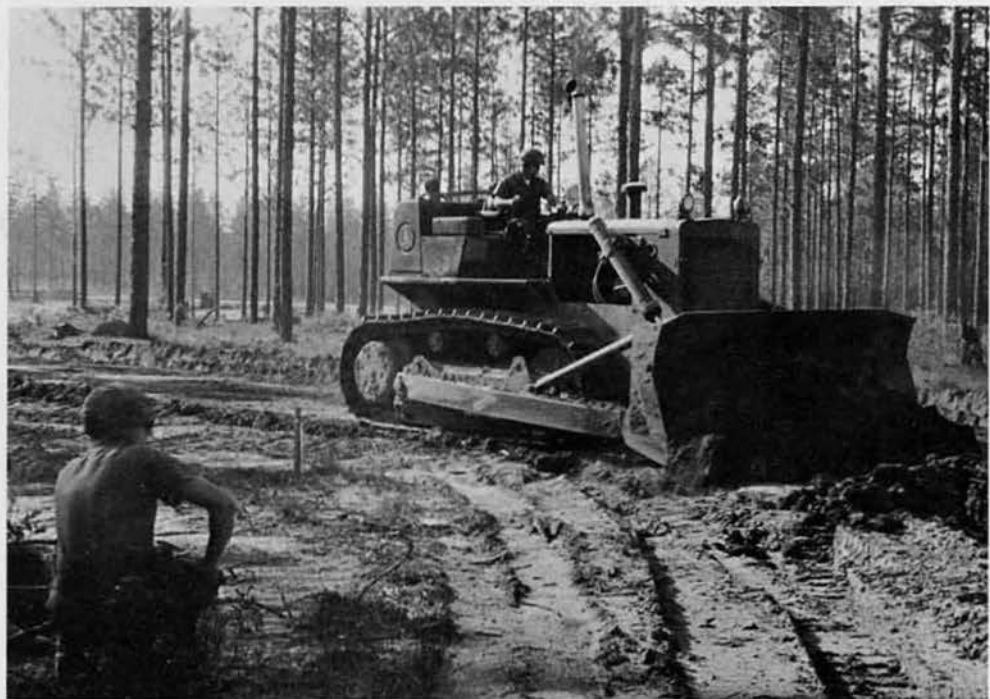
Road building in the field.
