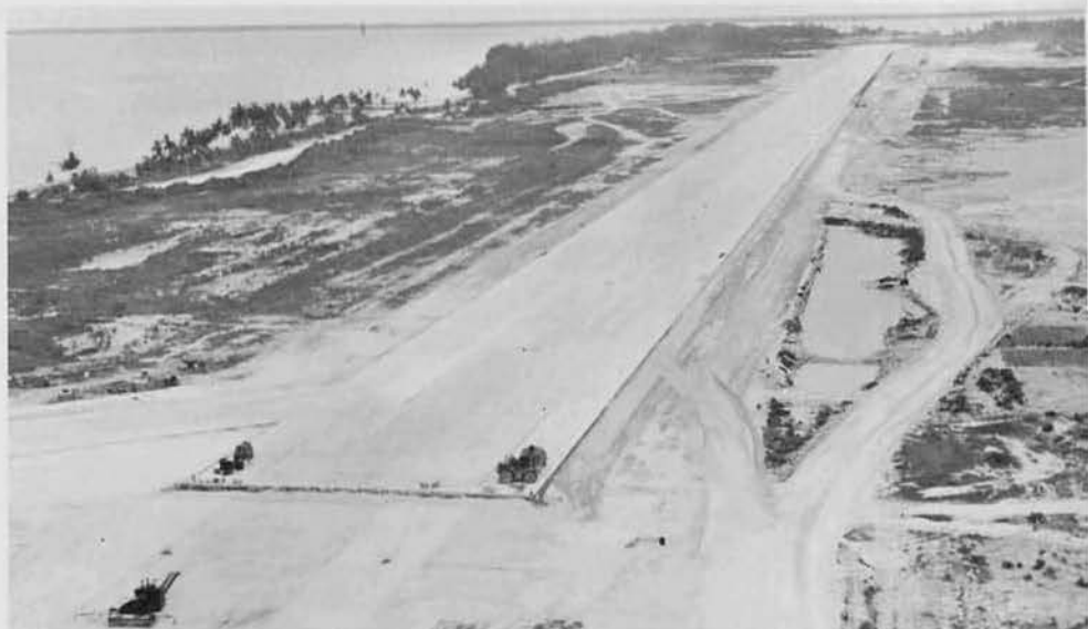
Aerial view of the runway built by NMCB-62
