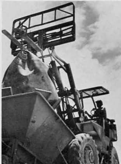
Loading the cement bin at the block plant.
