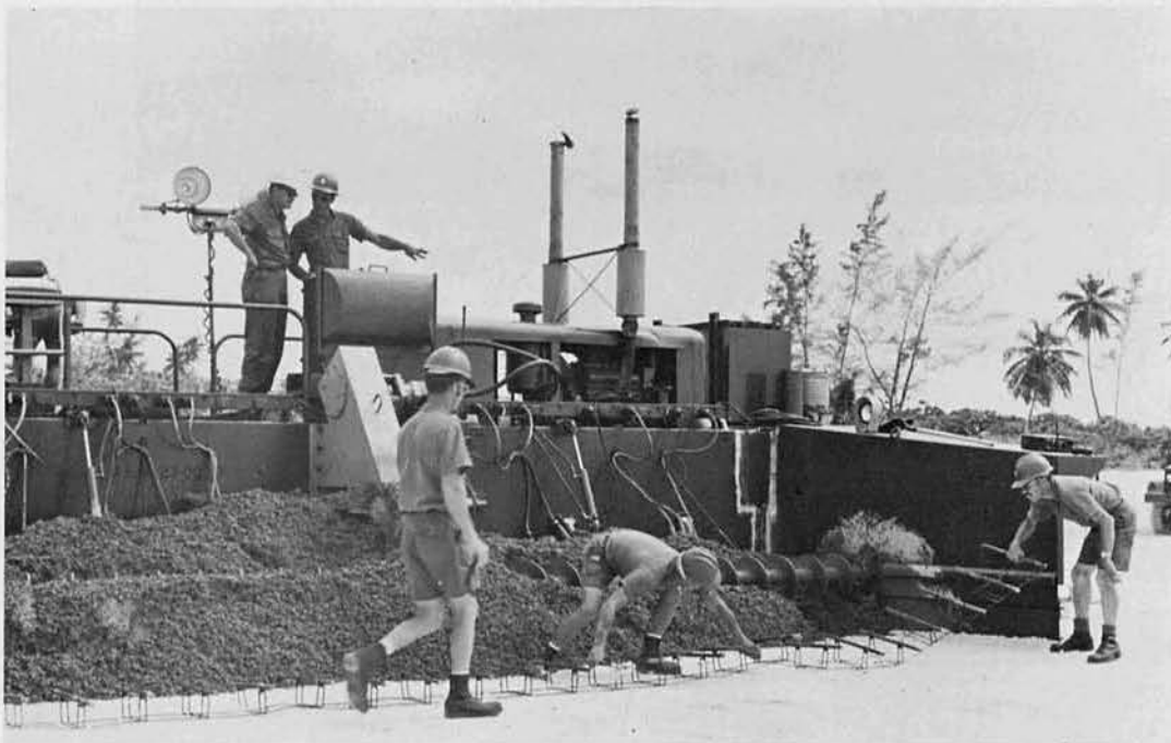
The slipform paver — maintained and operated by Alfa Co.
