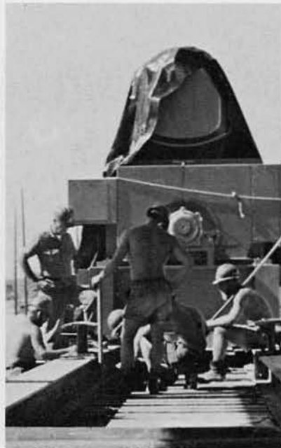
Setting the generators at Standby Power #1
