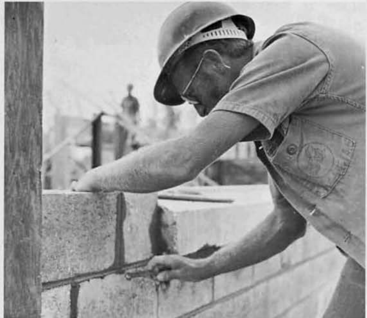
Jointing blocks at BEQ #2
