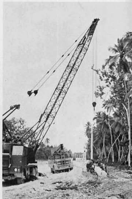
Setting power poles down south.
