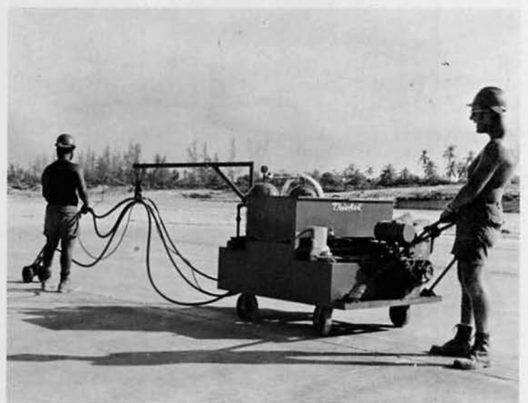
Sealing Joints on the Runway
