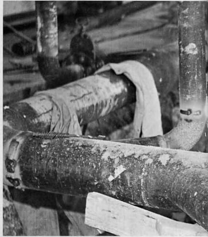
Welding Pipes at the Pub
