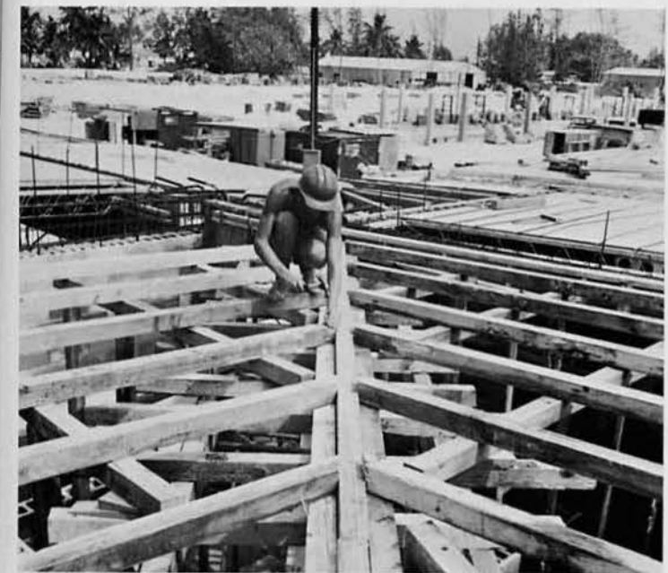
Building forms for a Concrete Roof Pour
