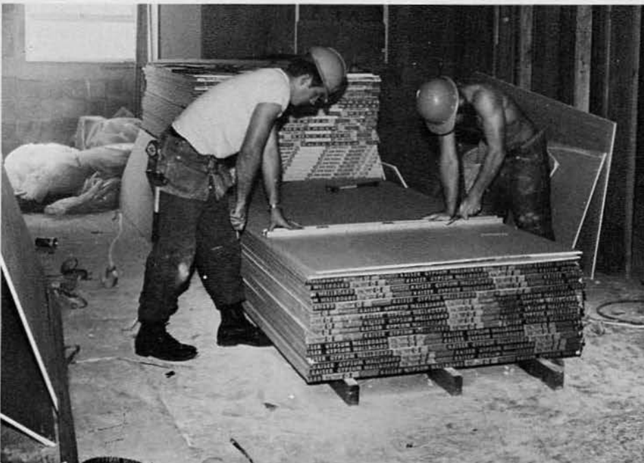
BU3 Stephenson and BUCN Michaud installing sheetrock on second deck.
