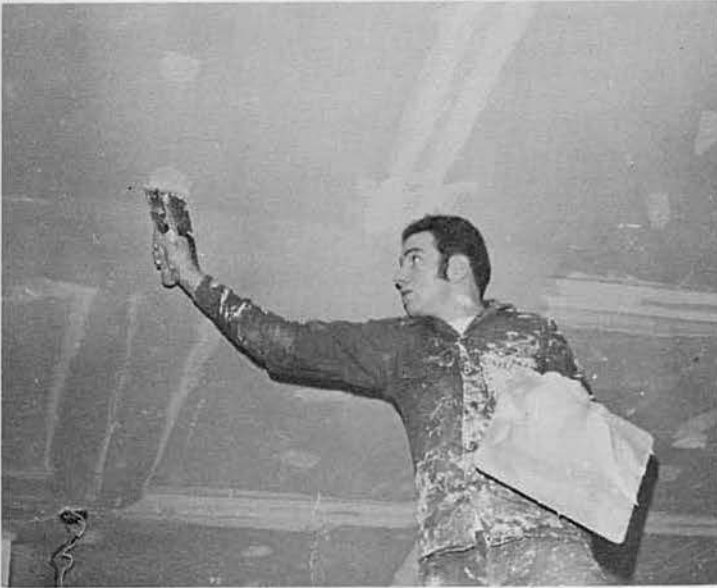
BUCN Coghlan finishing sheetrock.
