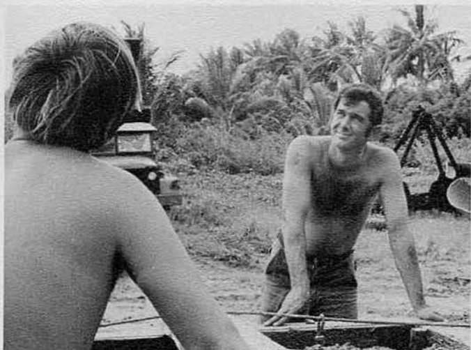
Chief Sadler waiting for concrete.
