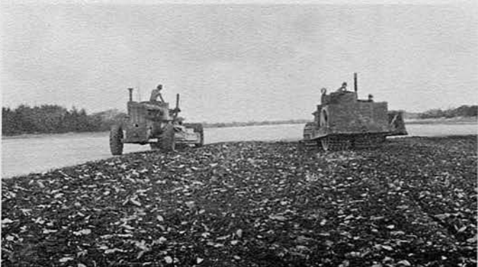
The job in progress
