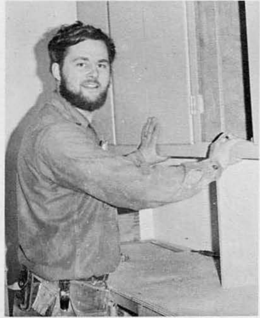
BU3 Larry McCollum installing cabinets.
