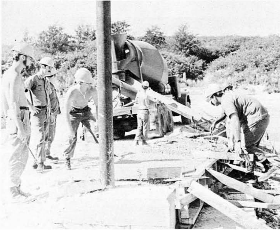
Pouring a wall for the Settling Pond at Orote Point.
