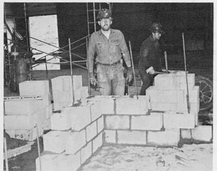
BU2 Wicks and EOCA Chapman laying classroom walls.
