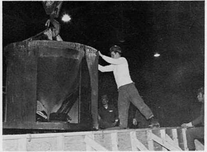
CN Freeman, BU1 Fitzpatrick, and BU3 Albright pouring classroom overhead slab.
