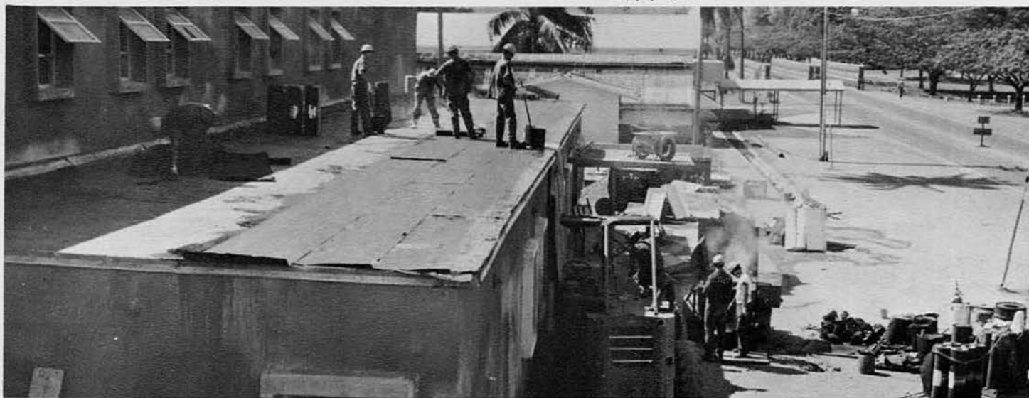
Application of built up roof.
