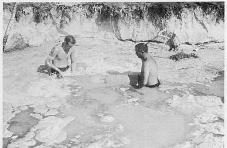
EOCN Doug Henle and UT3 "Rusty" Steele place brackish water well lateral. "Somebody has to do it!"
