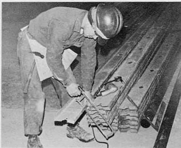
BUCN Moran cutting steel studs.
