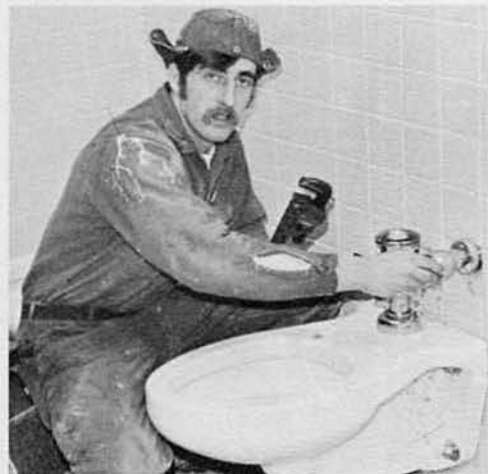
UT3 Ed Holleran installing plumbing fixtures
