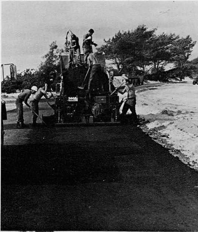
Laying cold mix I-62.
