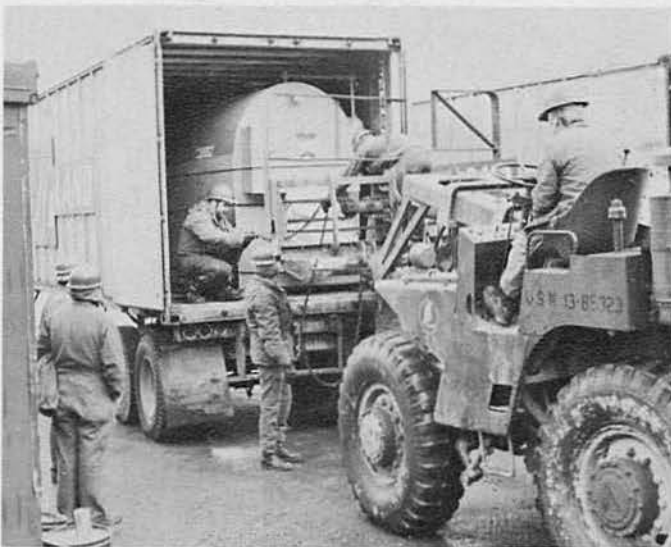
Unloading hot water boiler.
