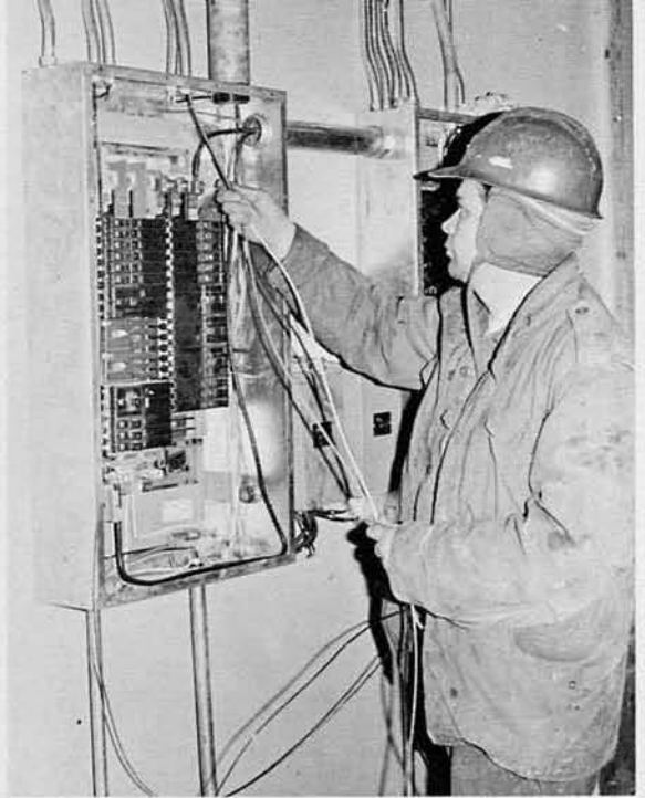
CE3 Dyer pulling wire into electric panel.
