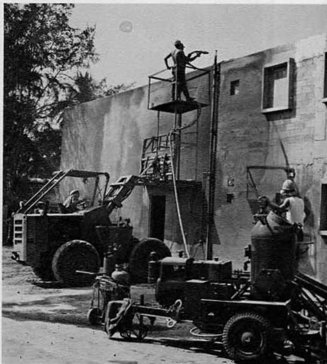
BU1 Viehmann operating the gunnite machine. BU2 Burnor operating the forklift while BU3 McPhearson and BUCN Sutton apply gunnite.
