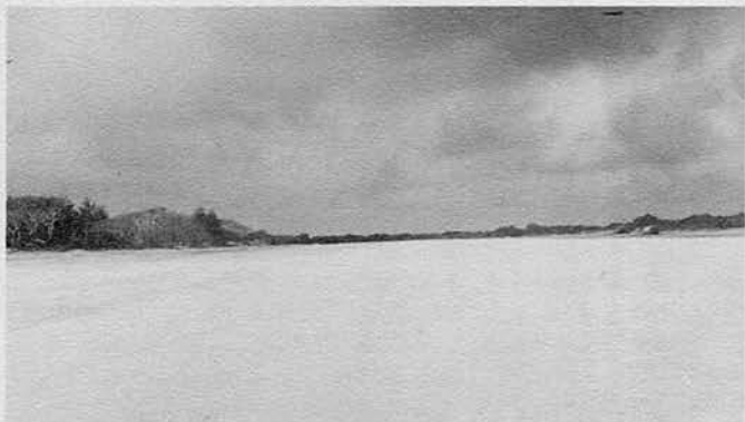
Compacted coral runway
