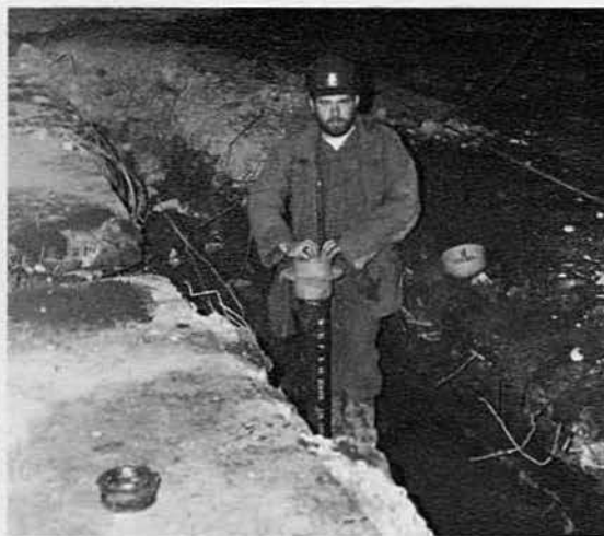
UT2 Bost installing underslab utilities.
