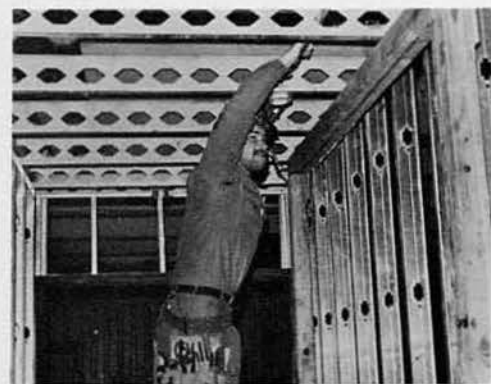
CE3 Drake installing conduit for overhead lighting.
