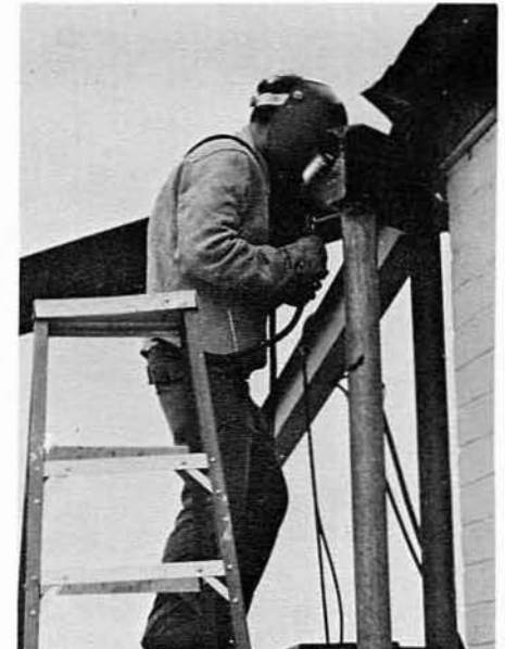
CA Edward J. Sullivan Doing overhead welding at Polaris Point Project.
