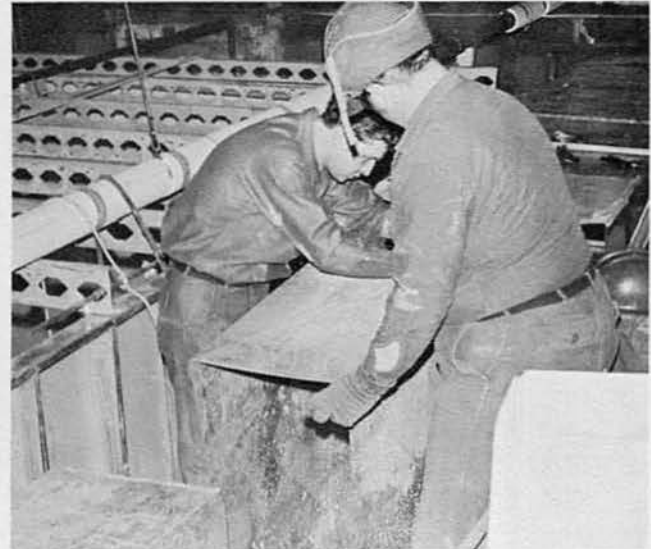
SW2 Terry Clotfelter and CA Mike Fosselman installing heating air ducts.
