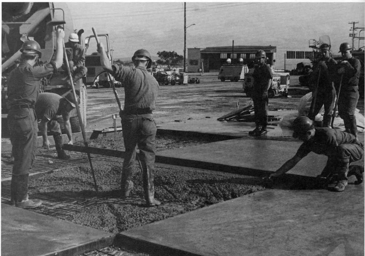
The Futenma Avionics Building.
