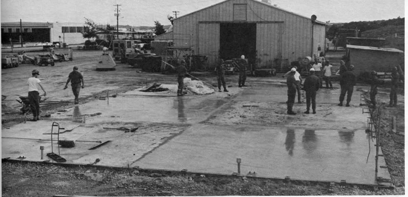
The pad is almost ready for the steel.
