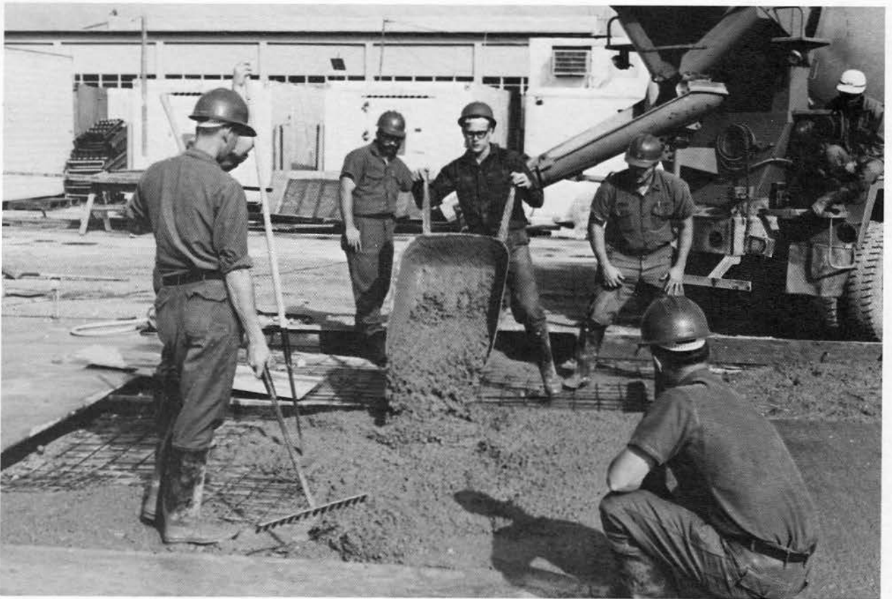
Concrete. Concrete, and more Concrete.
