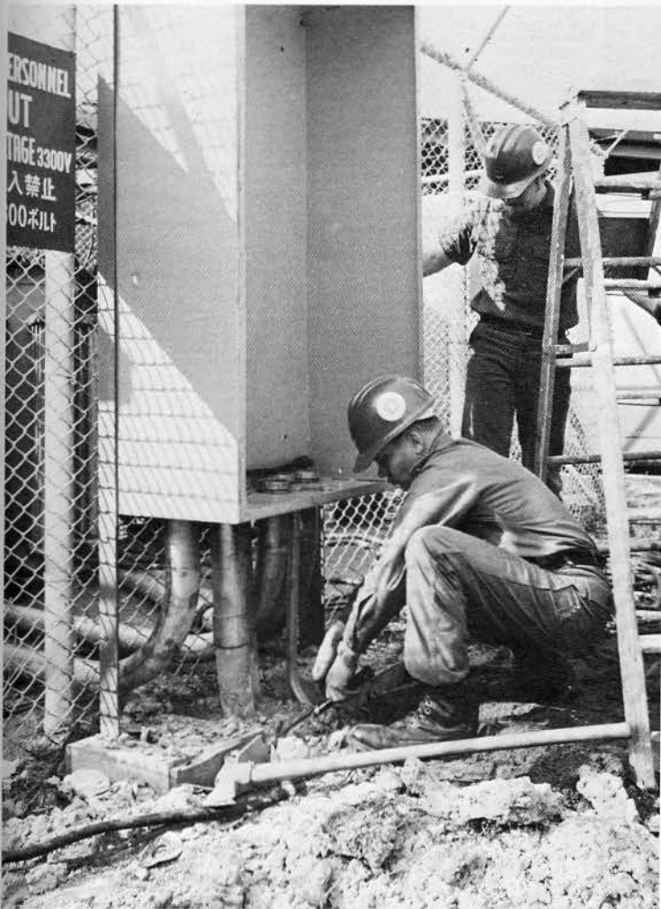
Conduit for the Generator Slabs.
