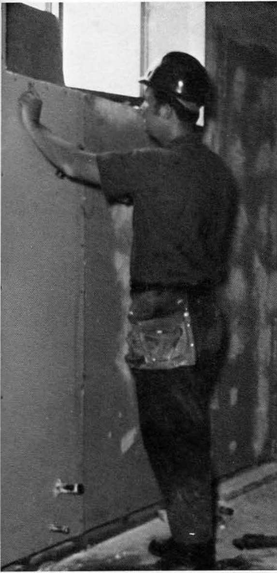
Nailing up sheetrock walls.
