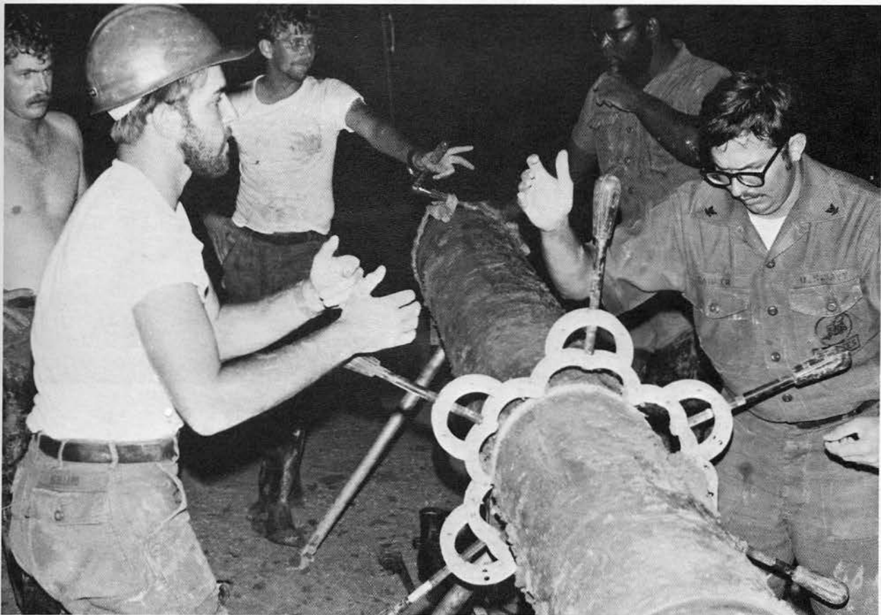
Midnight repairs in Camp Shields.
