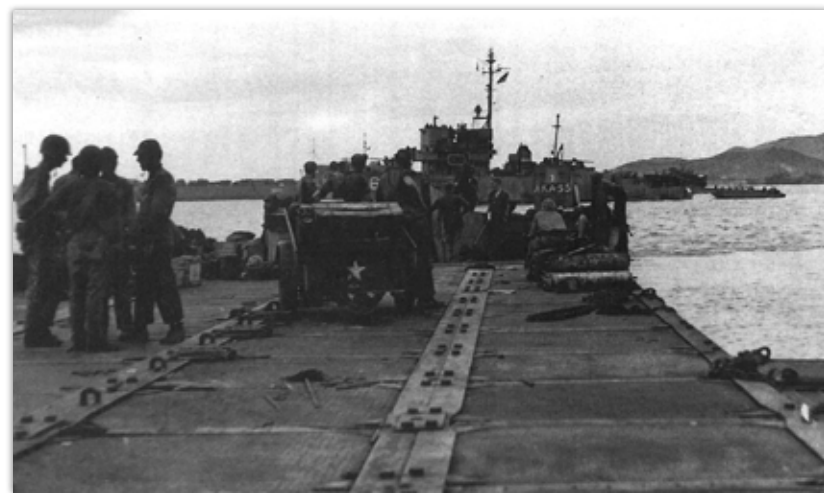
Two days after the initial assault at Inchon, Seabees unload attack cargo ship Alshain (AKA 55) landing craft onto the pontoon dock built by the naval constructionmen at Wolmi Do. (USN 420358)
