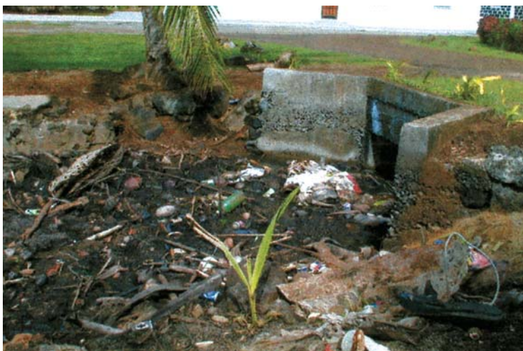
Figure 5 Wastewater outfall at Lalaleu.
