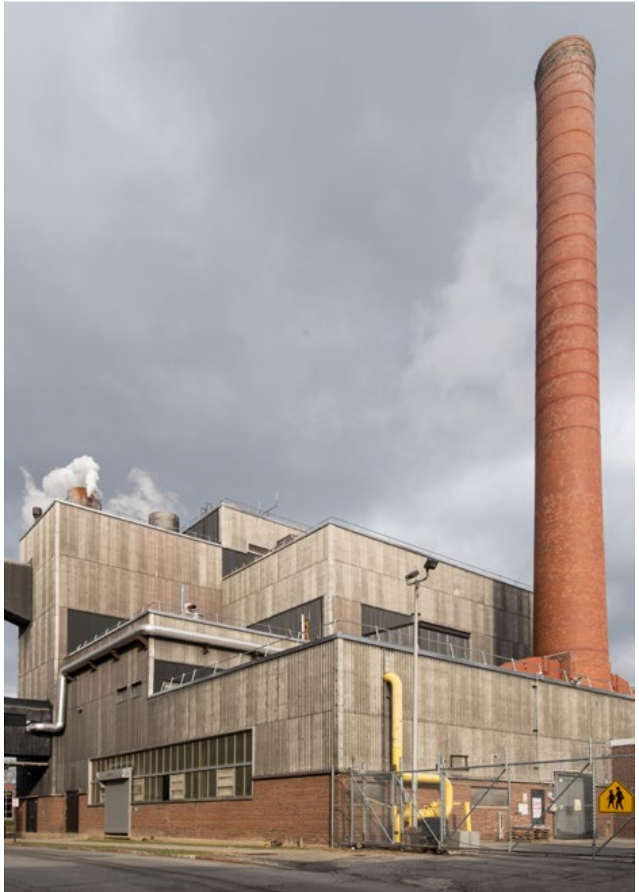
EXISTING ENERGY PLANT
