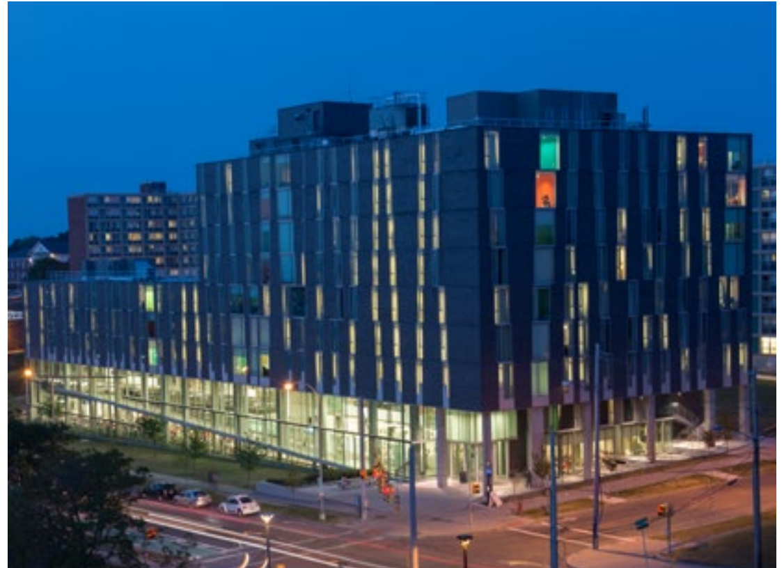
ERNIE DAVIS HALL CONSTRUCTION 2008-2009
