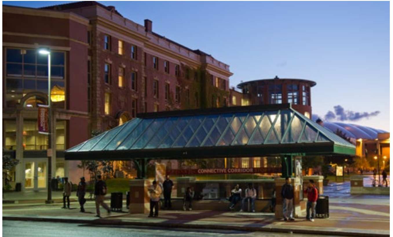
BUS SHELTERS HELP SHIELD TRANSIT RIDERS FROM INCLEMENT WEATHER, IMPROVING RIDER EXPERIENCE.
