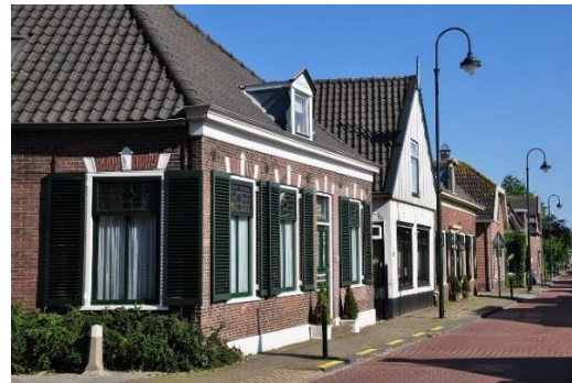
brick masonry mass wall structure
