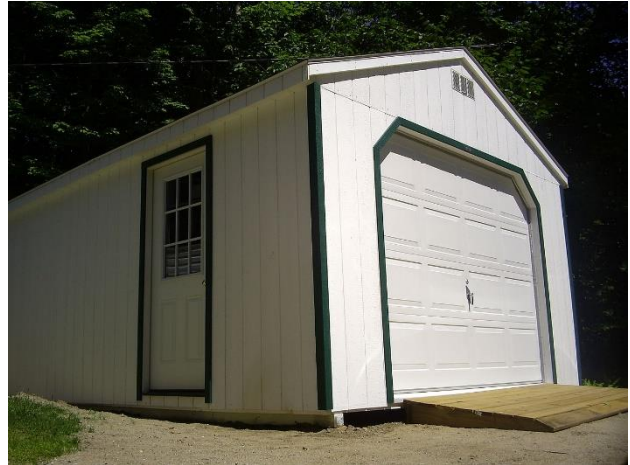
metal frame structure with wooden panels
