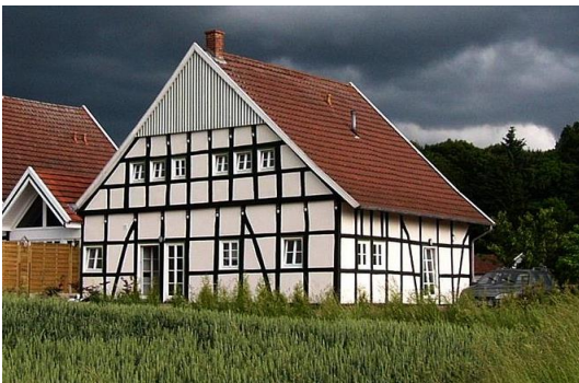
strong wooden frame structure
