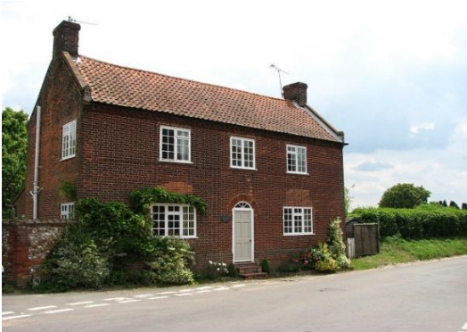
brick masonry mass wall structure
