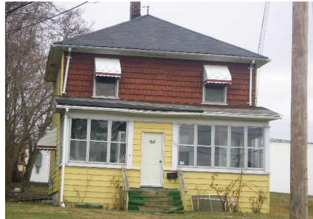
weak wooden frame structure
