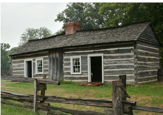
wood log (load carrying) building structure
