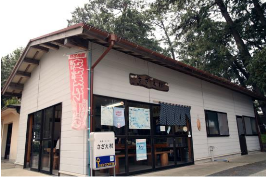
strong wooden frame structure
