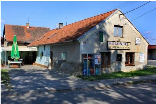
concrete block mass wall structure
