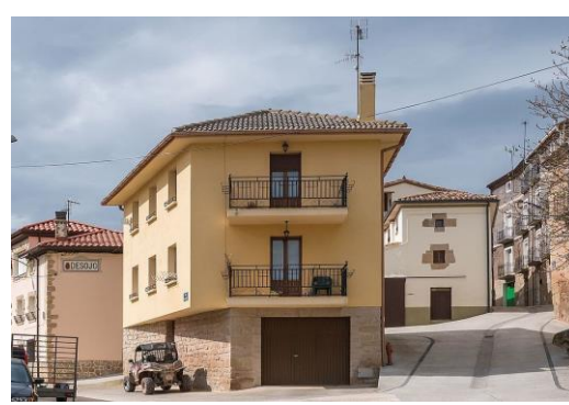
brick masonry mass wall structure
