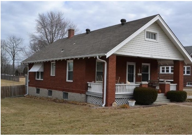
weak wooden frame structure with brick veneer
