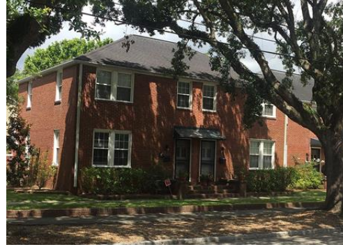
strong wooden frame structure brick veneer
