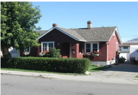
strong wooden frame structure with brick veneer
