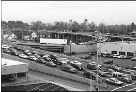
Center Street bridge on a typical morning.
