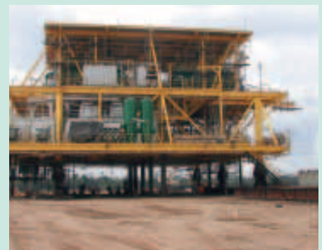
Estuary flowstation during construction in Warri
