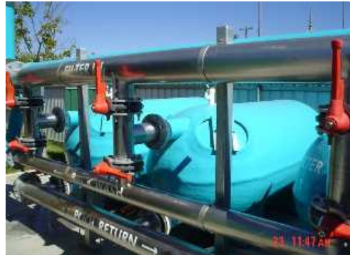
Castlemaine Swimming Pool Filtration Upgrade
