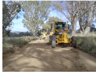
Routine Maintenance Grading
