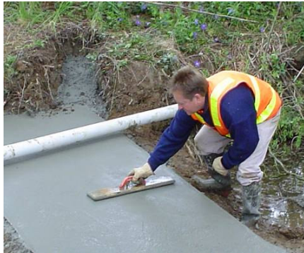
CHEWTON TOWN ENTRANCE Beautification Works Footbridge
