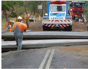
Placing Precast deck on Golden Point Road bridge
