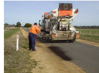
Sealed road patching
