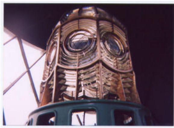
Souter Lighthouse biform lens
