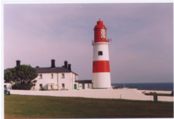
Souter Lighthouse and former keeper's dwelling
